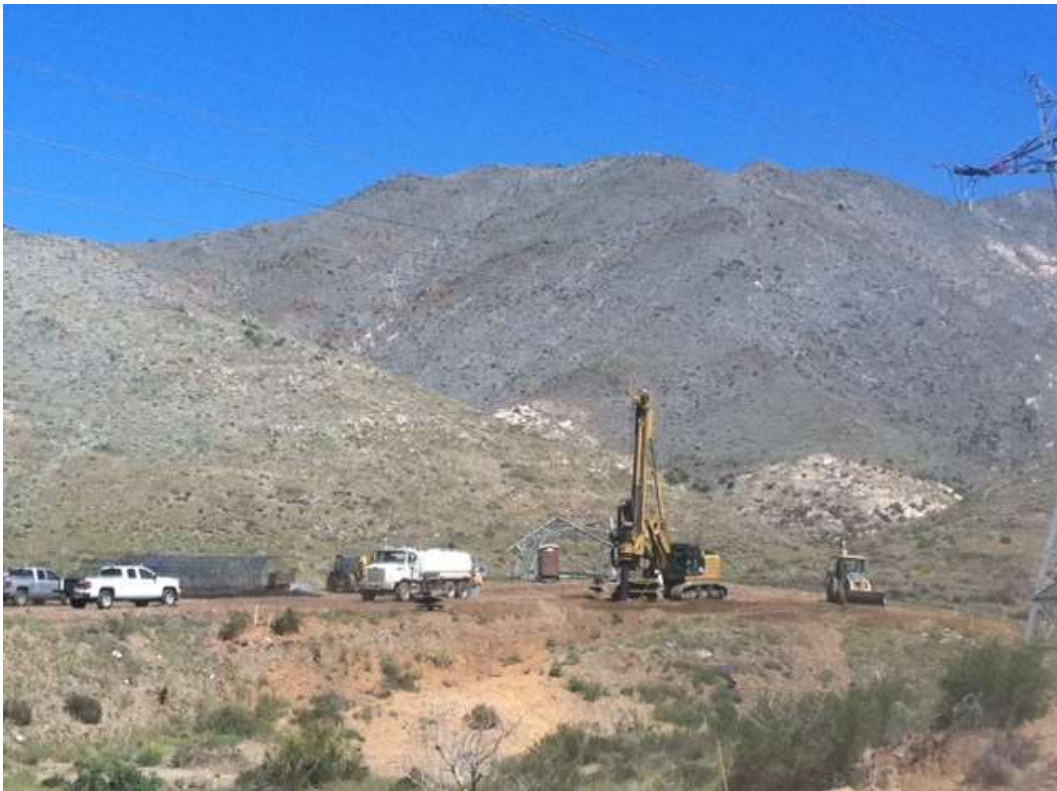
Figure 2: Foundation excavation occurring at Construct 11XX, Segment 11C.
