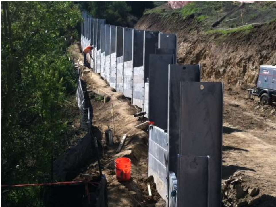
Figure 5: Wall panel installation at Tower M49-T1, Segment 8, Phase 4.
