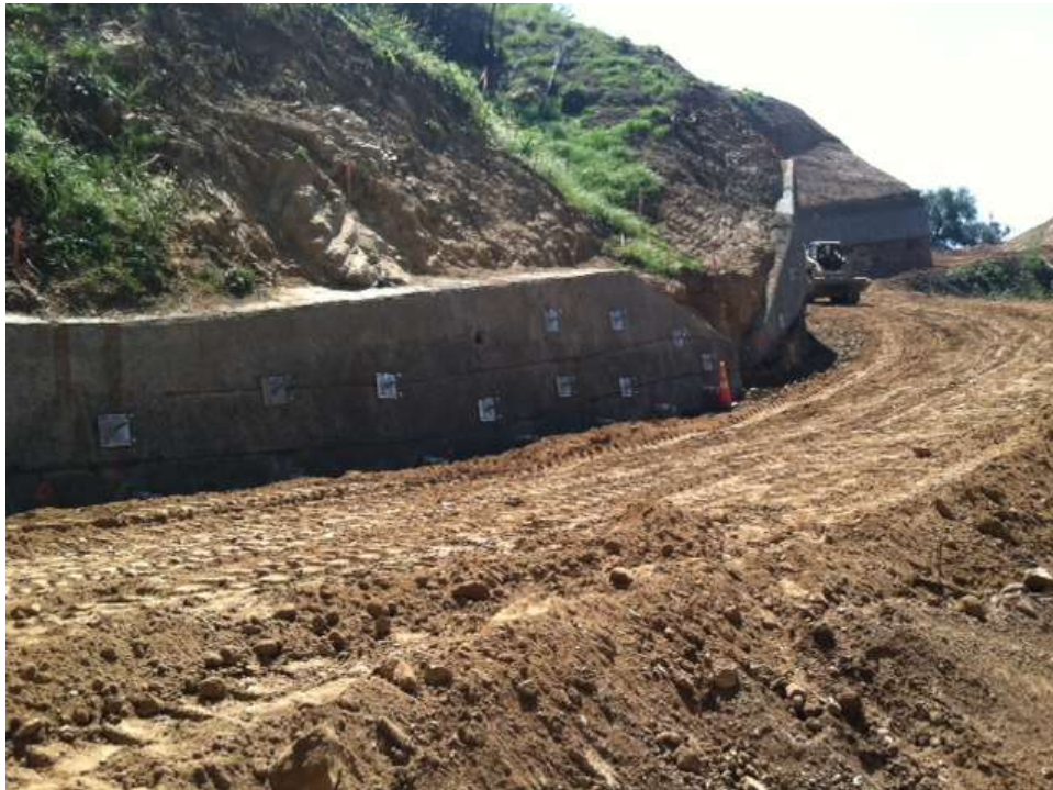
Figure 4: Soil nail wall construction at Tower M27-T3, Segment 7.
