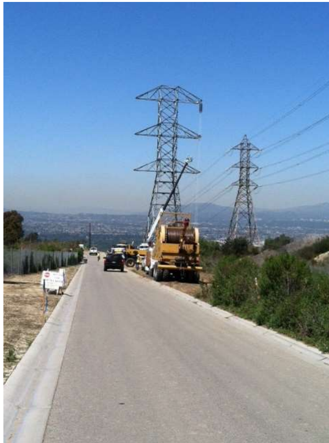
Figure 6: Wire stringing continued near Rose Hills, Segment 8, Phase 4.
