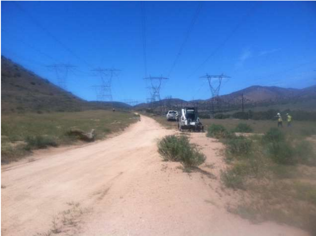
Figure 1: BMP removal crews working on Segment 5.
