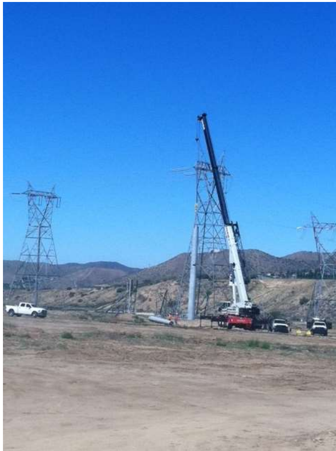
Figure 3: Tower erection occurring at Construct 0, Segment 11C.
