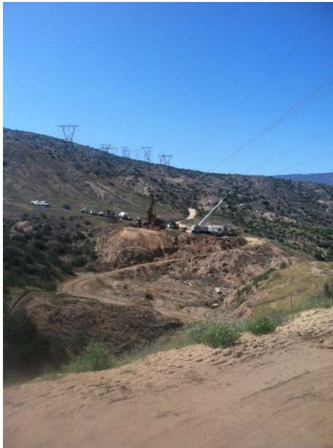
Figure 3: Foundation activities at Construct 11AX, Segment 11C.
