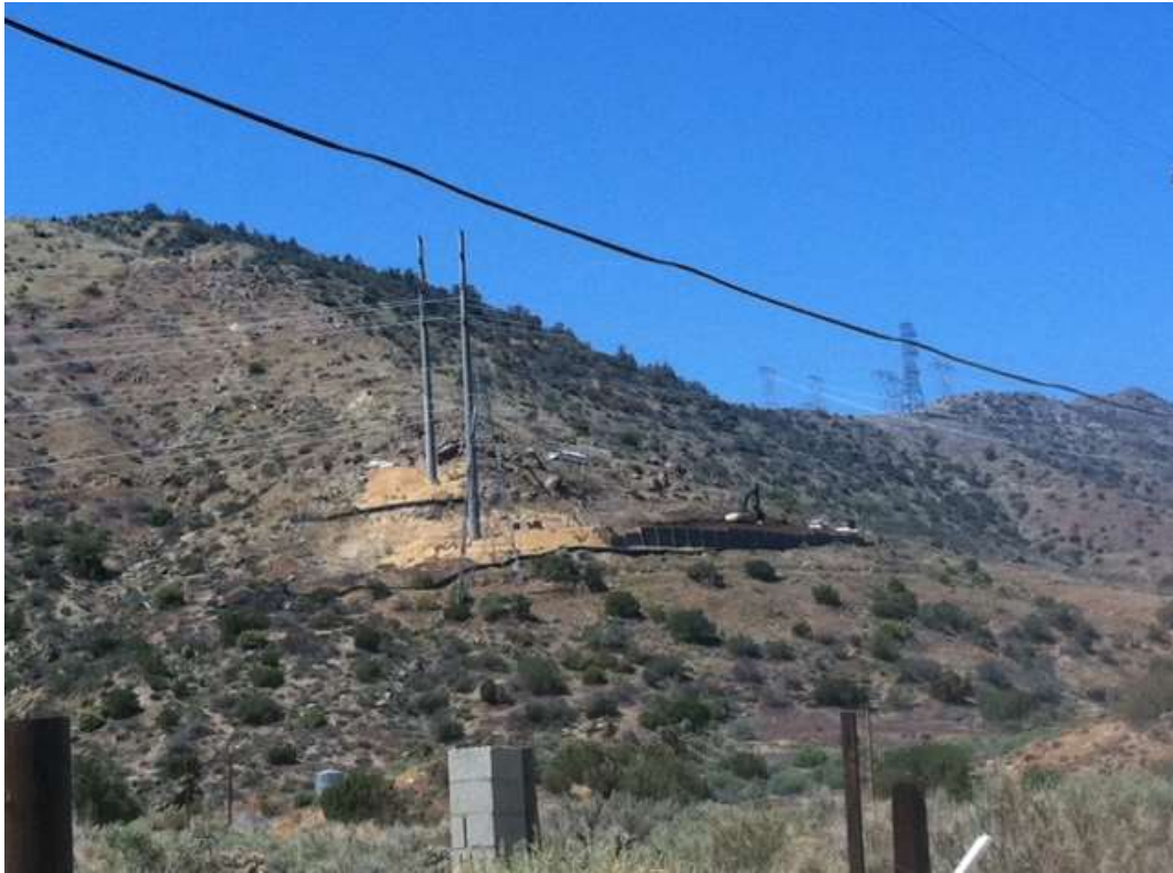
Figure 1: Final stabilization activities, Construct 8, Segment 6.
