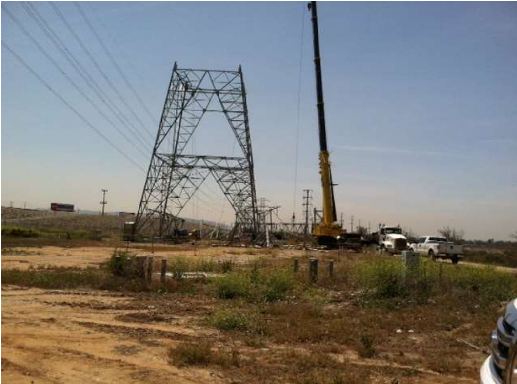
Figure 8: Tower assembly, Segment 7.
