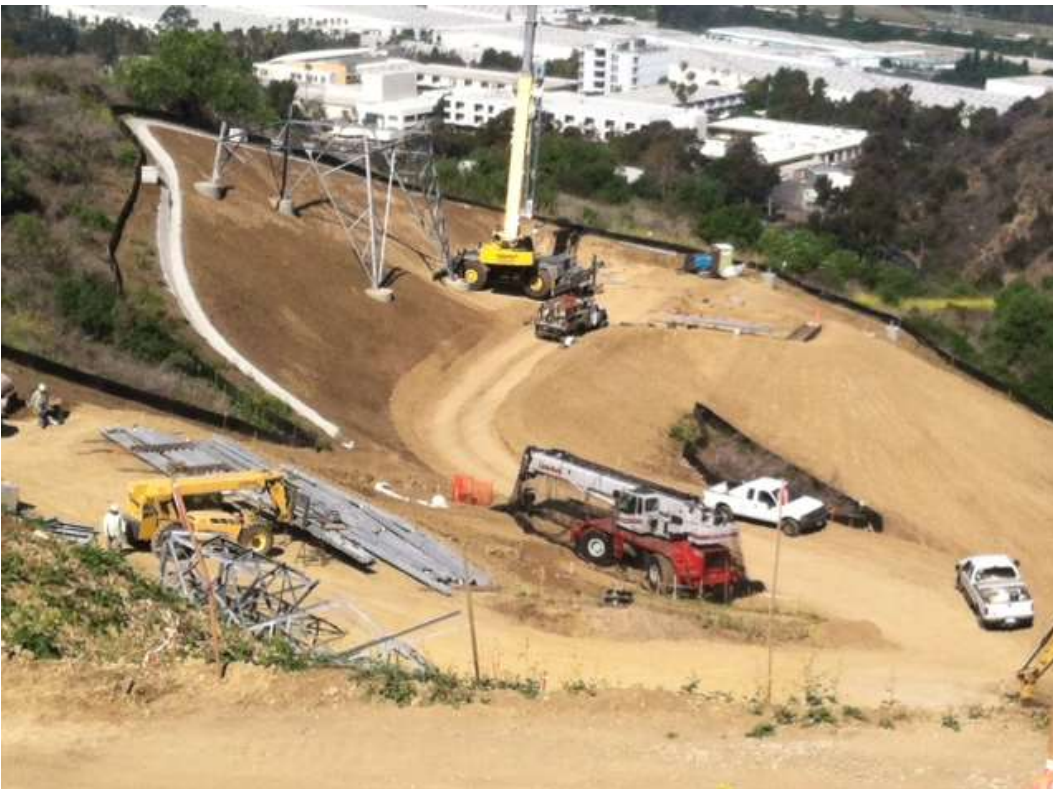
Figure 10: Assembly of Tower 43/3, Segment 8, Phase 4.
