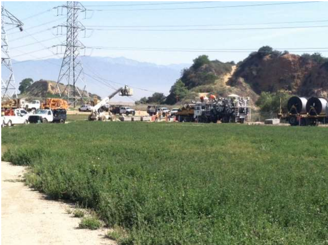
Figure 11: Wire stringing activities near Rose Hills, Segment 8, Phase 4.
