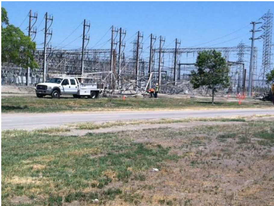
Figure 6: SCE crews removing 66 kV tower near the Chino Substation.
