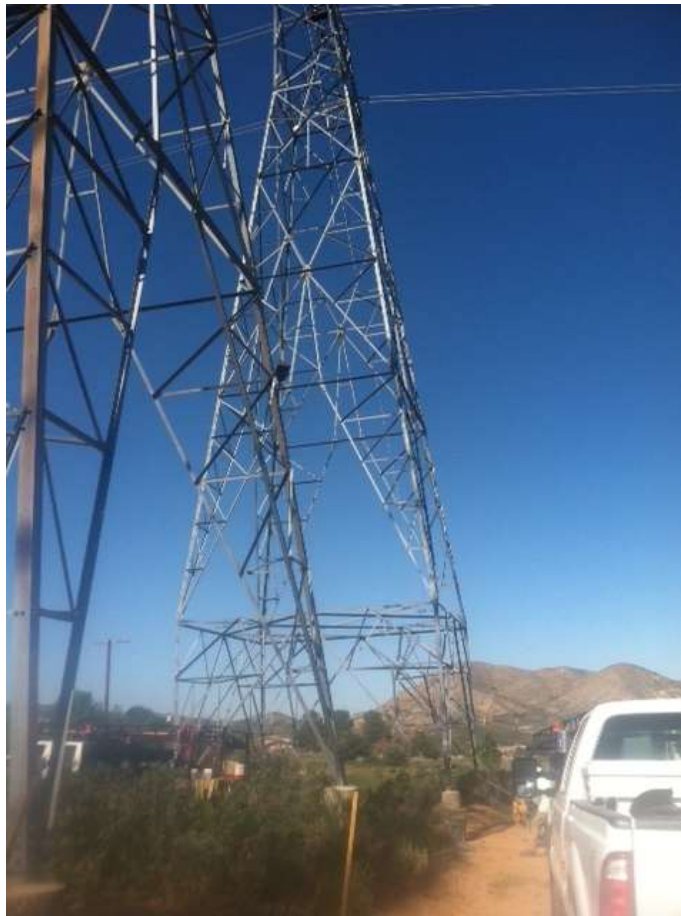
Figure 5: Traveler installation for wire removal activities at Construct 15, Segment 11C.
