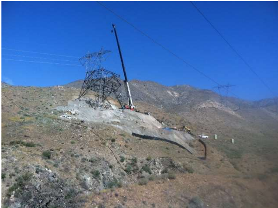
Figure 4: Construct 10 erection activities on Segment 11C.
