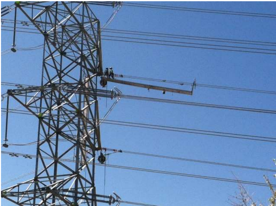
Figure 8: Wire stringing activities near Rose Hills, Segment 8, Phase 4.
