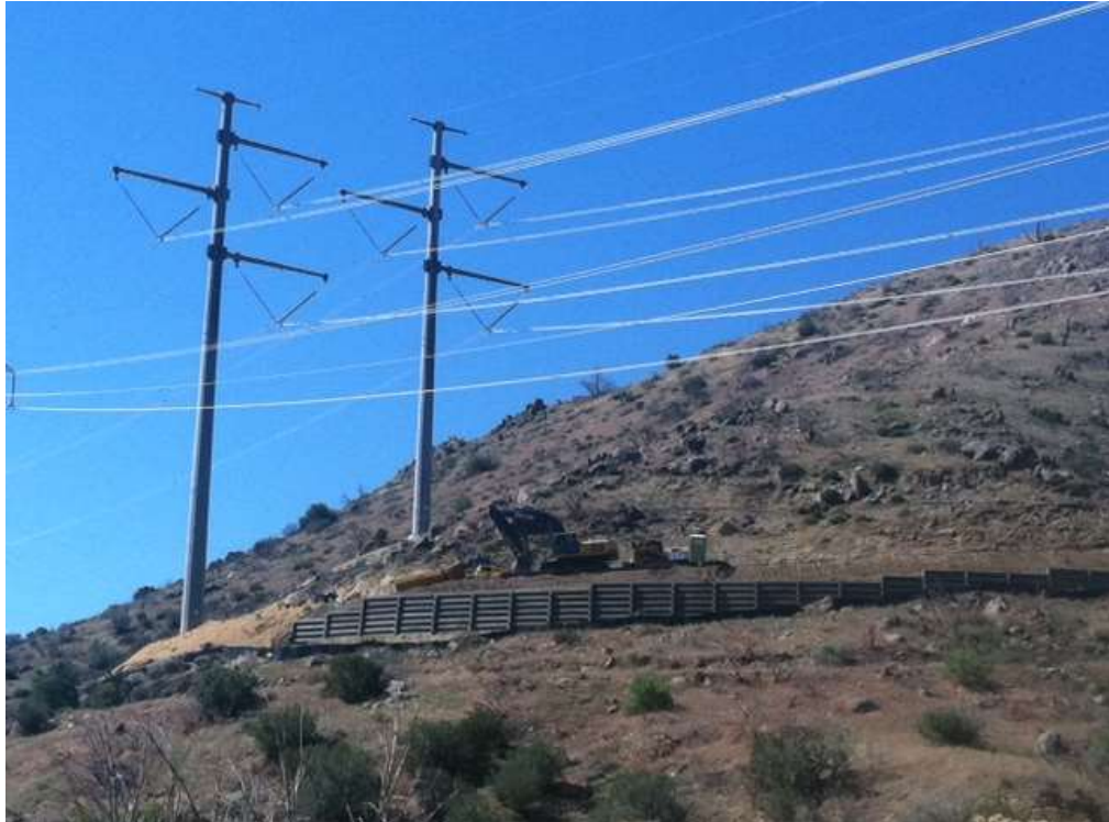
Figure 2: Final stabilization activities, Construct 8, Segment 6.
