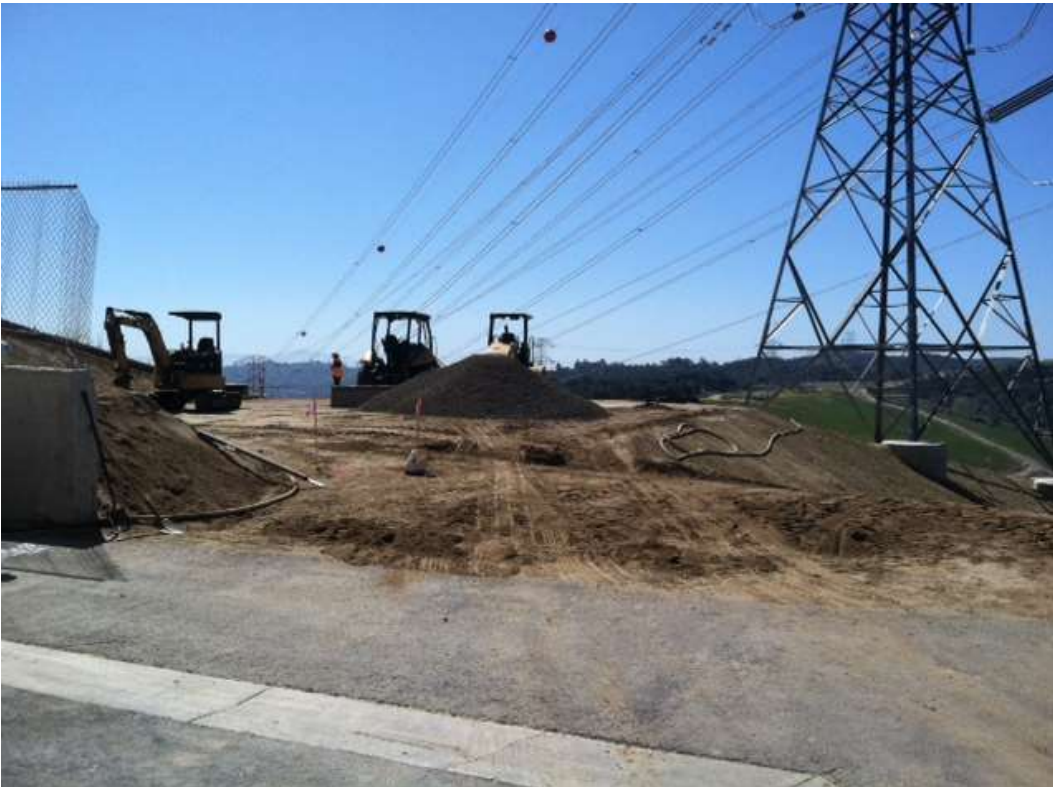
Figure 6: Spur road construction (fill and grading) at Tower M44-T3, Segment 8, Phase 4.
