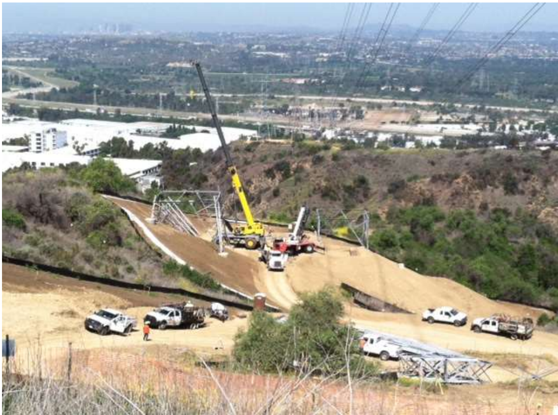
Figure 7: Tower assembly at Tower M43-T3, Segment 8, Phase 4.
