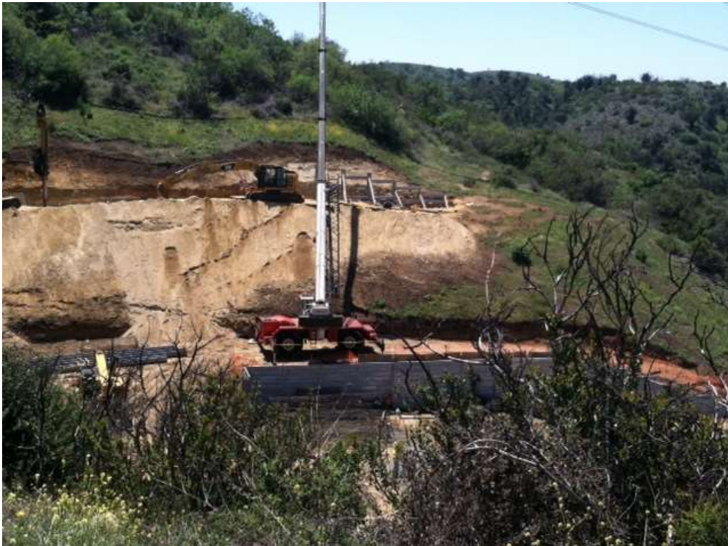
Figure 5: Soldier pile wall construction at Tower 57-T1, Segment 8, Phase 1.
