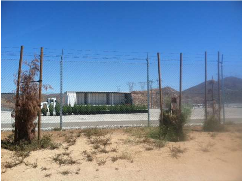
Figure 1: Dead trees were replaced along the outside of the Vincent Substation.
