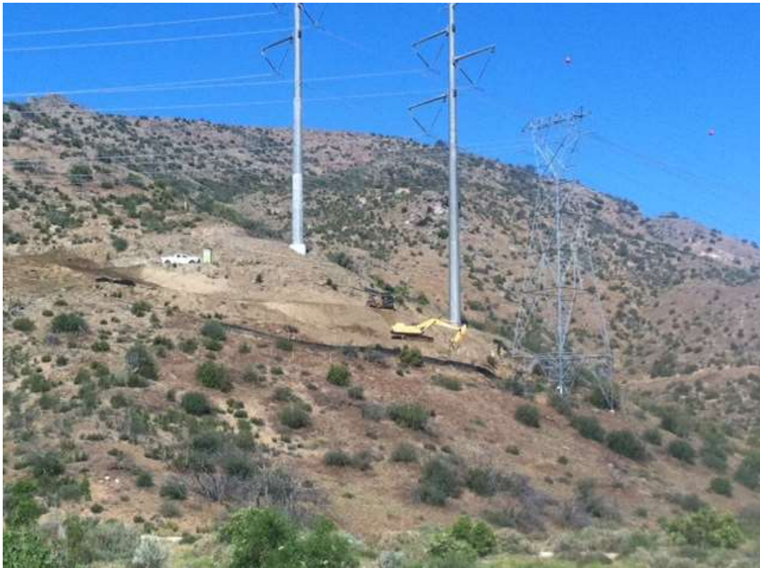
Figure 3: Final stabilization activities, Construct 10, Segment 6.
