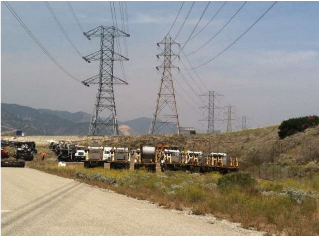
Figure 7: Wire pulling equipment set up prior to pulling operations, Segment 7.
