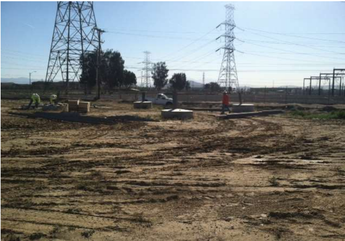
Figure 8: Assembly at Tower M73-T4, Segment 8, Phase 3.
