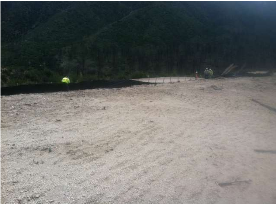
Figure 4: Exclusionary silt fence being up-righted at Pull/Tensioner Site 62/63, Segment 6.
