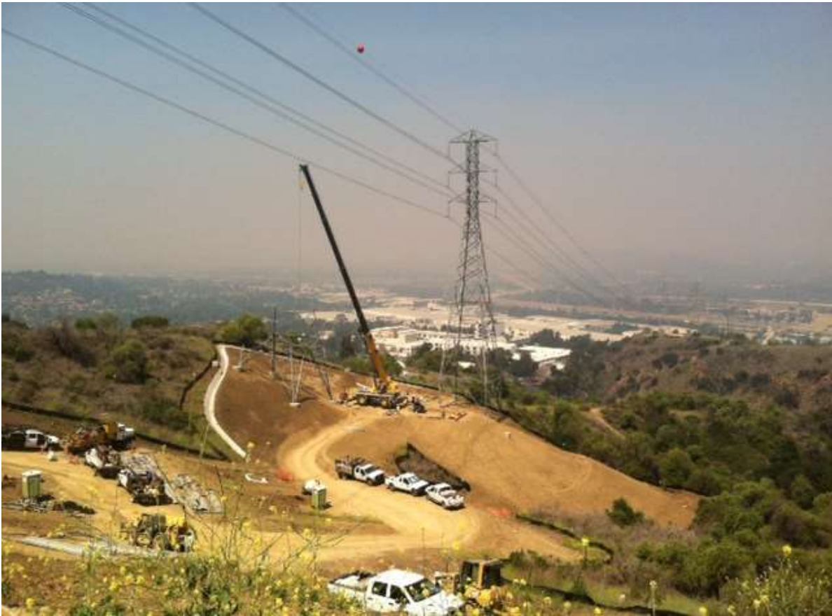
Figure 9: Assembly at Tower M43-T3, Segment 8, Phase 4.
