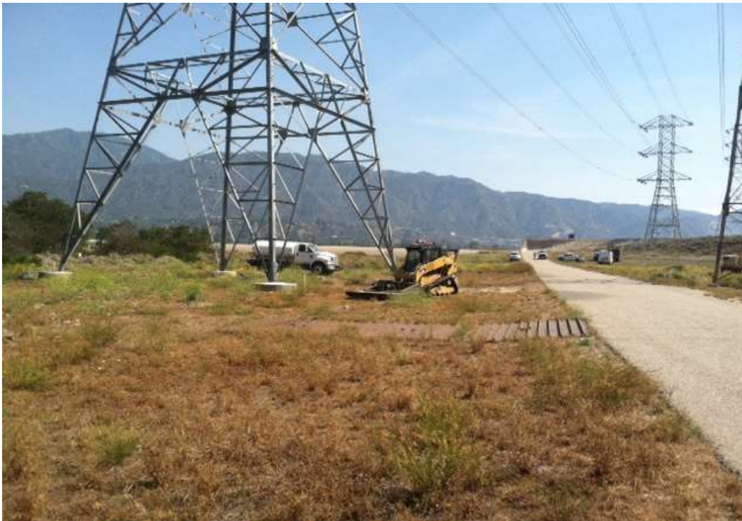
Figure 6: Vegetation clearing in tower disturbance areas and wire stringing sites, Segment 7.
