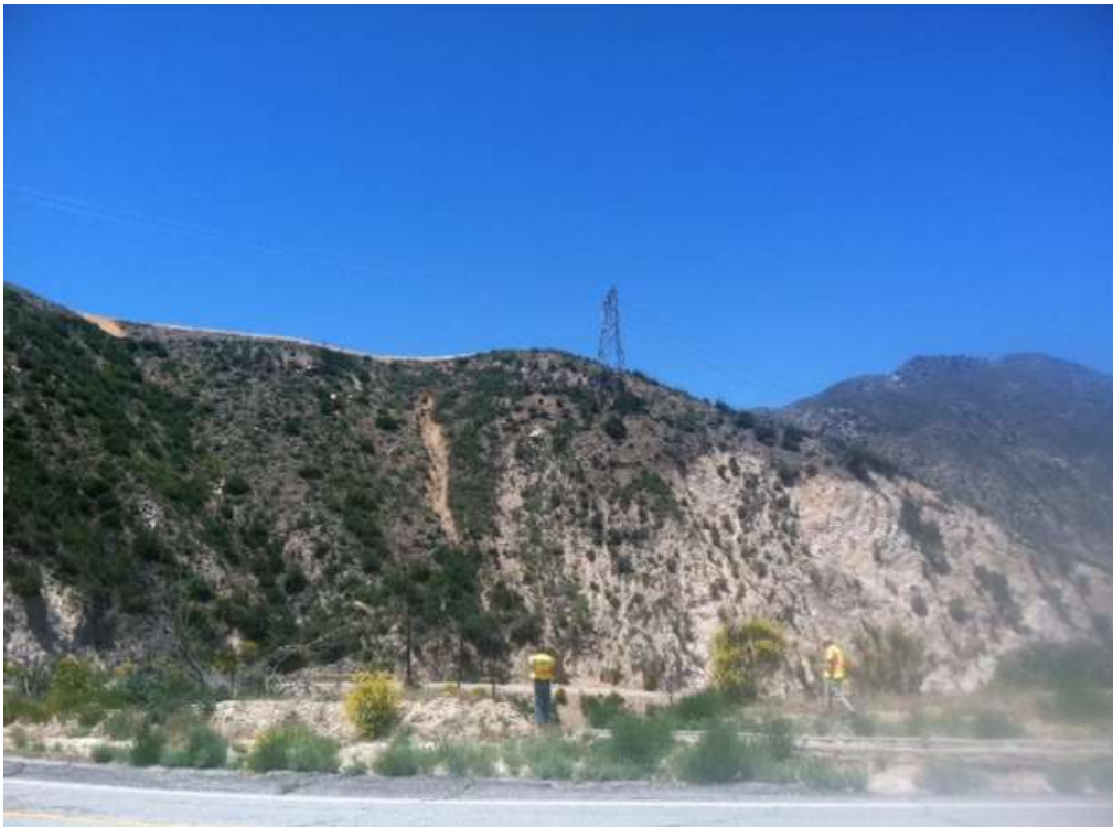
Figure 2: Water Board review of Pull/Tensioner Site 53/54, Segment 11C.
