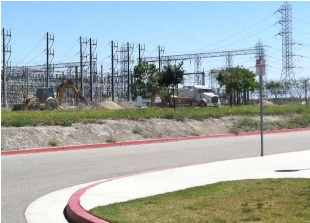
Figure 5: Wreck-out and site compaction at Tower M0-T3, Segments 7 and 8 66 kV.
