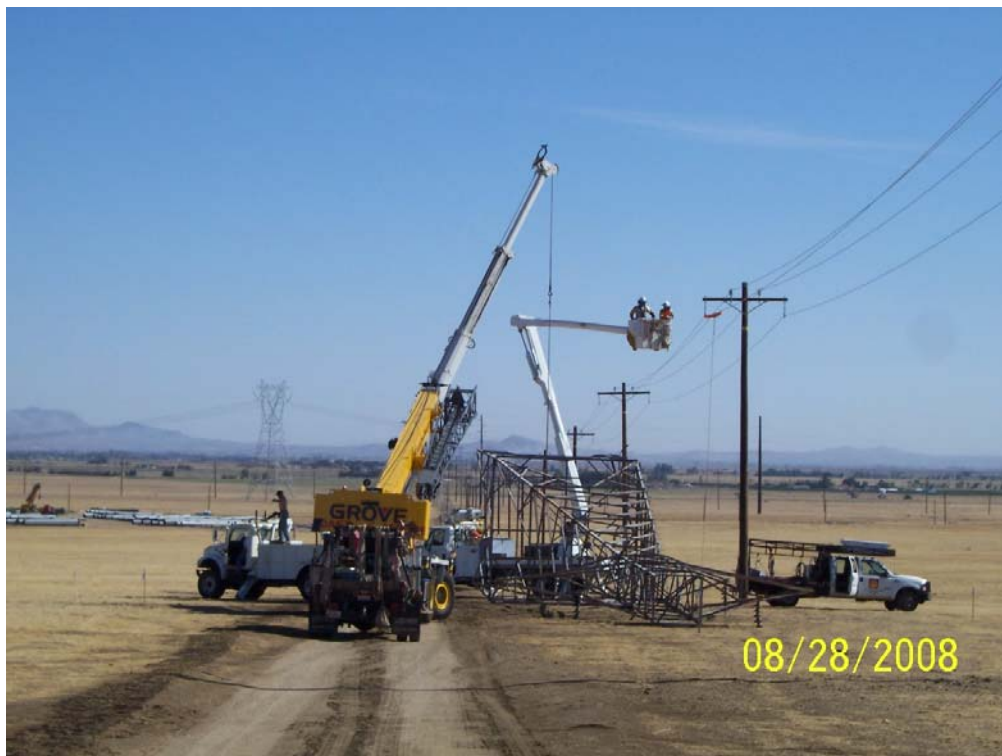
Figure 2: Dismantling of 66 kV towers in Section 3.
