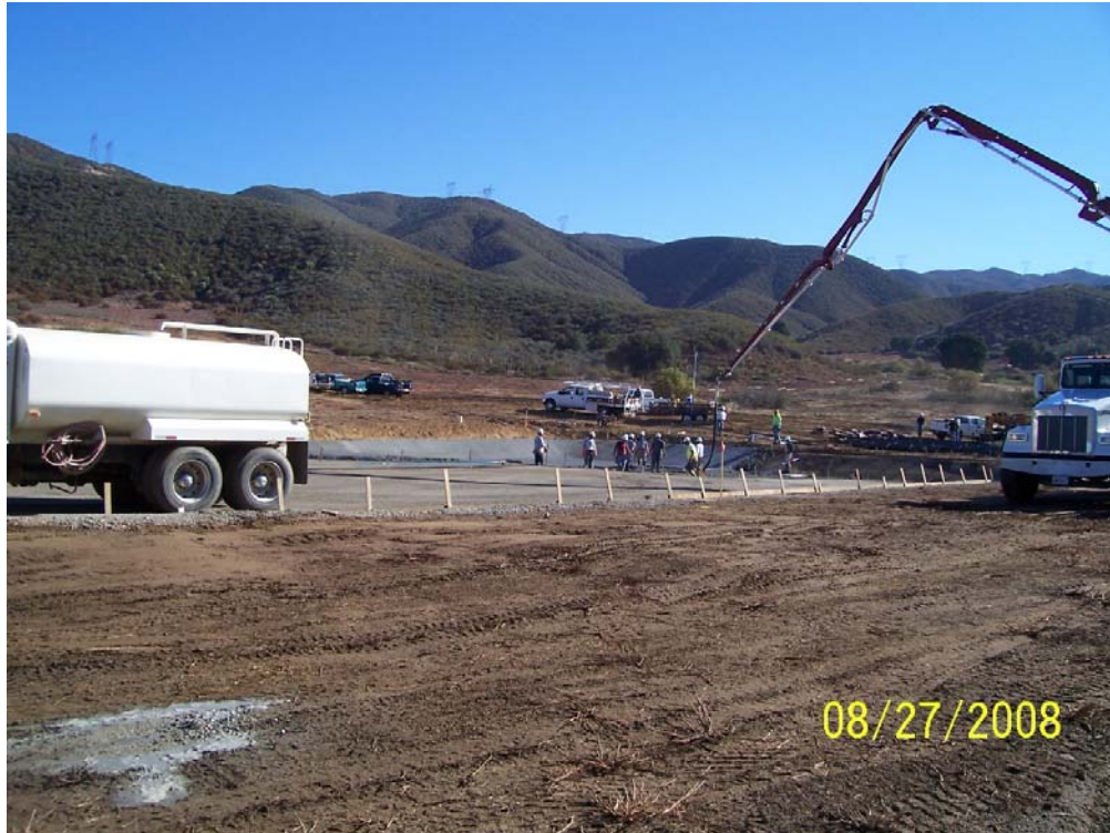
Figure 1: Construction of helicopter and fueling containment pad Hydrant Yard.
