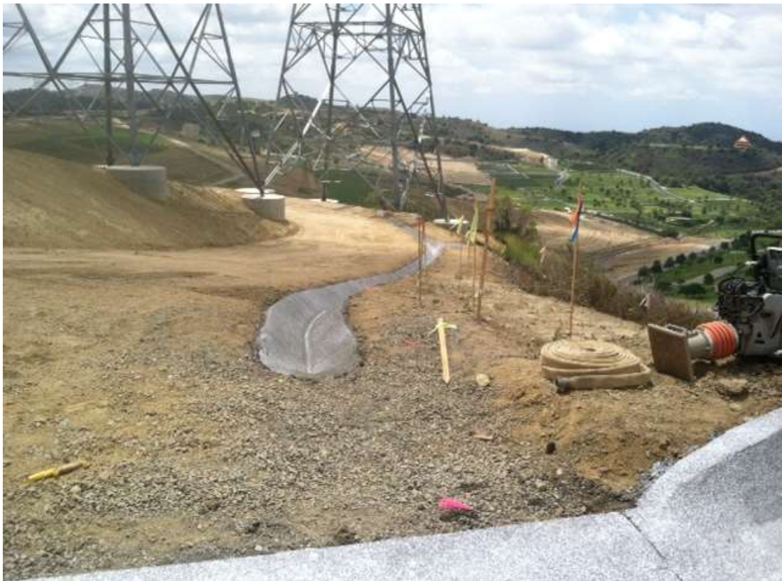
Figure 6: V-ditch installation at Tower M44-T3, Segment 8, Phase 4.
