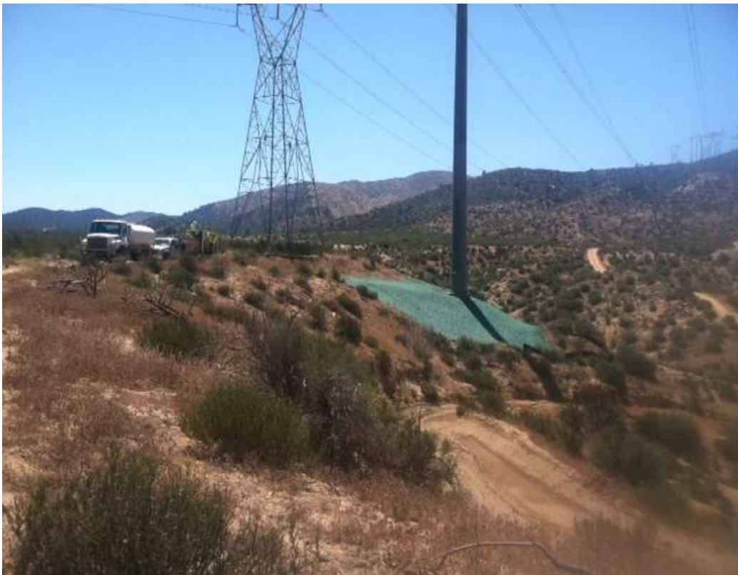
Figure 2: Hydromulching activities (BMP installation) occurring at Construct 16, Segment 6A.
