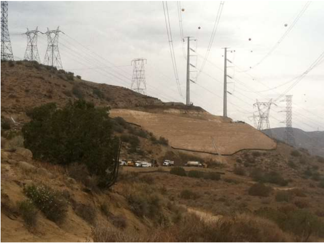
Figure 1: Grading activities at Construct 5, Segment 6A.
