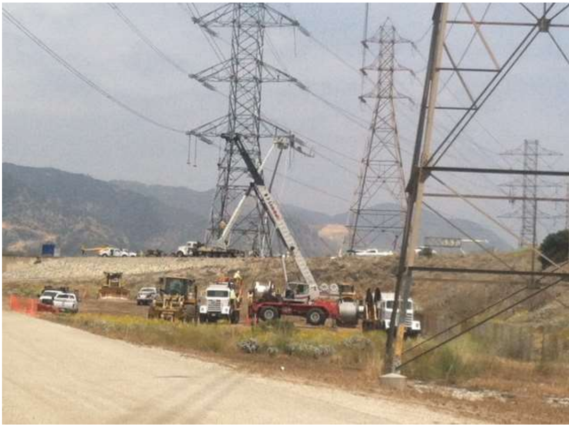
Figure 3: Wire stringing operations crossing the 605 Freeway, Segment 7.
