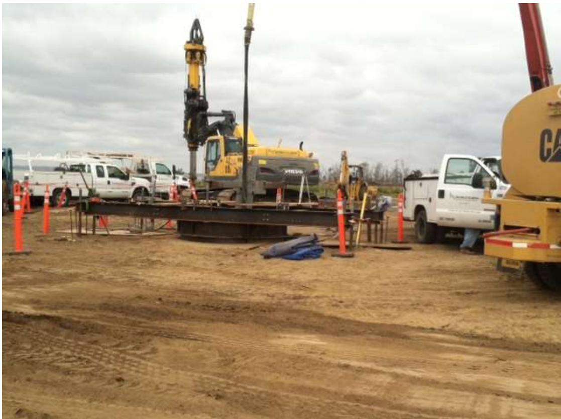
Figure 4: Concrete pouring of Tower M70-T5 foundation, Segment 8, Phase 4.
