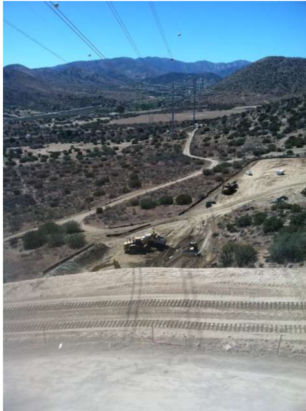
Figure 1: Grading activities at Construct 5, Segment 6A.
