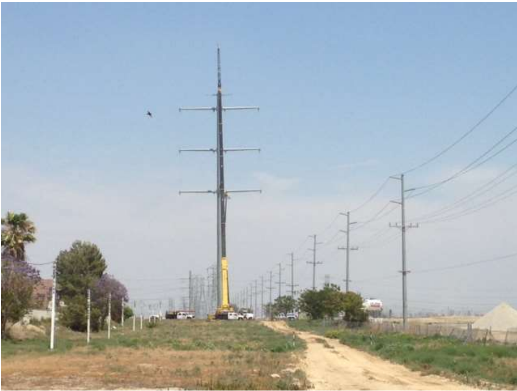
Figure 8: Crews assembling Tower M72-T2 in the City of Chino, Segment 8, Phase 3.
