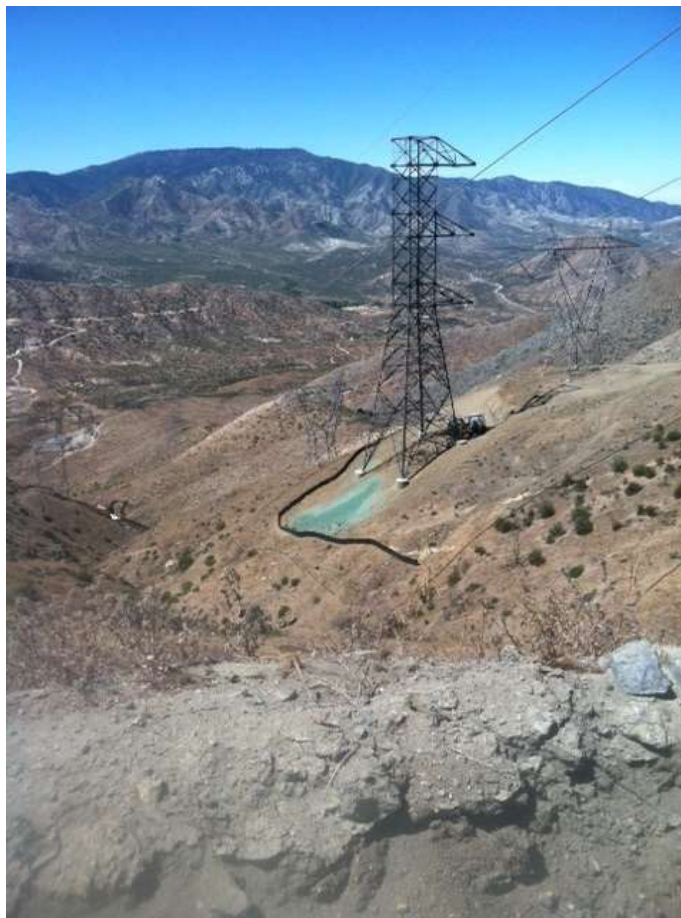
Figure 4: Hydromulching activities at Construct 9, Segment 11C.
