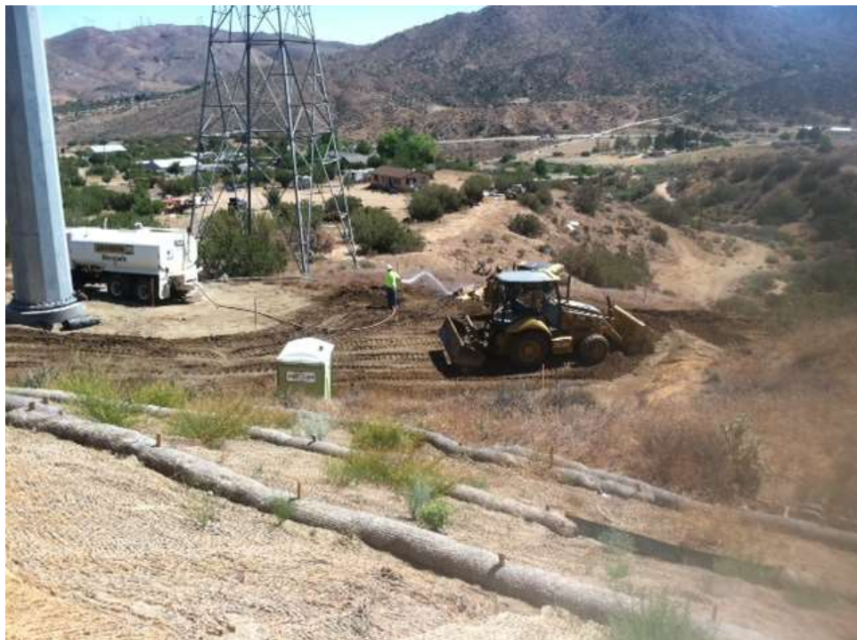
Figure 2: Grading activities at Construct 6, Segment 6A.
