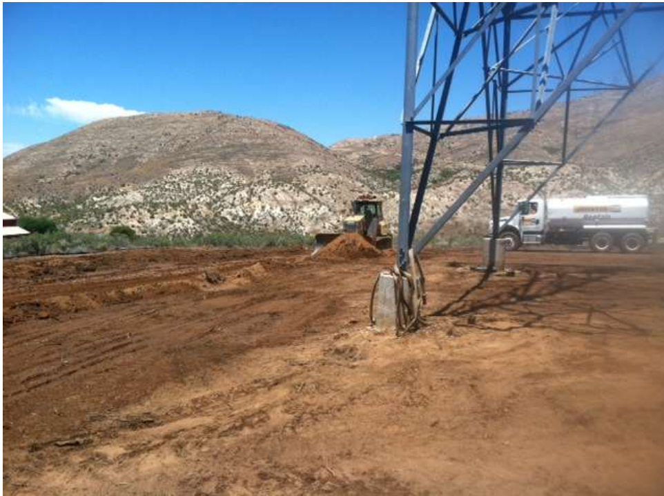
Figure 3: Grading activities at Construct 16, Segment 11C.
