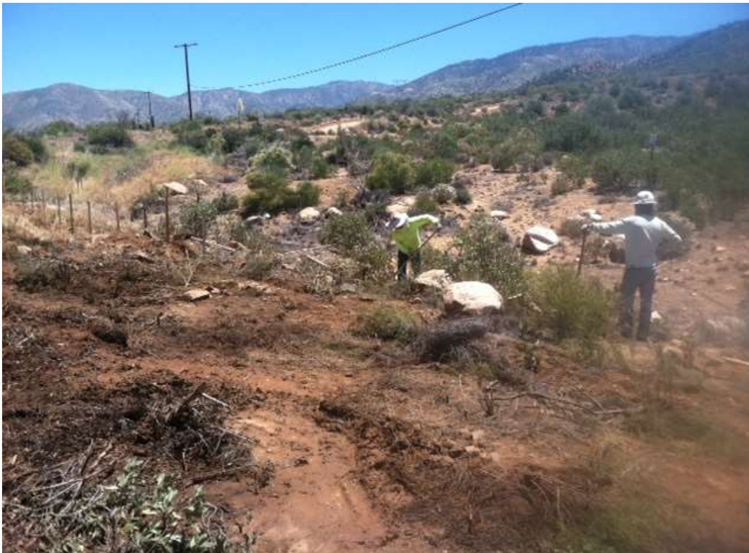
Figure 5: BMP installation at Construct 16, Segment 11C.
