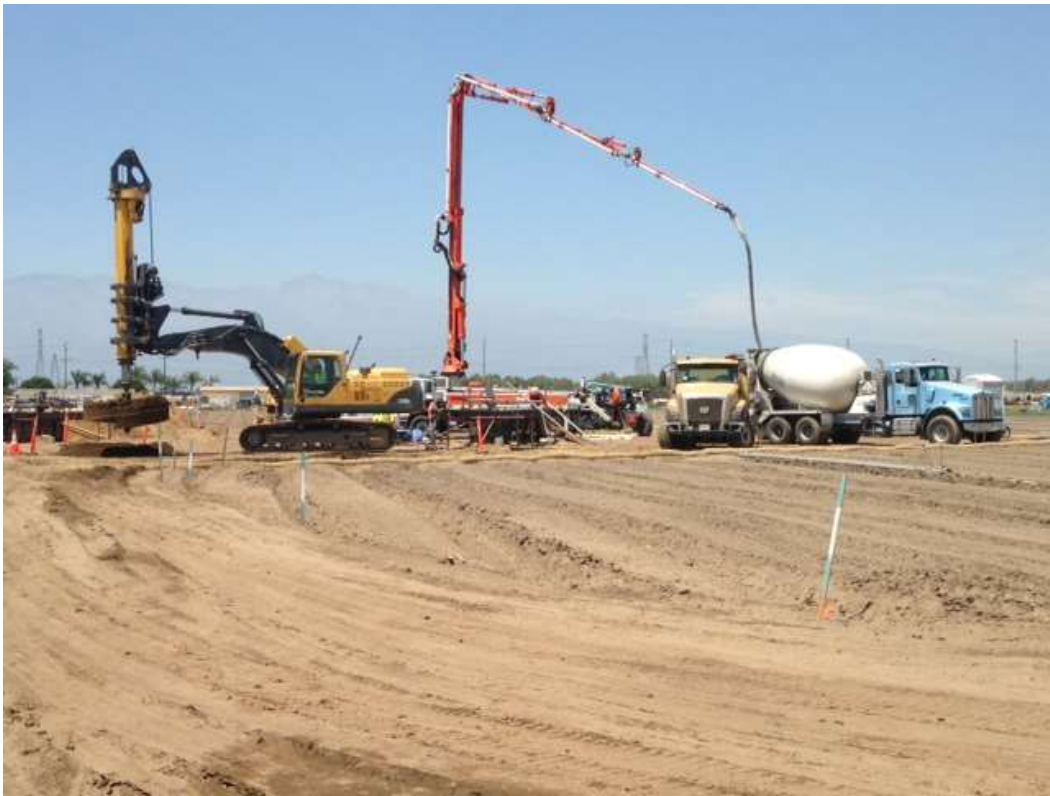
Figure 7: Tower foundation pouring at Tower M70-T6, Segment 8, Phase 3.
