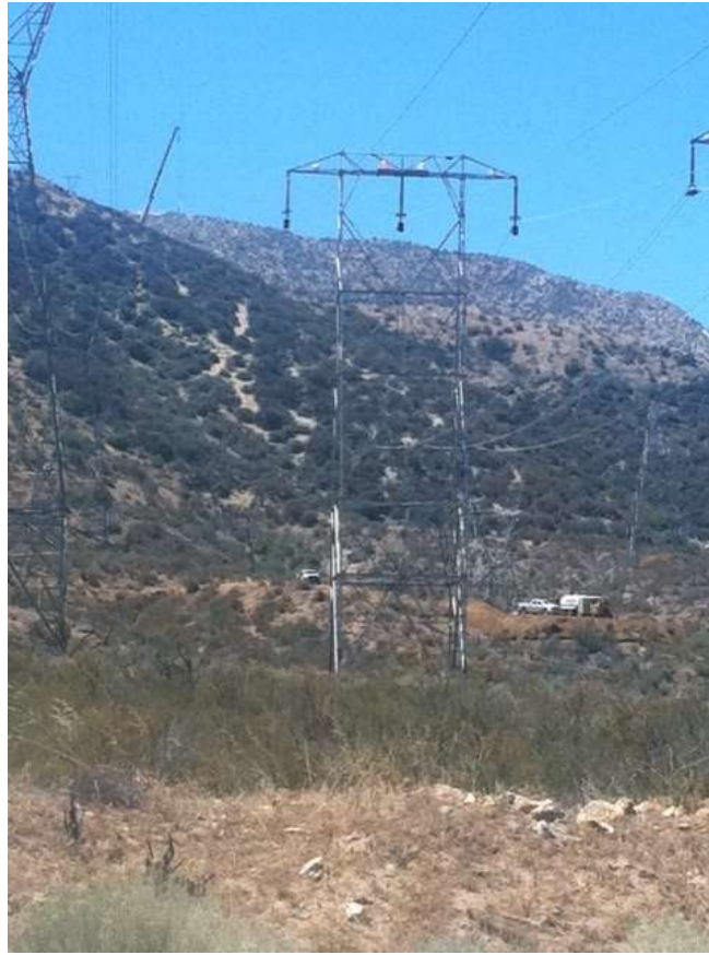
Figure 1: Wire removal activities at Constructs 17 and 18, Segment 11C.
