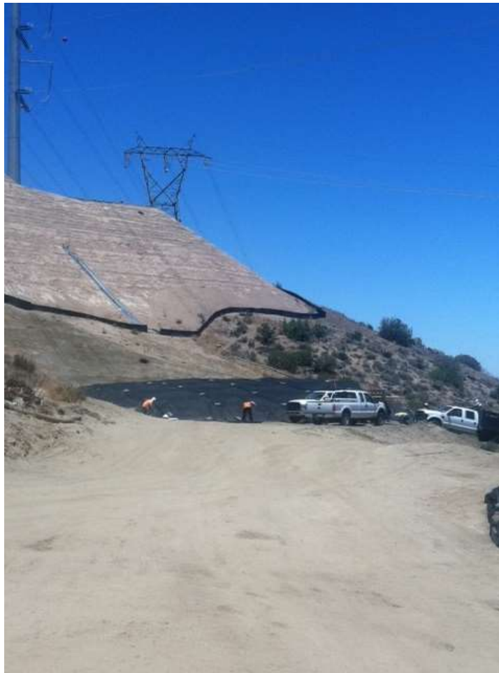
Figure 3: Stockpile covering activities at Construct 5, Segment 6A.
