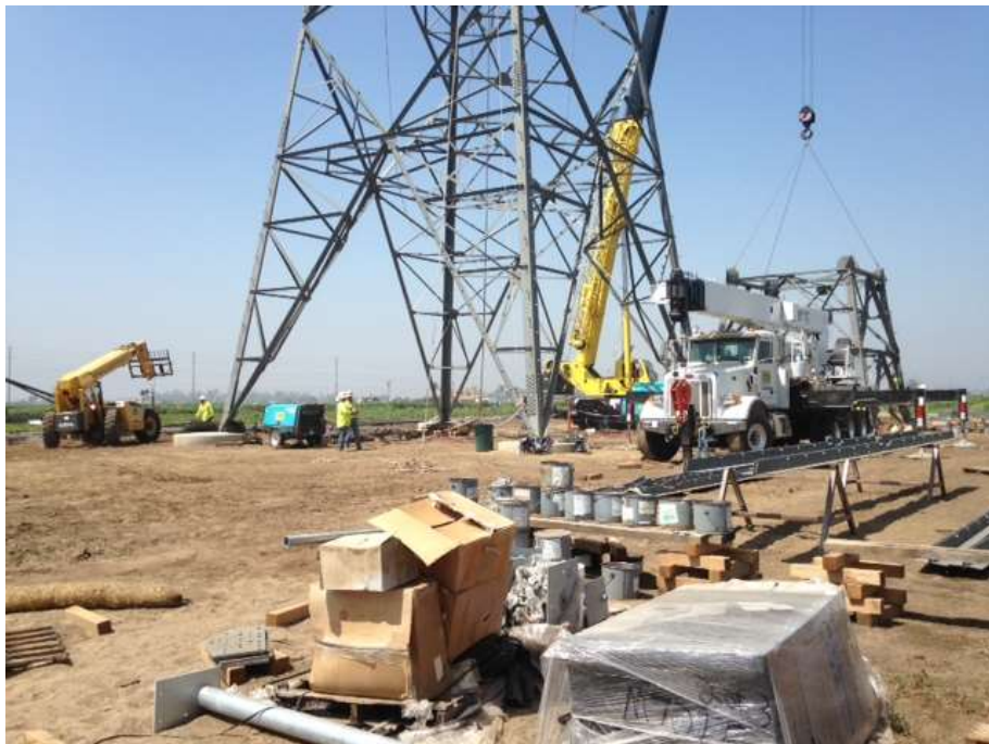
Figure 4: Tower assembly at Tower M70-T5, Segment 8, Phase 3.
