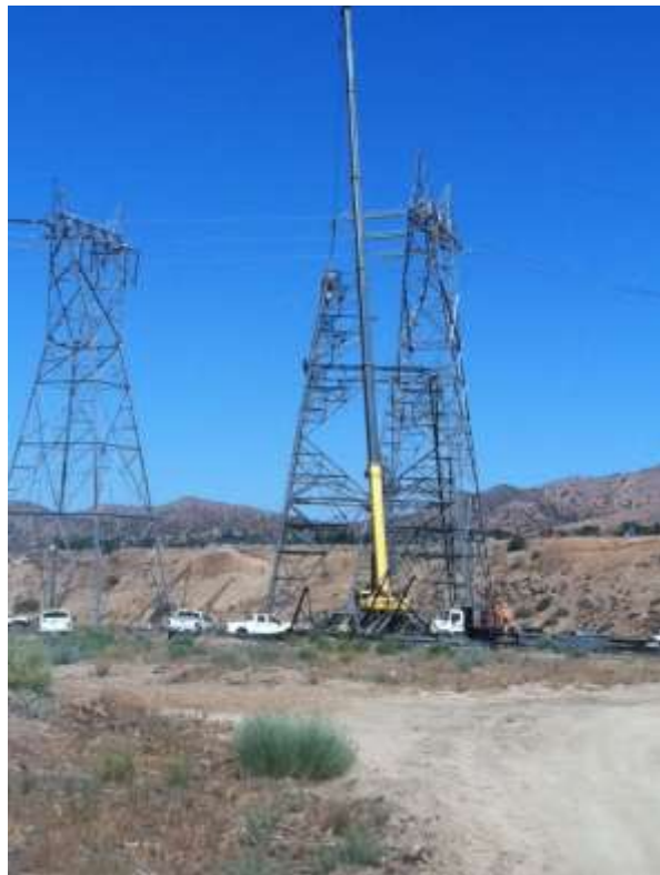
Figure 4: Tower assembly at Construct 1, Segment 11C.
