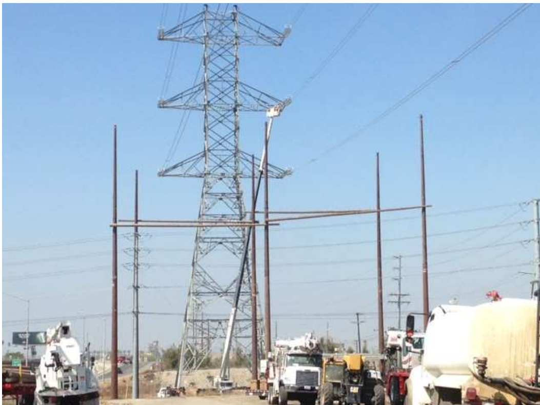
Figure 6: Wire pulling activities near the Rio Hondo Substation, Segment 7.
