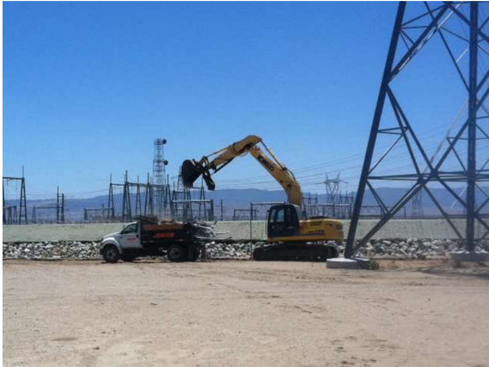
Figure 1: Fence removal at Whirlwind Substation.
