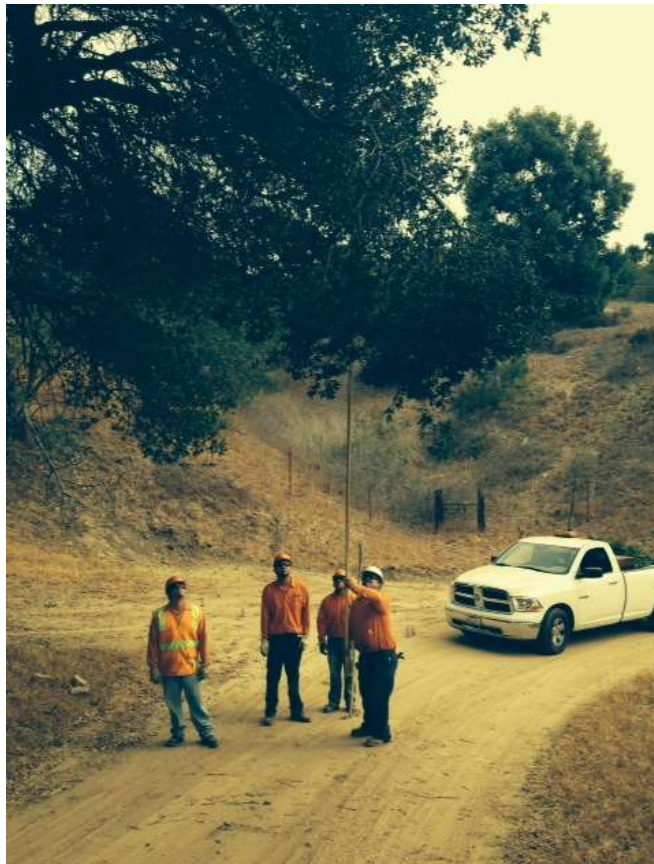
Figure 8: Tree trimming along access roads to allow access for large construction equipment, Segment 8, Phase 1.
