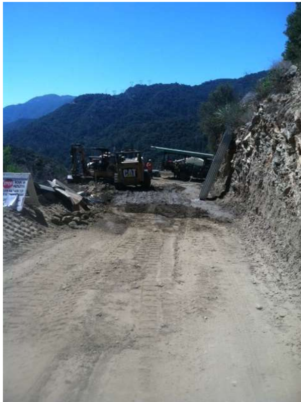
Figure 2: Grading and drainage operations along Loop Road L, Segment 6C.
