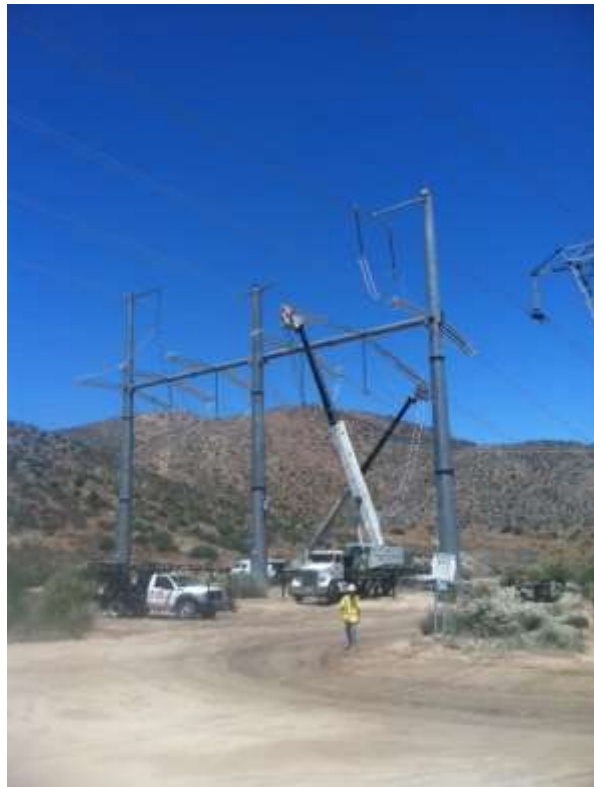
Figure 3: Wire activities at Construct 11, Segment 6A.
