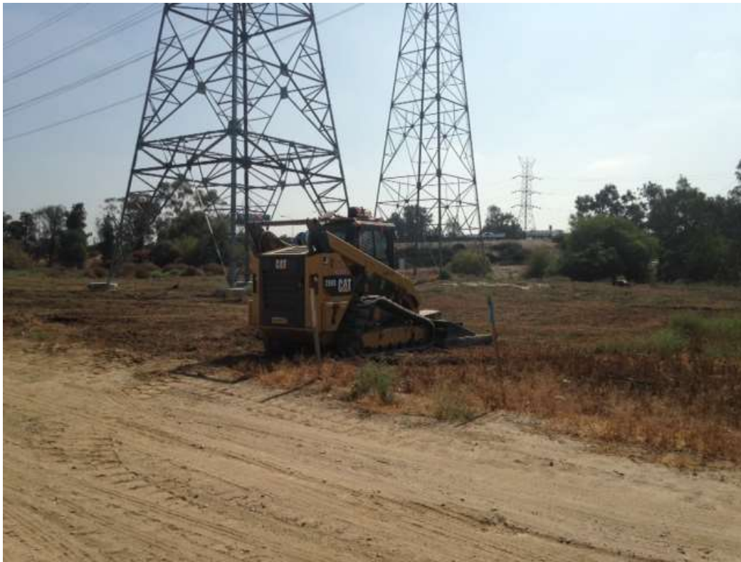
Figure 5: Vegetation mowing to prepare work areas prior to conductor installation, Segment 7.
