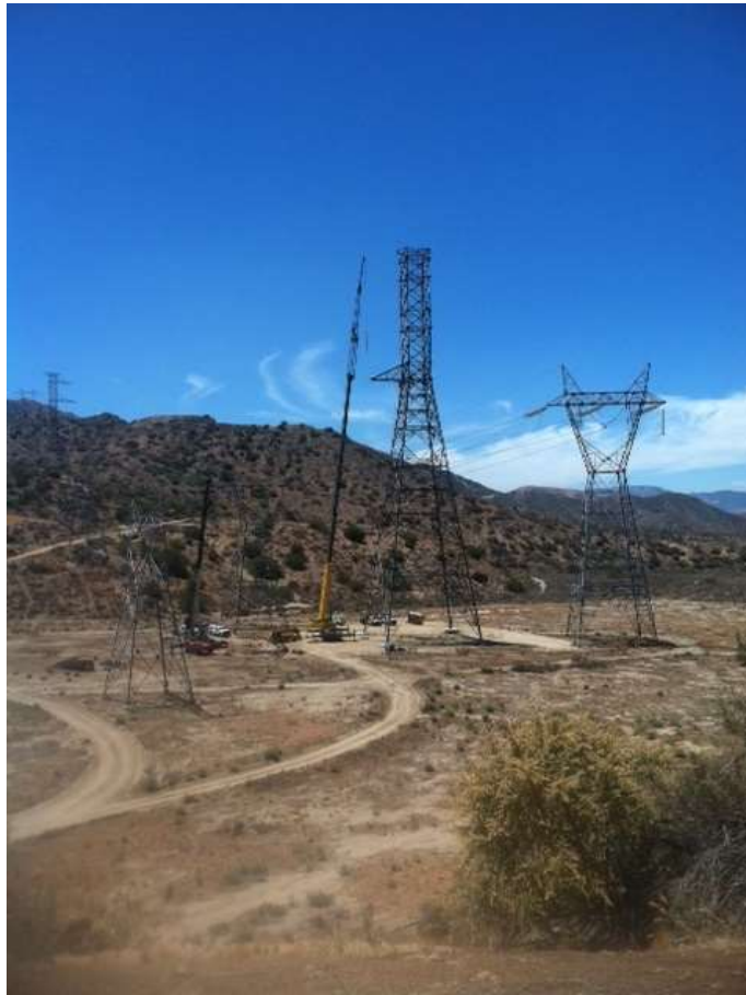
Figure 3: Erection activities at Construct 1, Segment 11C.
