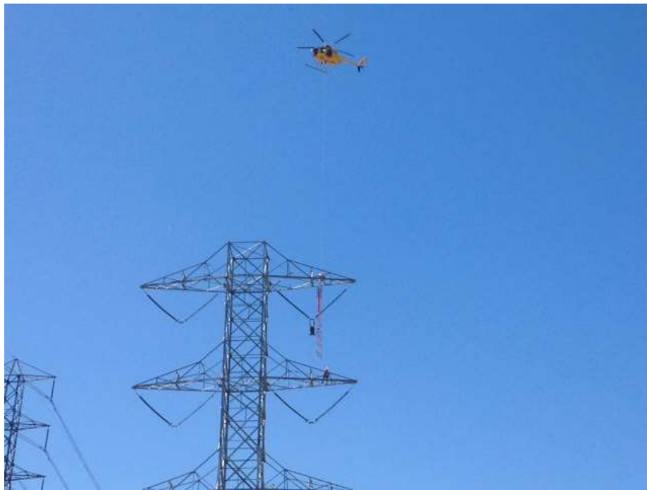
Figure 4: Helicopter delivering travelers in preparation for conductor installation, Segment 7.
