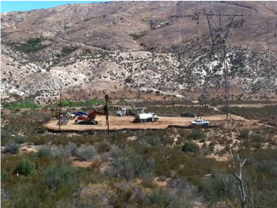
Figure 2: Foundation activities at Construct 15, Segment 11C.
