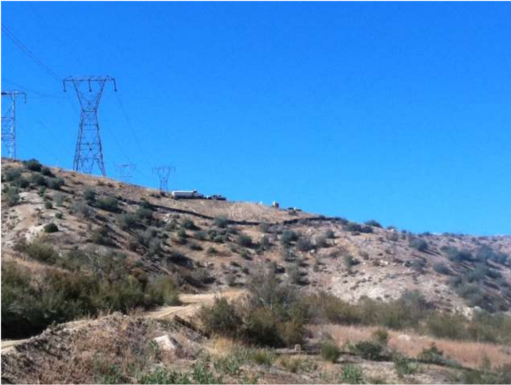
Figure 1: Grading activity at Construct 12, Segment 11C.
