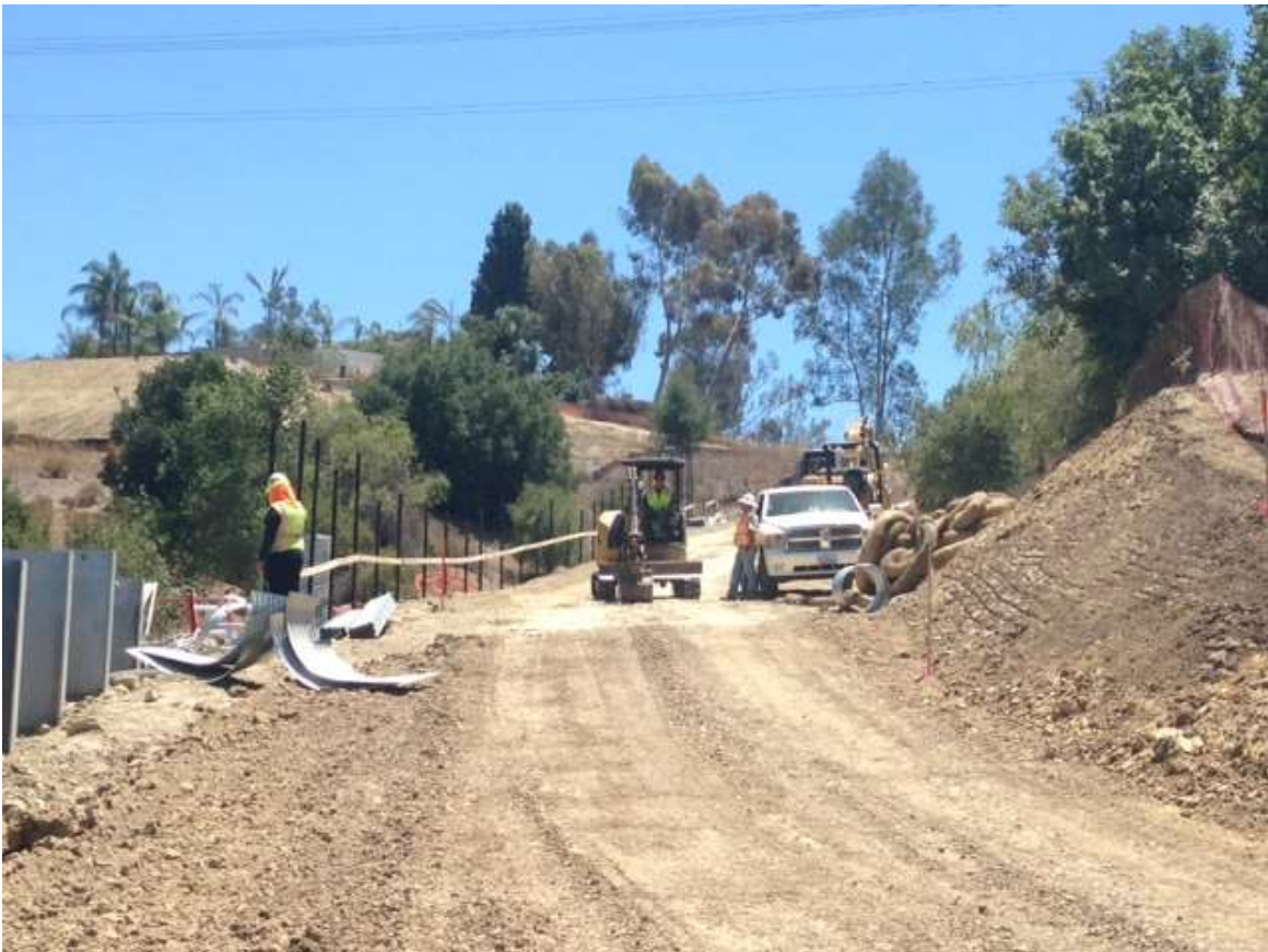
Figure 7: Wall construction and backfilling access road at Tower M49-T1, Segment 8, Phase 4.
