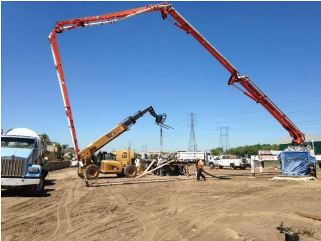
Figure 5: Foundation pouring at Tower M68-T1, Segment 8, Phase 3.
