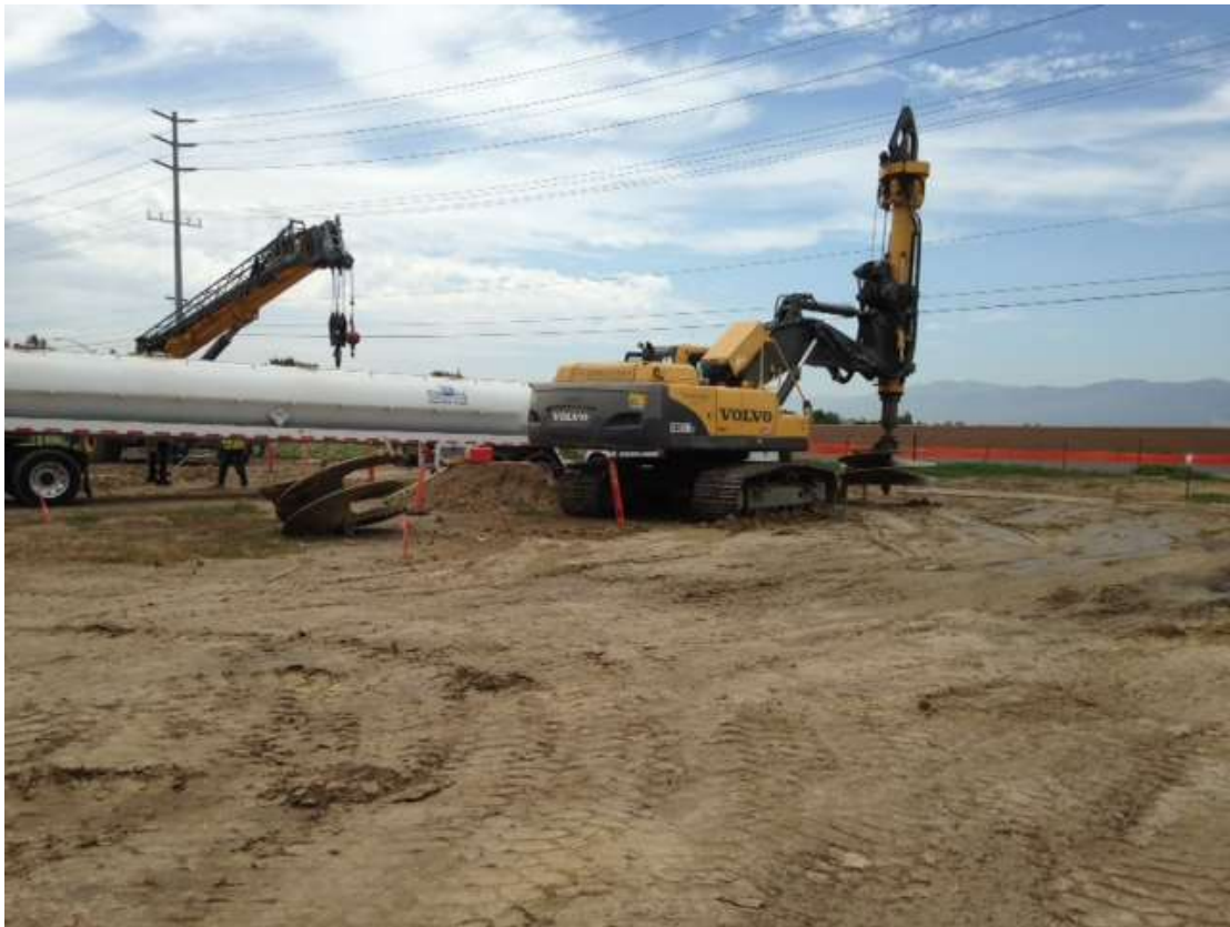
Figure 6: Foundation excavation at Tower M67-T4, Segment 8, Phase 3.
