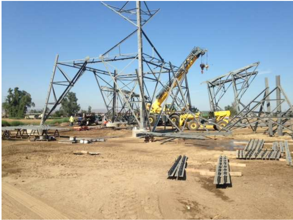
Figure 7: Assembly at Tower M68-T5, Segment 8, Phase 3.
