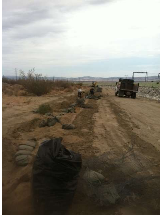
Figure 1: BMP removal at Whirlwind Substation.
