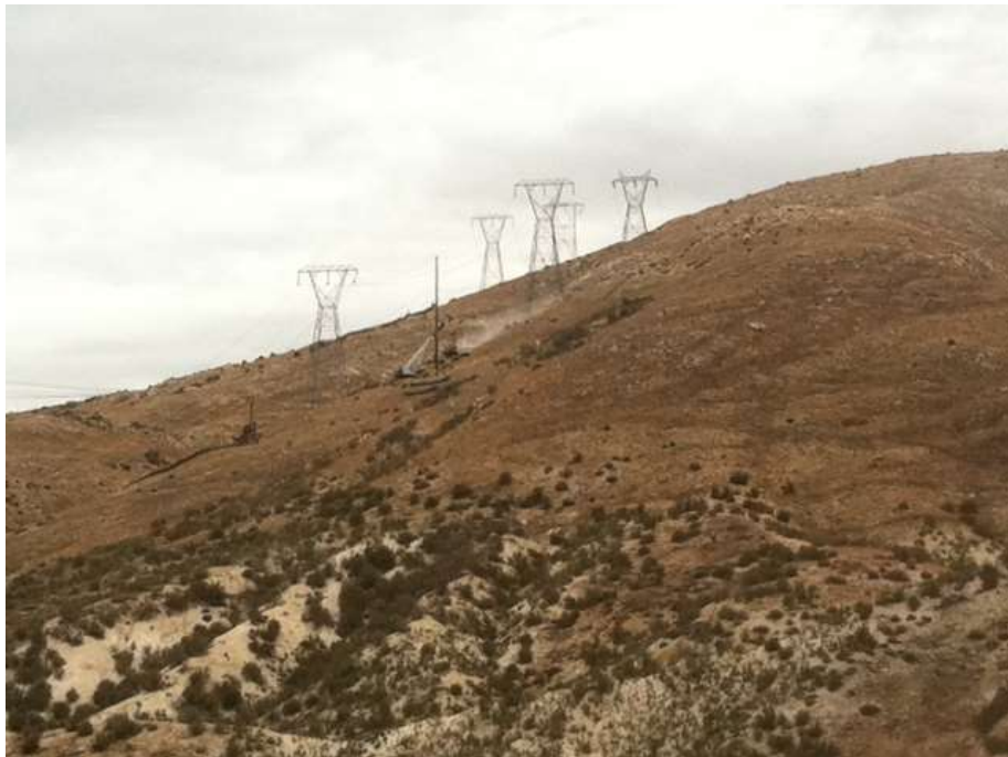
Figure 2: Foundation activities (micropile) at Construct 14, Segment 11C.
