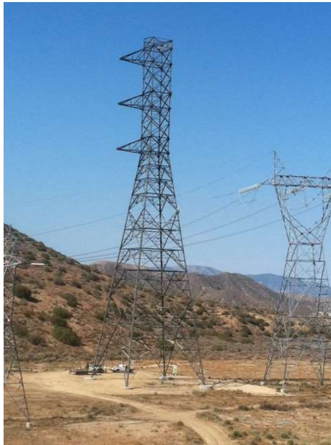
Figure 3: QA/QC activities at Construct 1, Segment 11C.
