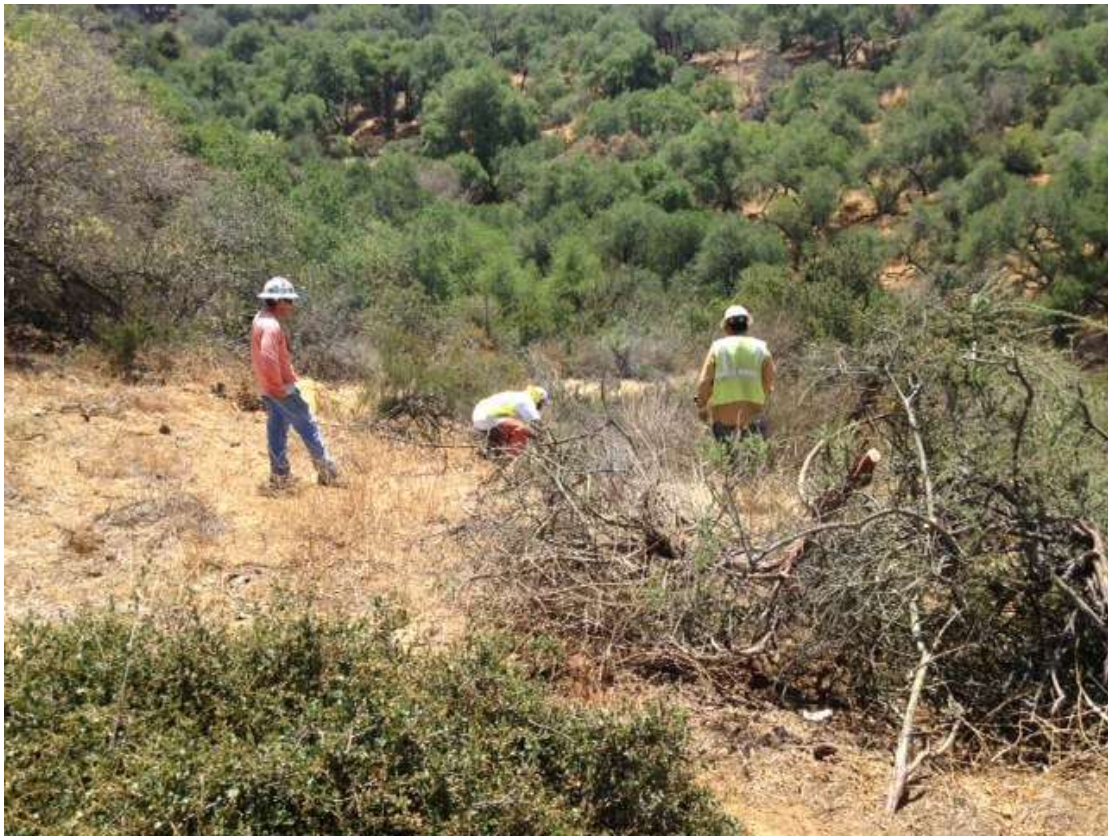
Figure 5: Vegetation clearing at Tower M52-T2, Segment 8, Phase 4.
