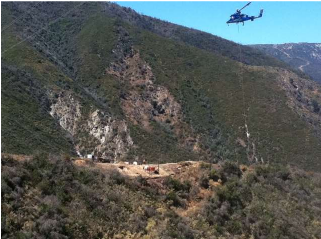
Figure 6: Foundation (micropile) activity at Construct 58, Segment 11C.
