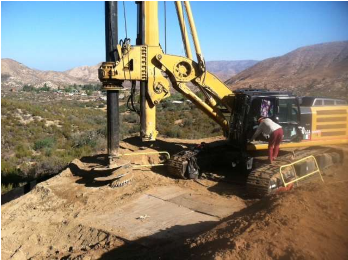
Figure 5: Foundation activities at Construct 15, Segment 11C.
