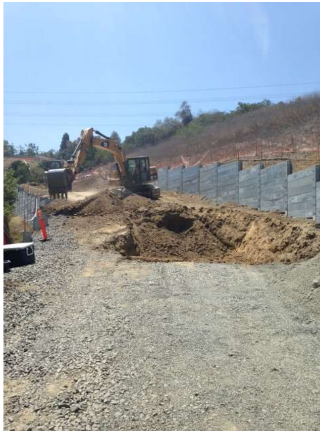
Figure 10: Road grading at Tower M49-T1, Segment 8, Phase 4.
