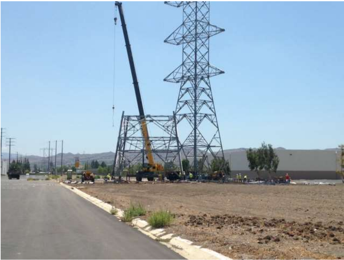
Figure 9: Tower assembly at Tower M65-T3, Segment 8, Phase 1.
