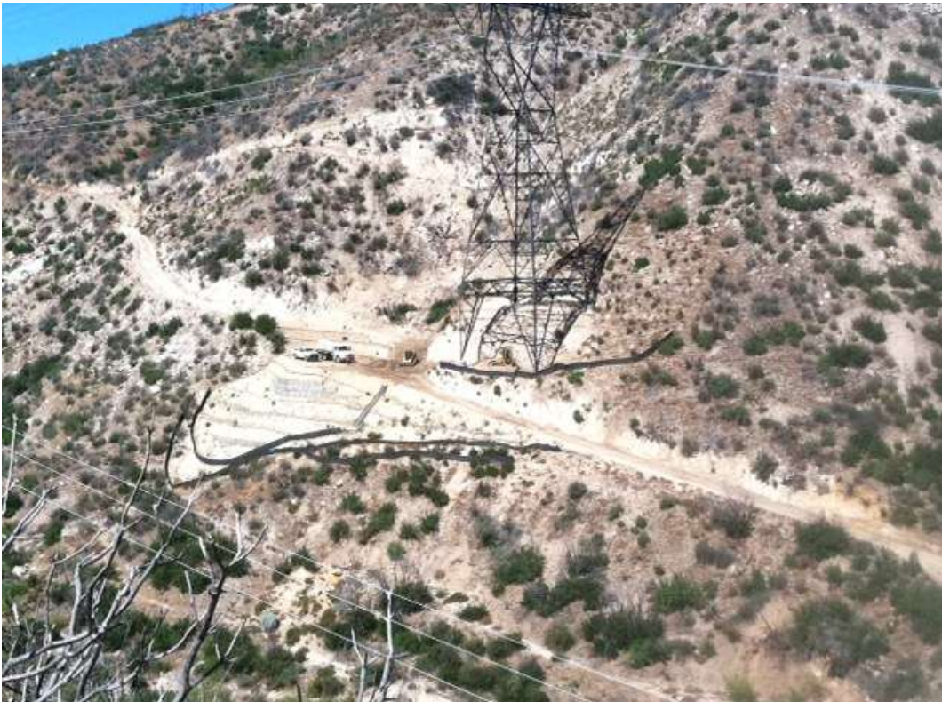
Figure 2: Restoration grading activities at Construct 33, Segment 6A.
