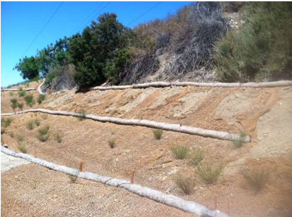
Figure 4: BMP deficiencies at Chaney Trails Pullsite, Segment 11B.
