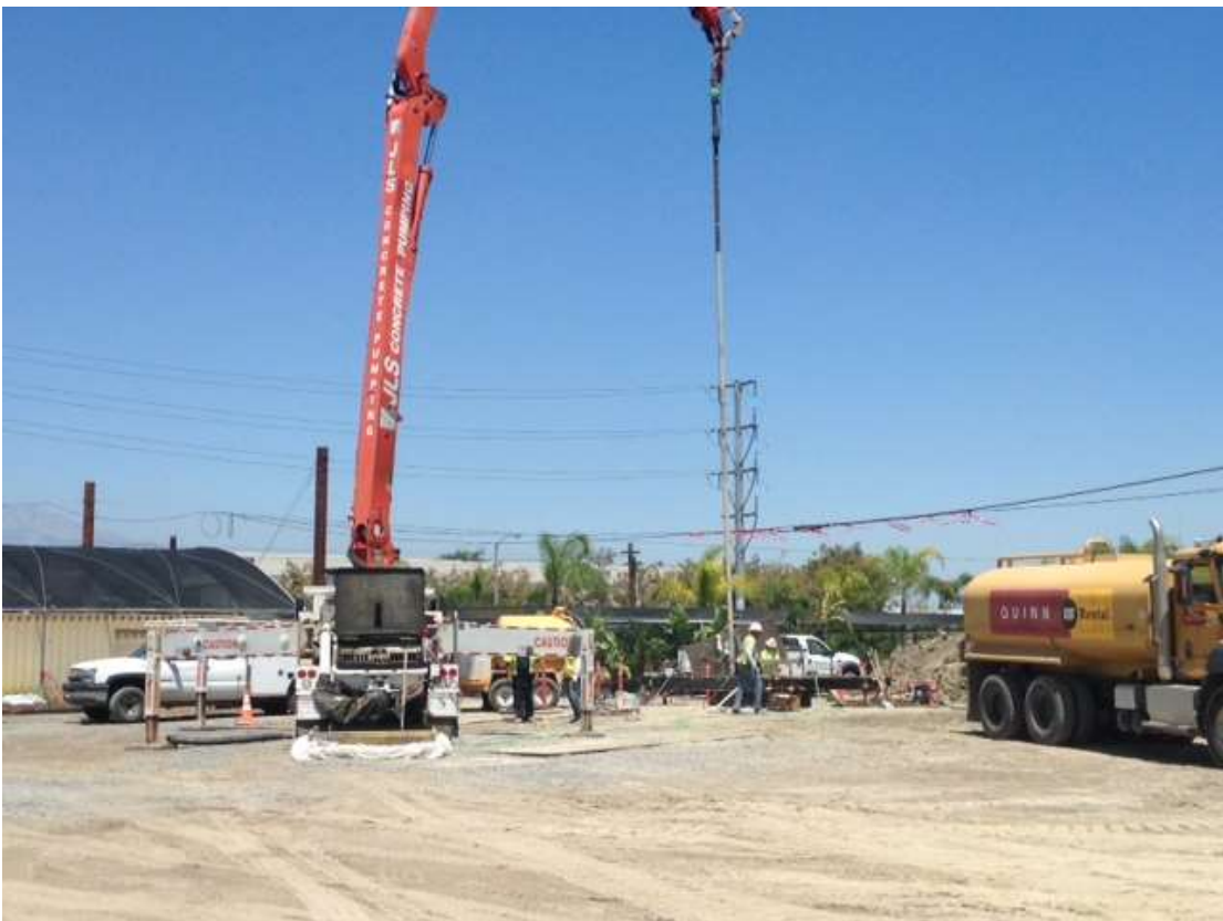
Figure 10: Concrete pour of Tower M66-T1 foundations, Segment 8, Phase 3.
