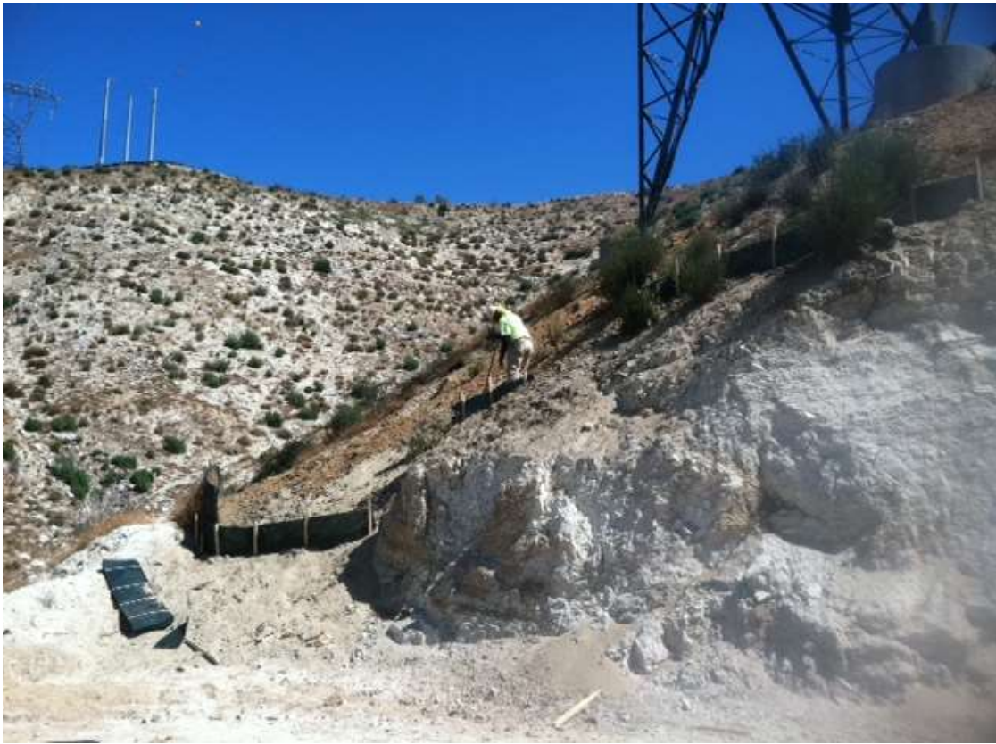
Figure 3: BMP maintenance at Construct 20, Segment 6A.
