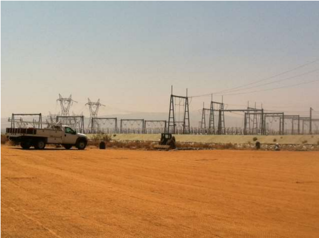
Figure 1: BMP removal at Whirlwind Substation.
