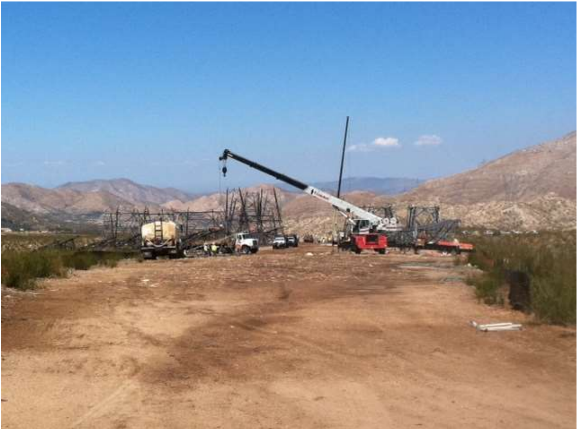
Figure 7: Erection activities at Aliso Canyon HAY, Segment 11C.
