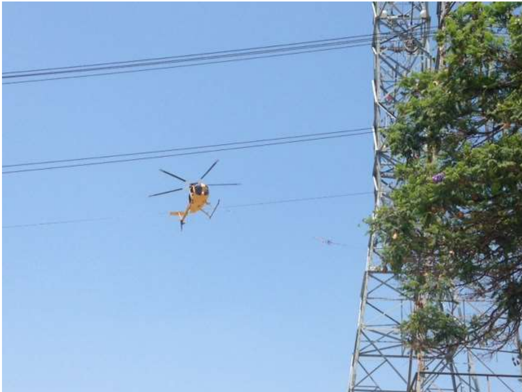
Figure 8: Wire pulling activities in Duarte, Segment 7.
