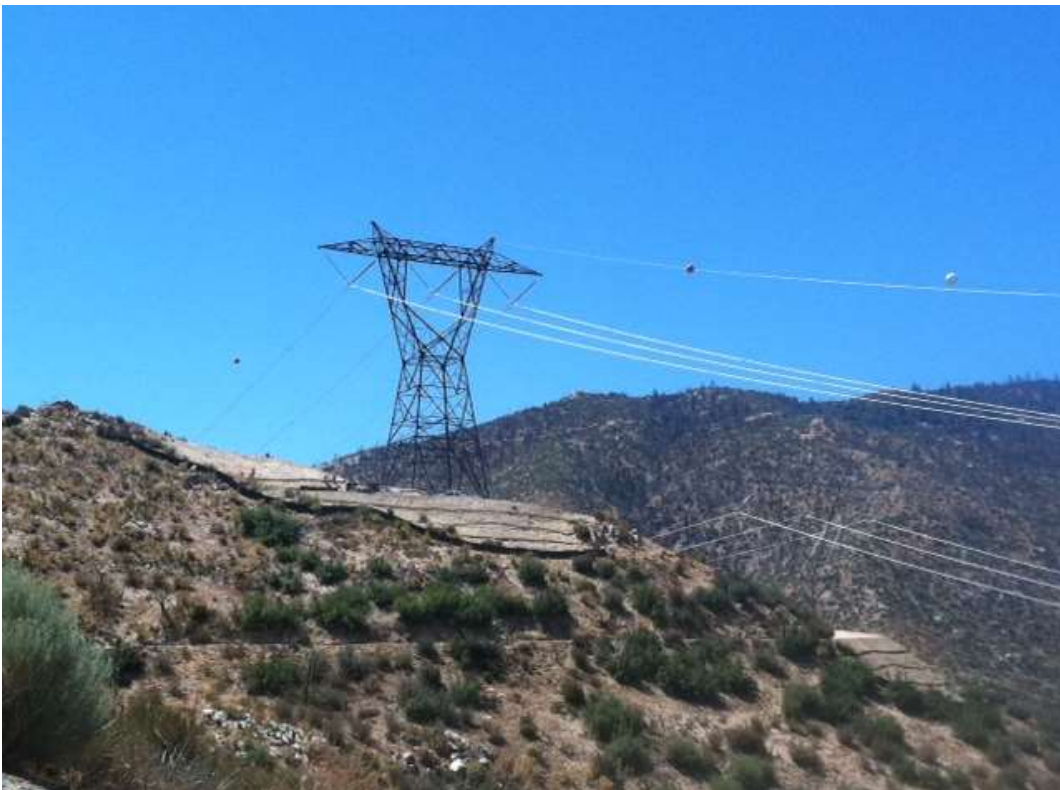
Figure 2: BMP installation at Construct 24, Segment 6A.
