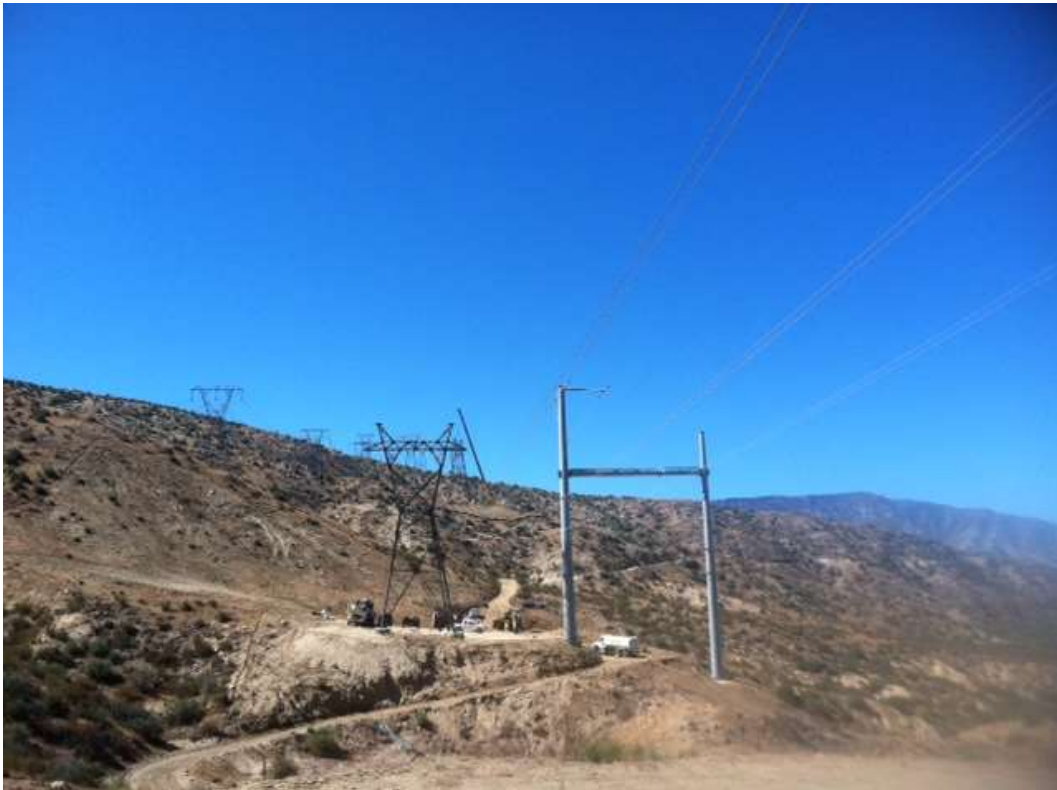
Figure 3: Erection activity at Construct 12 and 13, Segment 11C.
