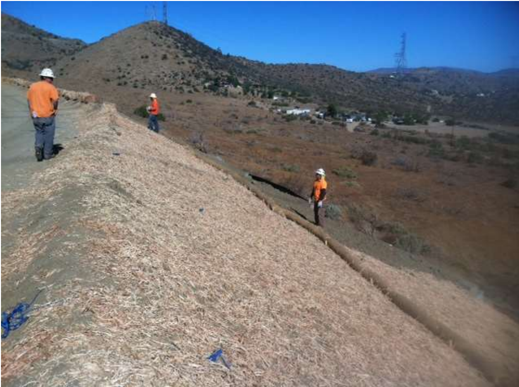
Figure 1: BMP installation (wood straw) at Construct 8, Segment 6A.
