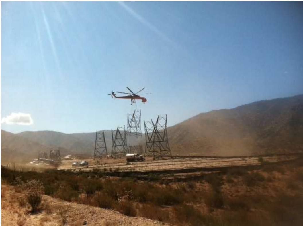
Figure 3: Erection activities at Aliso Canyon HAY, Segment 11C.
