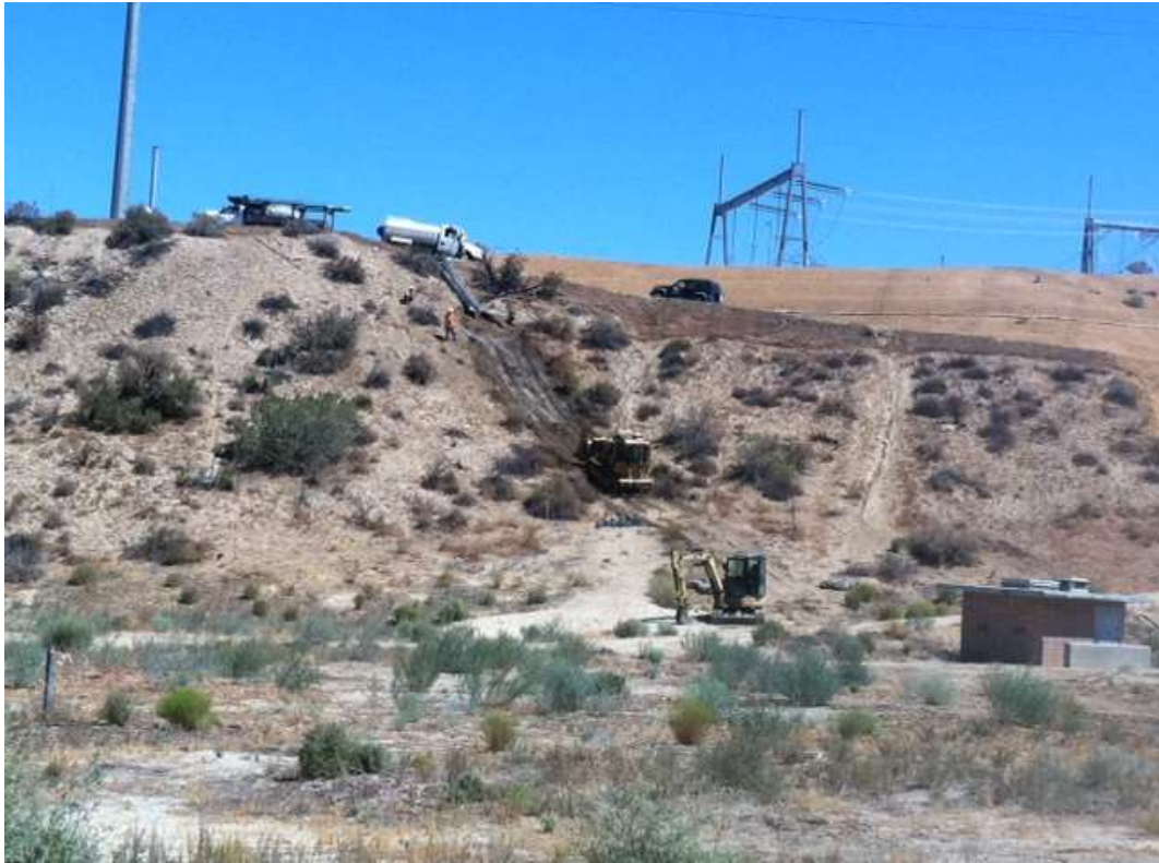
Figure 1: Drainage improvement at Construct 1, Segment 6A.
