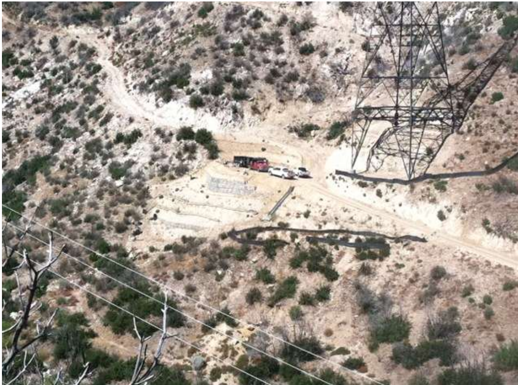
Figure 2: BMP removal at Construct 33, Segment 6A.
