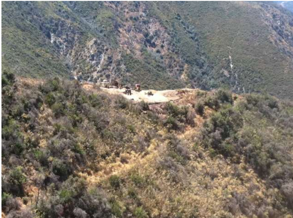
Figure 2: Foundation activity at Construct 58, Segment 11C.
