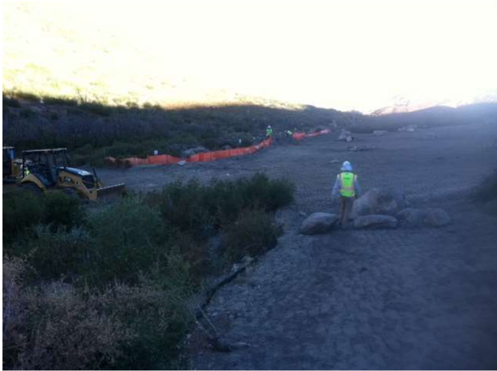
Figure 1: Recontouring and topsoil reapplication at Pull/Tension Site 28/29, Segment 6A.
