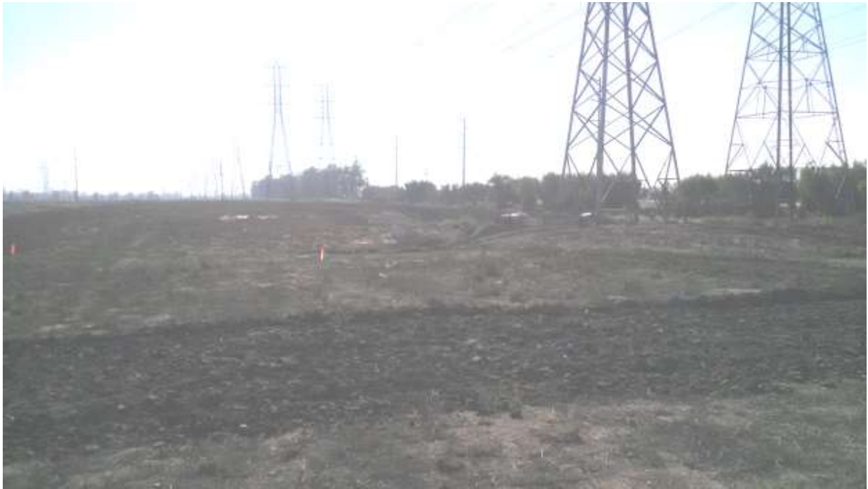
Figure 3: Staking verification of proposed work areas in Segment 8, Phase 3.
