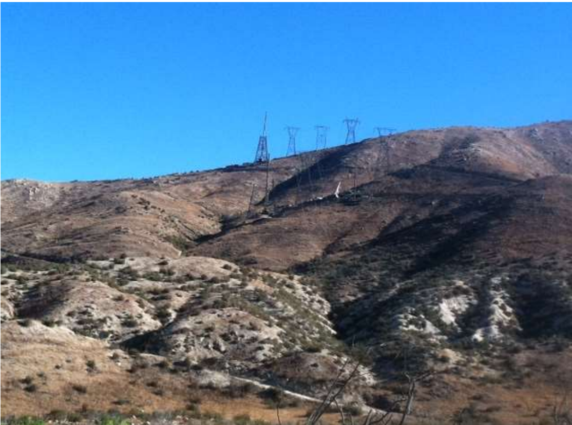
Figure 2: Erection activity at Construct 13 and 14, Segment 11C.
