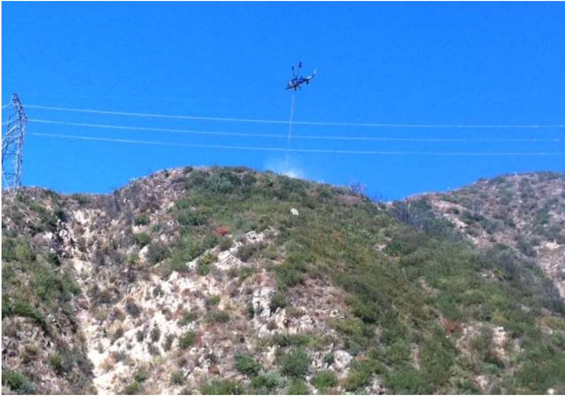
Figure 1: Foundation activities at Construct 61, Segment 11C.
