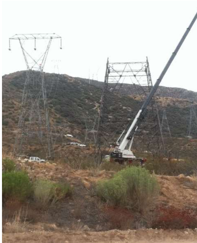
Figure 2: Erection activity at Construct 15, Segment 11C.
