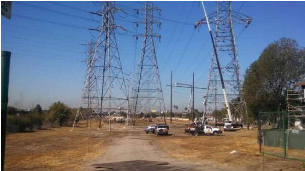
Figure 4: Helicopter supporting wire stringing operations near Segment 7, Tower M37-T3. Biological Monitors were on site to measure noise generated by construction adjacent to the least Bell's vireo territory in compliance with Mitigation Measure B-15.
