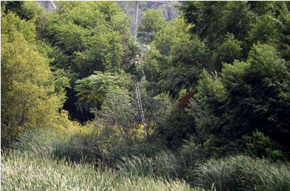
Figure 3: Photo of the dropped conductor and damage to least Bell's vireo habitat that occurred on September 7 when the conductor fell across the San Gabriel River between Towers M37-T3 and M37-T4, Segment 7. (Photo courtesy of FRED)
