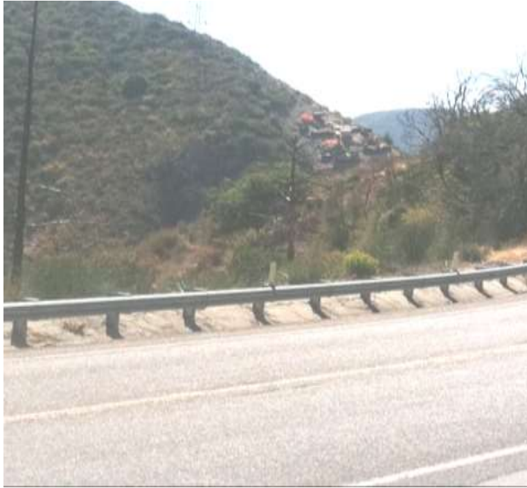
Figure 1: Foundation activities at Construct 62, Segment 11C.
