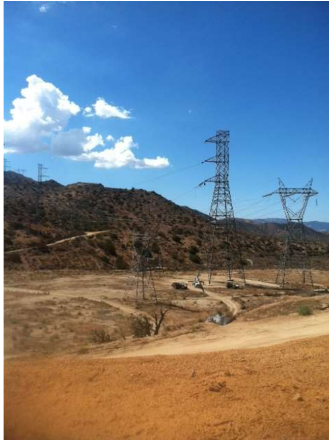
Figure 1: Wire stringing activities at Construct 1, Segment 11C.
