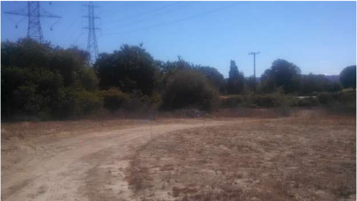
Figure 3: TRTP crews began utilizing the access road prior to staking being verified by the CPUC EM.
