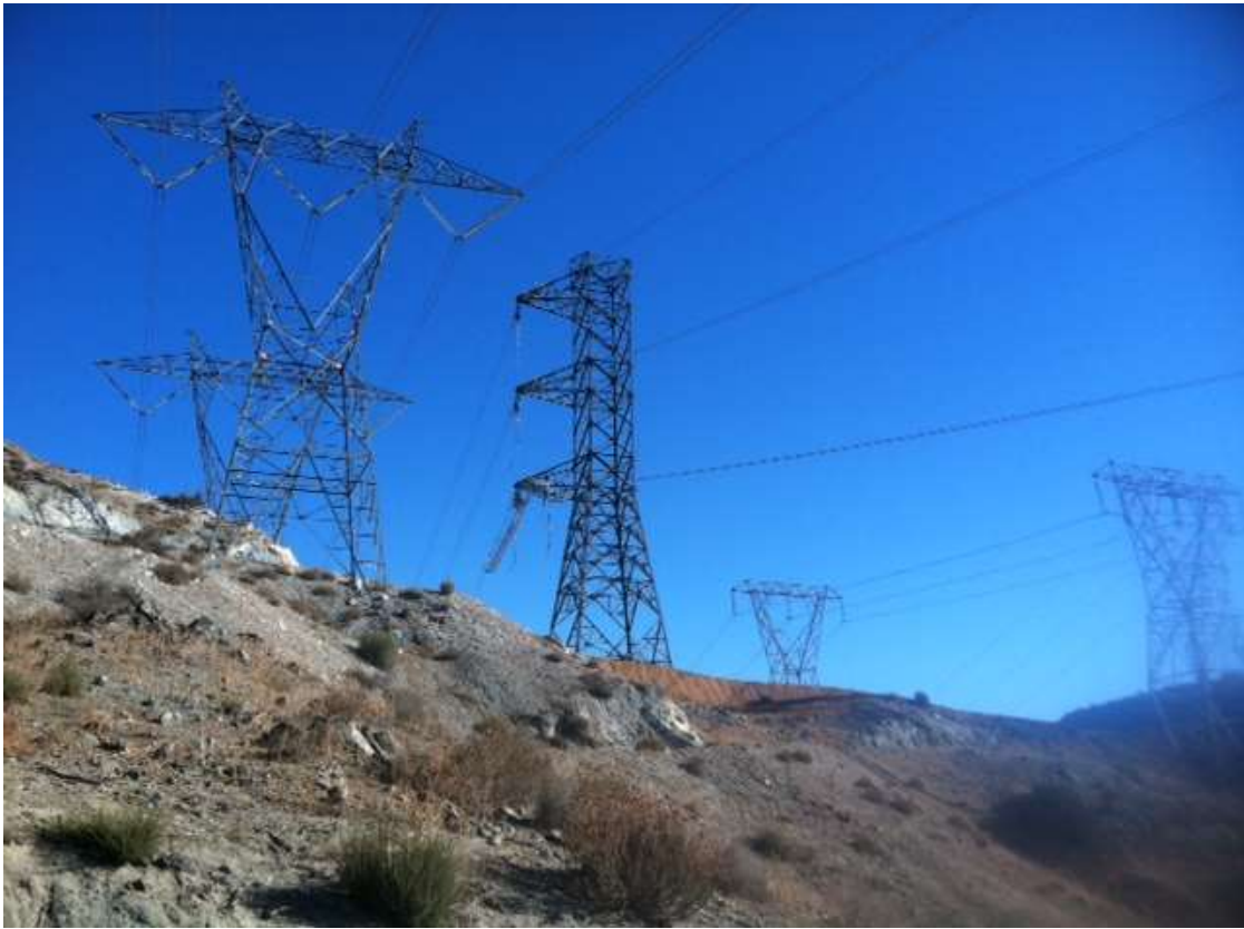
Figure 3: Wire stringing activities occurring at Construct 9, Segment 11C.
