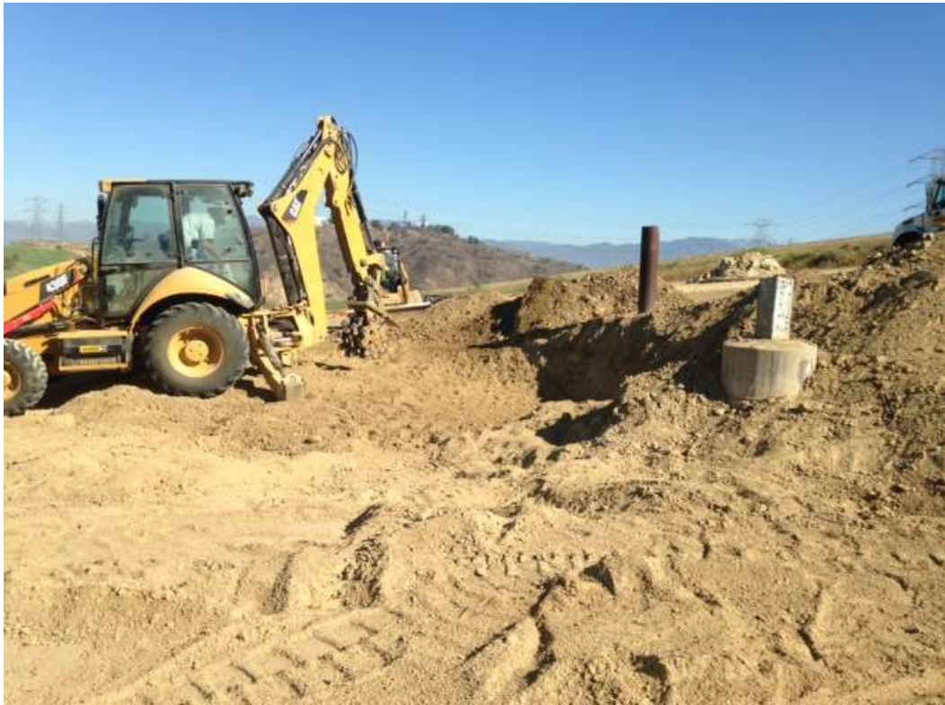
Figure 7: Foundation removal at Tower M7-T2 near Rose Hills, Segment 8, Phase 4.
