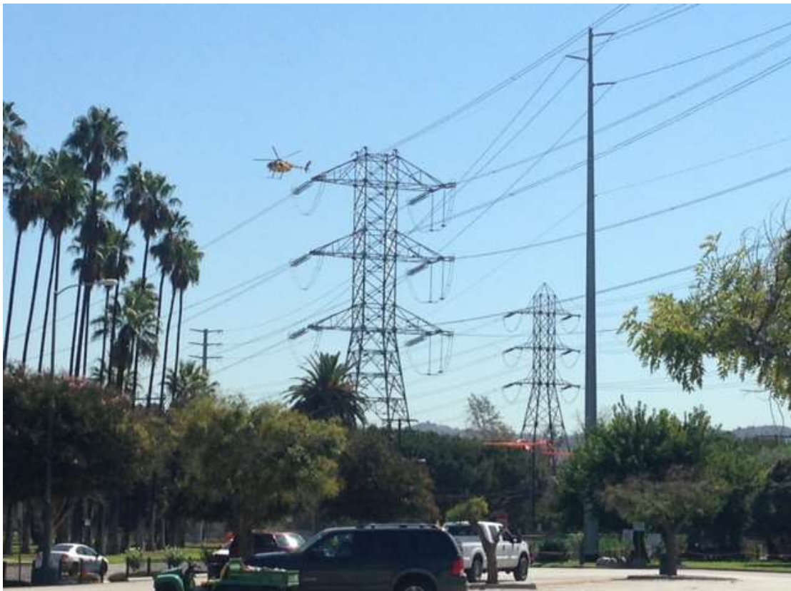
Figure 5: Wire stringing activities near Legg Lake, Segment 7.
