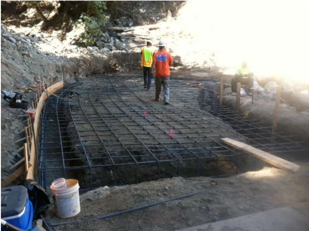
Figure 1: Wet crossing installation at Civil ID 153, Segment 6C.
