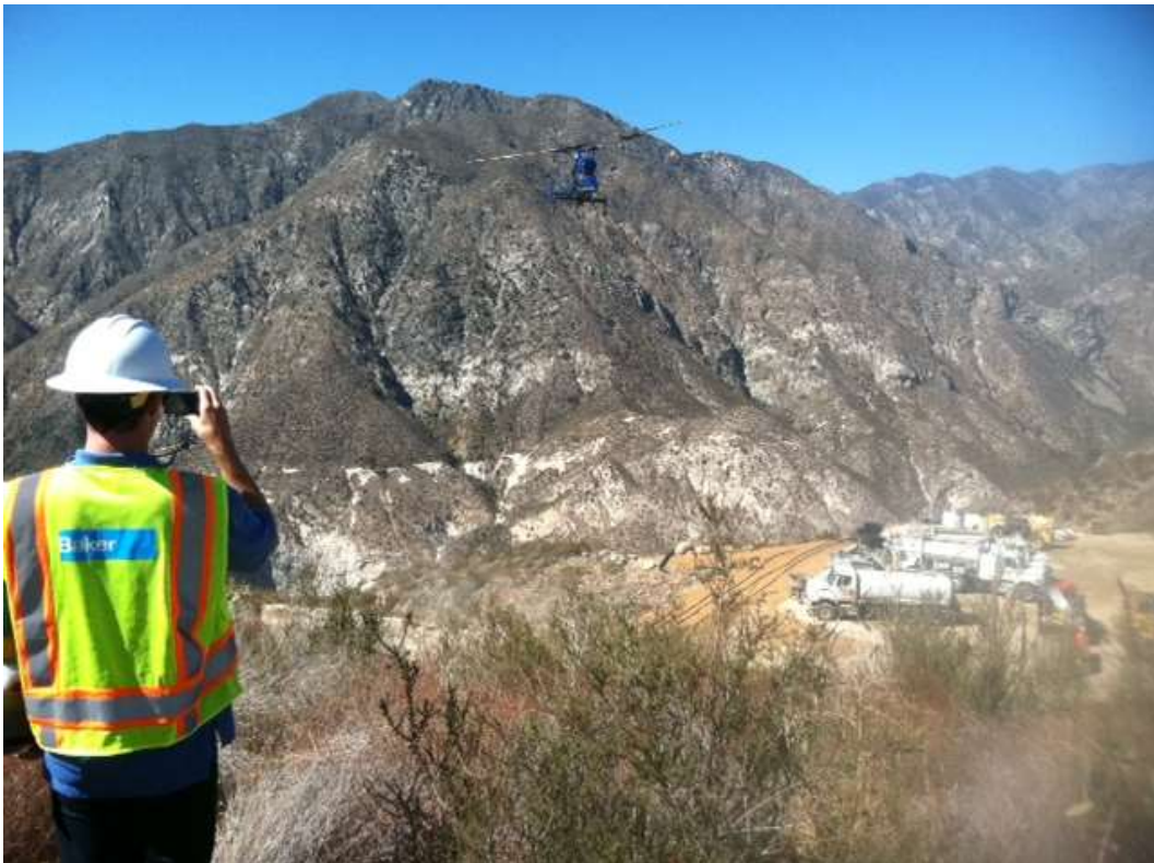
Figure 2: Foundation related activities occurring at Construct 53/54, Segment 11C.
