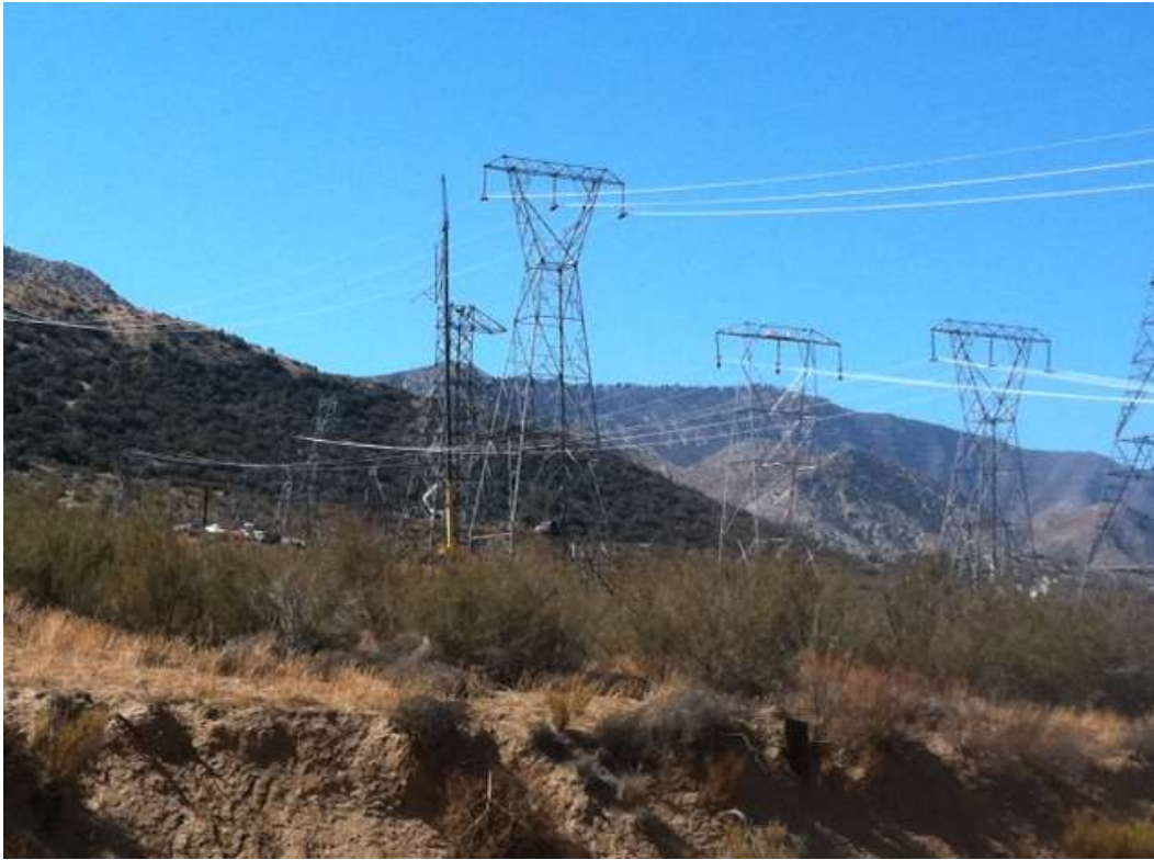
Figure 1: Erection activity at Construct 16, Segment 11C.
