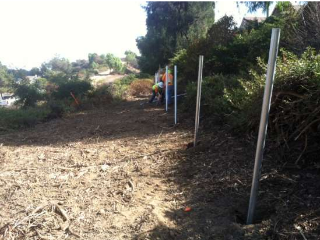
Figure 4: Fencing installation along the right-of-way for the Chino Hills Underground.
