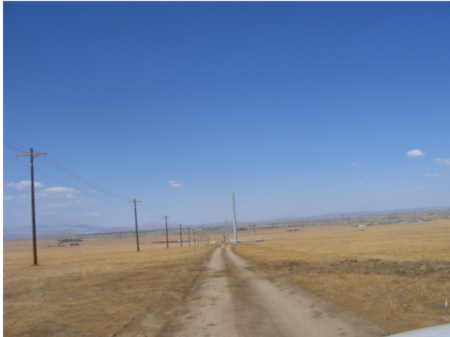
Figure 2: A new tubular steel pole (TSP) being erected along Section 3 near the Antelope Substation.
