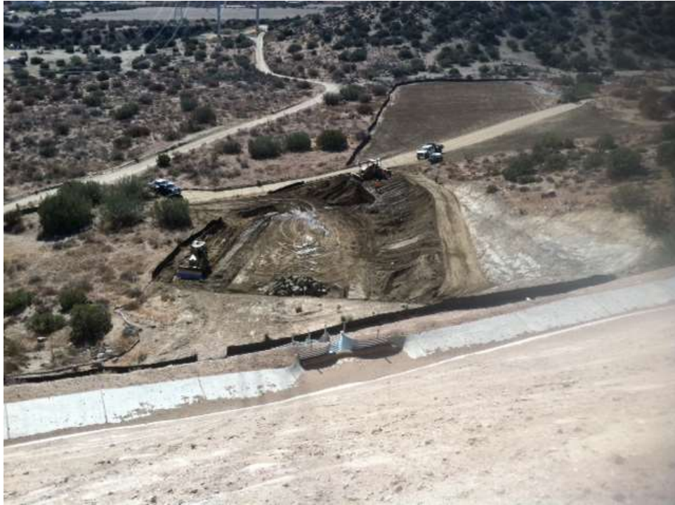
Figure 1: Grading activity at Construct 5/6, Segment 6A.
