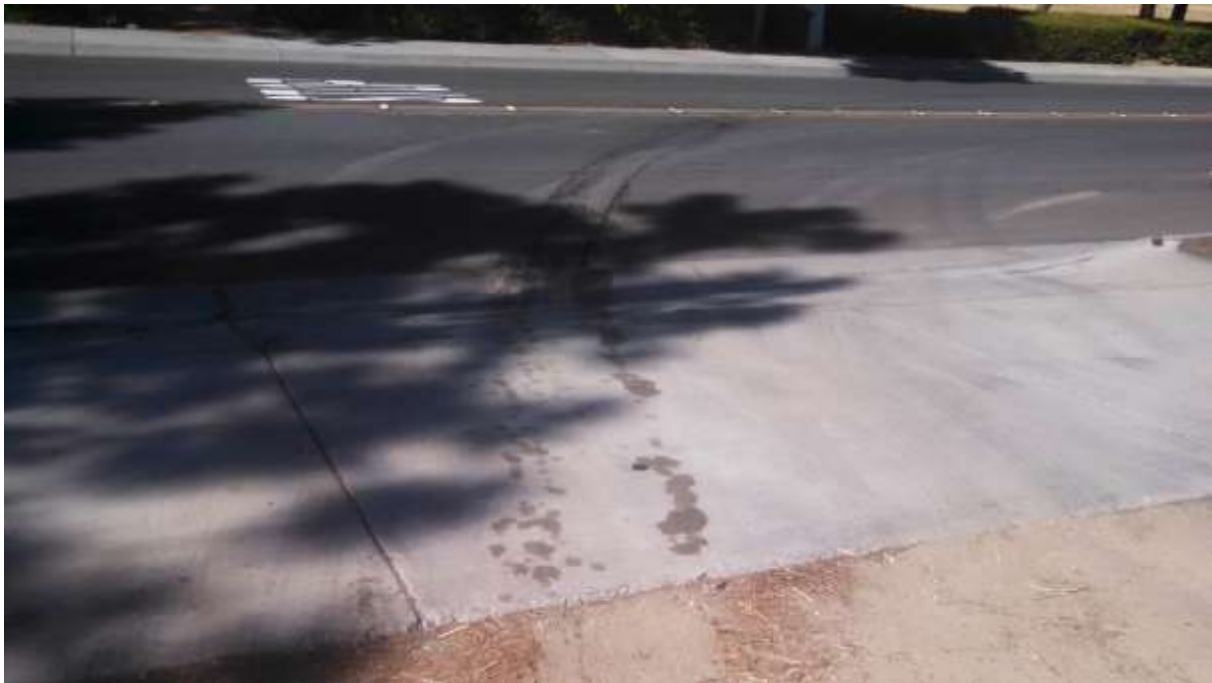
Figure 4: The CPUC EM observed a diesel fuel leak from project equipment exiting onto Eucalyptus Avenue in Chino Hills. The spill was immediately reported to SCE and remediation actions were taken.
