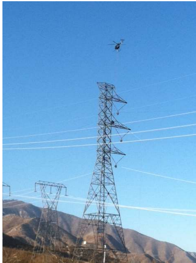
Figure 2: Wire stringing operations on Construct 15, Segment 11C.
