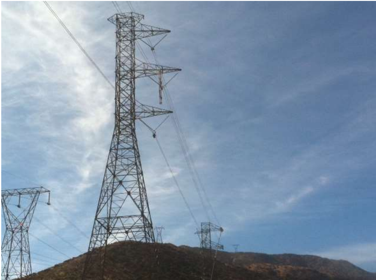
Figure 3: Wire Stringing activities at Constructs 15 and 16, Segment 11C.
