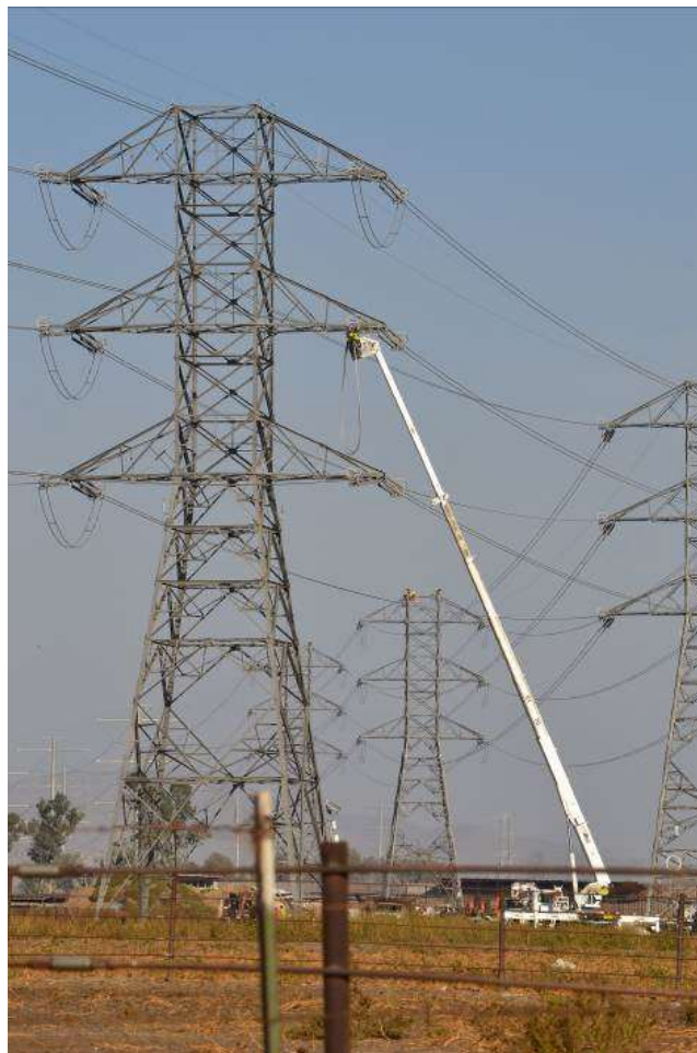
Figure 4: Jumper installation at dead end tower in Segment 8, Phase 3.
