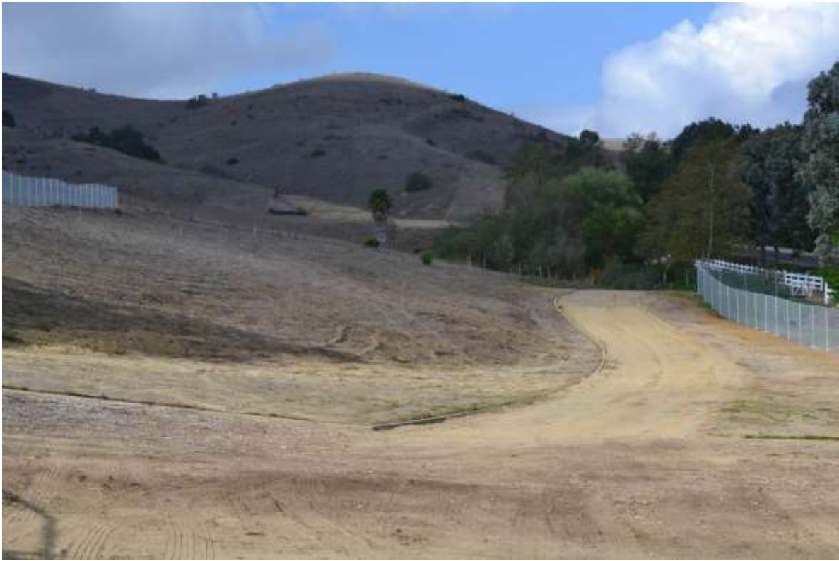
Figure 7: Temporary right-of-way fencing installation continues along the CHUG right-of-way.
