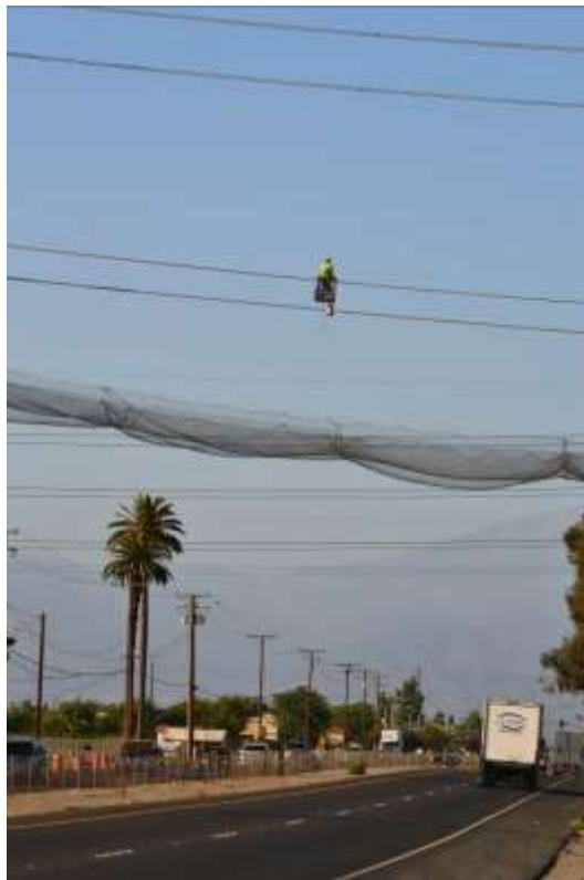
Figure 5: Spacer installation above Euclid Avenue, Segment 8, Phase 3.
