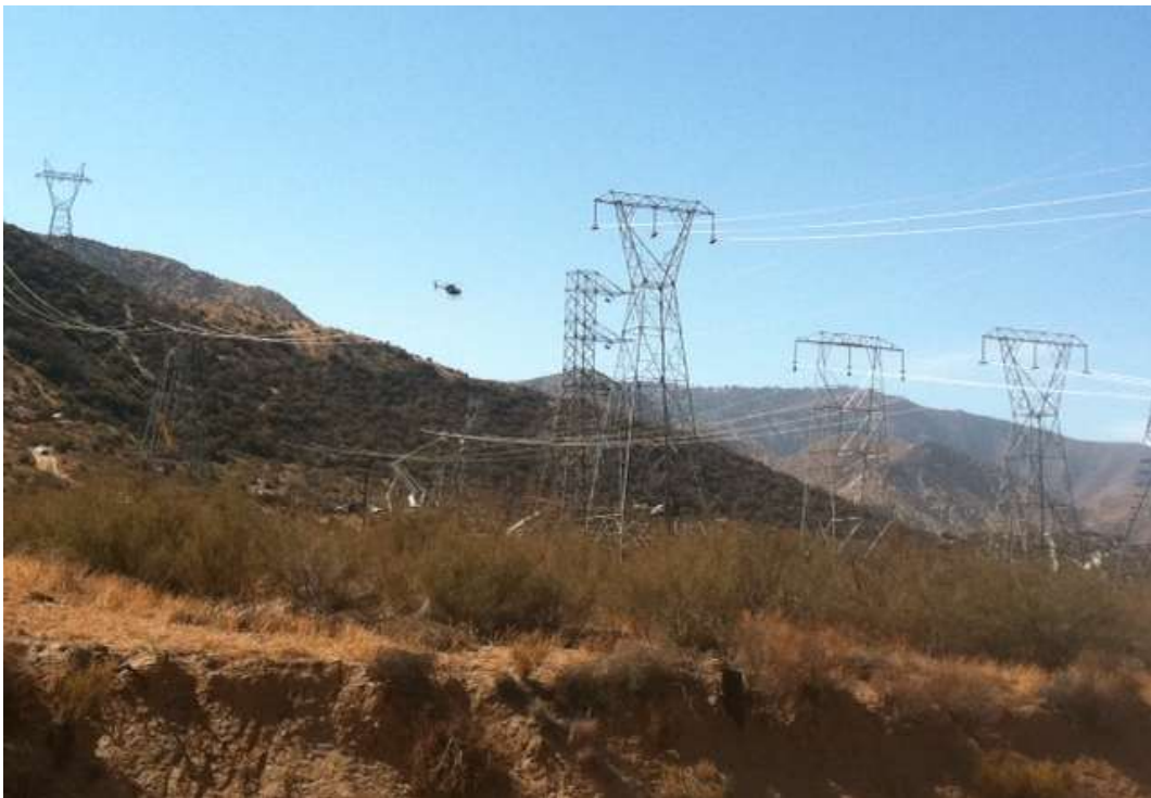
Figure 2: Wire activity at Constructs 16/17, Segment 11C.
