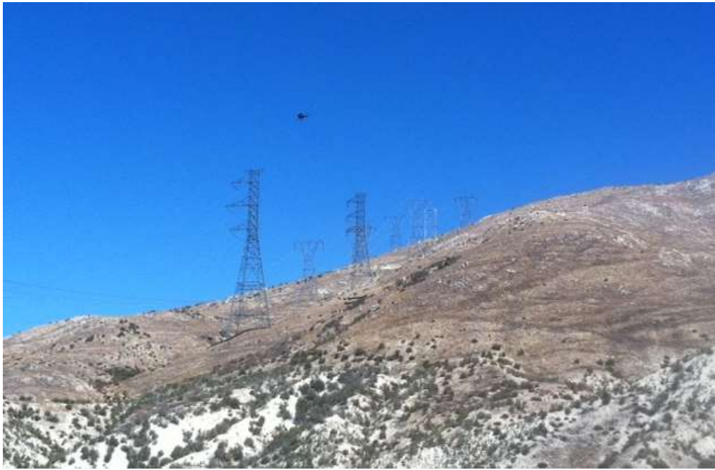
Figure 3: Wire stringing operations on Construct 14, Segment 11C.
