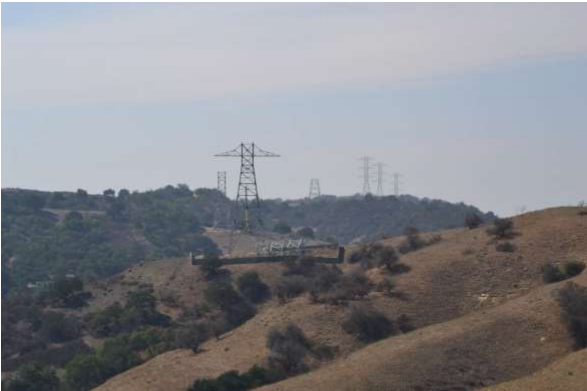
Figure 6: Assembly of towers in Tonner Canyon, Segment 8, Phase 1.
