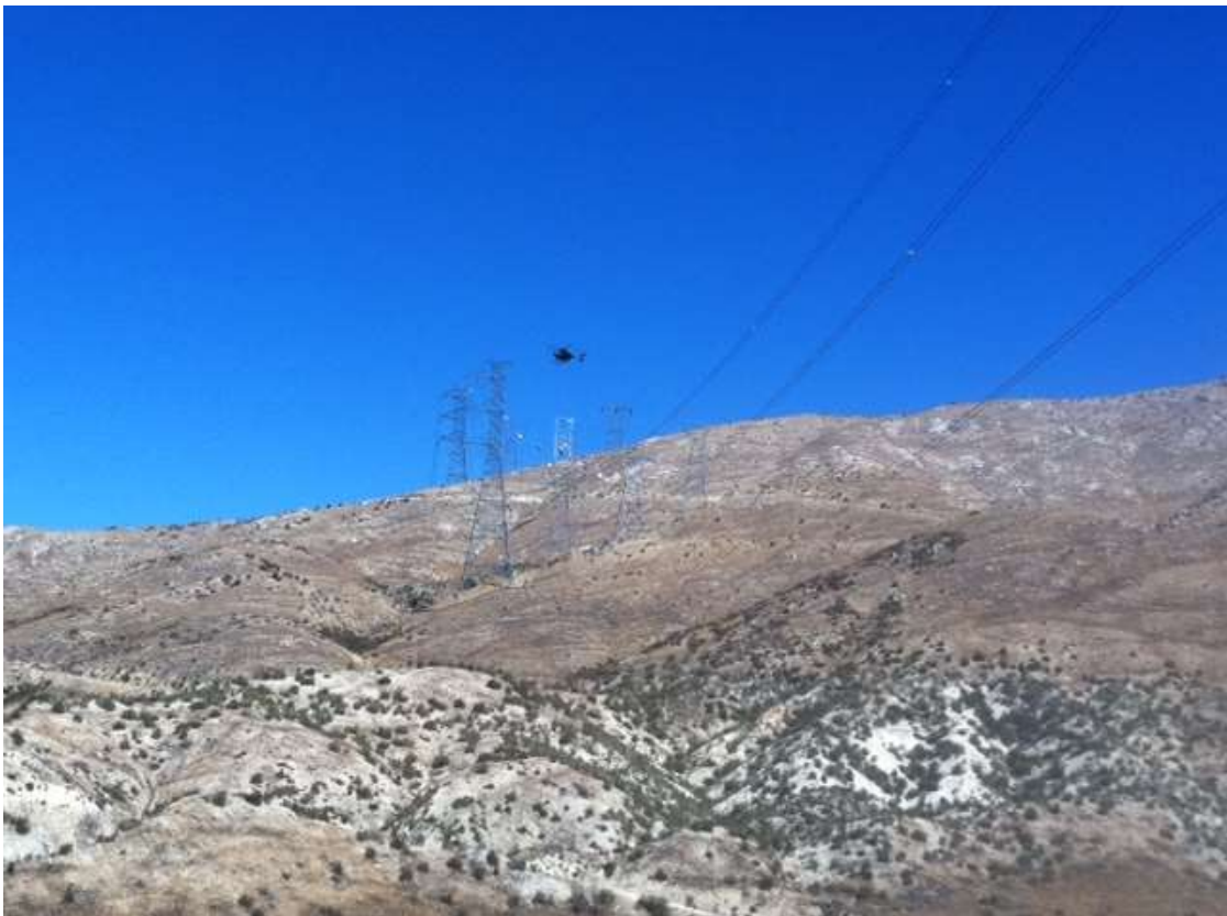
Figure 4: Wire stringing activity between Constructs 14 and 15, Segment 11C.
