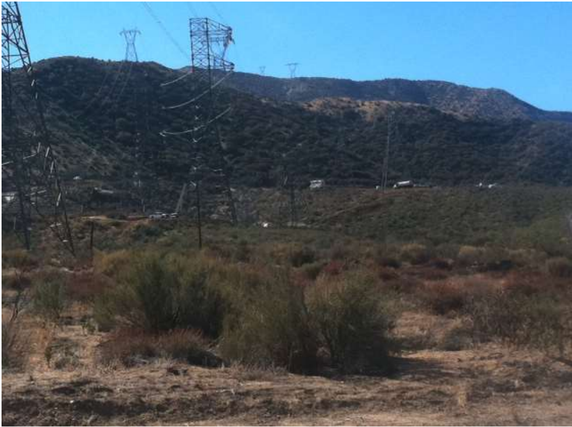
Figure 3: Wire stringing activity at Construct 16, Segment 11C.
