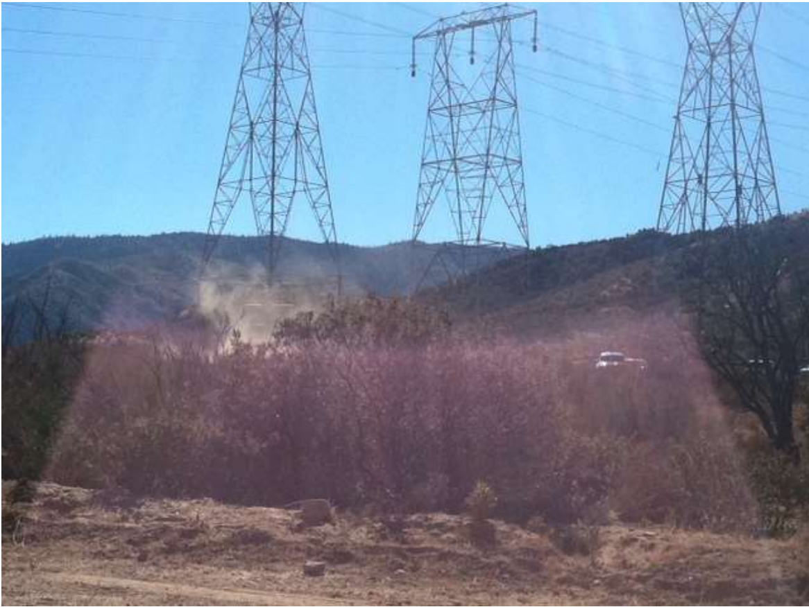
Figure 5: Fugitive dust generation near Construct 15, Segment 11C.
