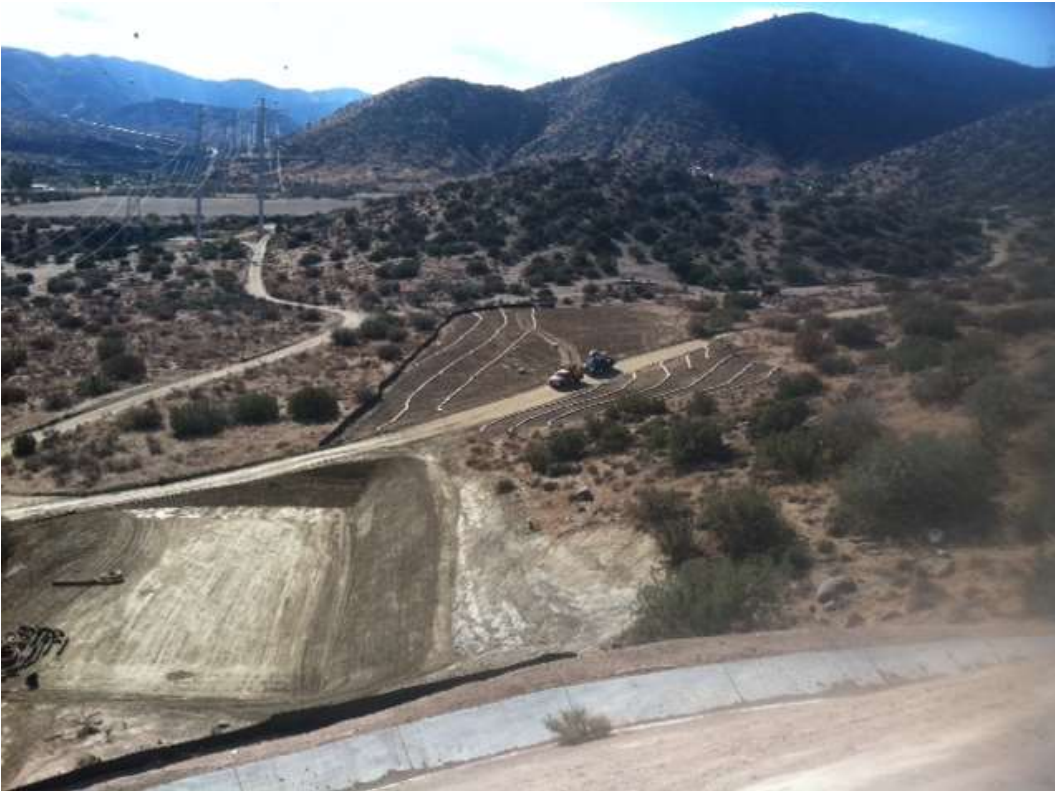
Figure 1: BMP installation activity at Construct 5/6, Segment 6A.
