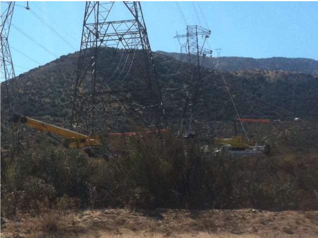
Figure 2: Wire stringing operations on Construct 16, Segment 11C.
