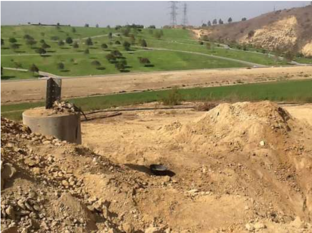
Figure 8: Foundation removal at Tower M7-T2 in Rose Hills, Segment 8, Phase 4.
