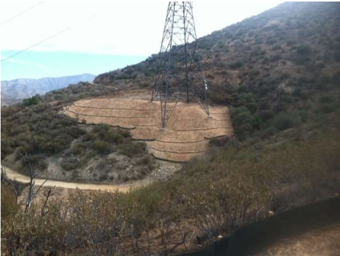
Figure 3: BMP installation at Construct 17, Segment 11C.
