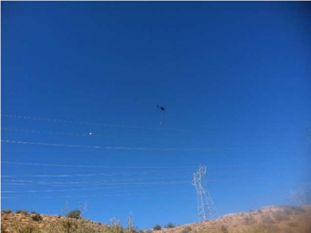
Figure 1: Marker ball installation between Constructs 4 and 5, Segment 11C.
