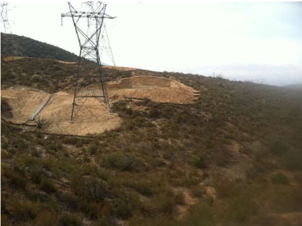
Figure 2: BMP installation at Construct 16, Segment 11C.
