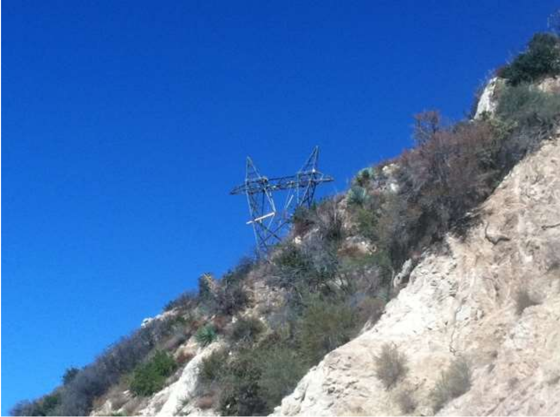
Figure 1: Tower erection activity at Construct 57, Segment 11C.
