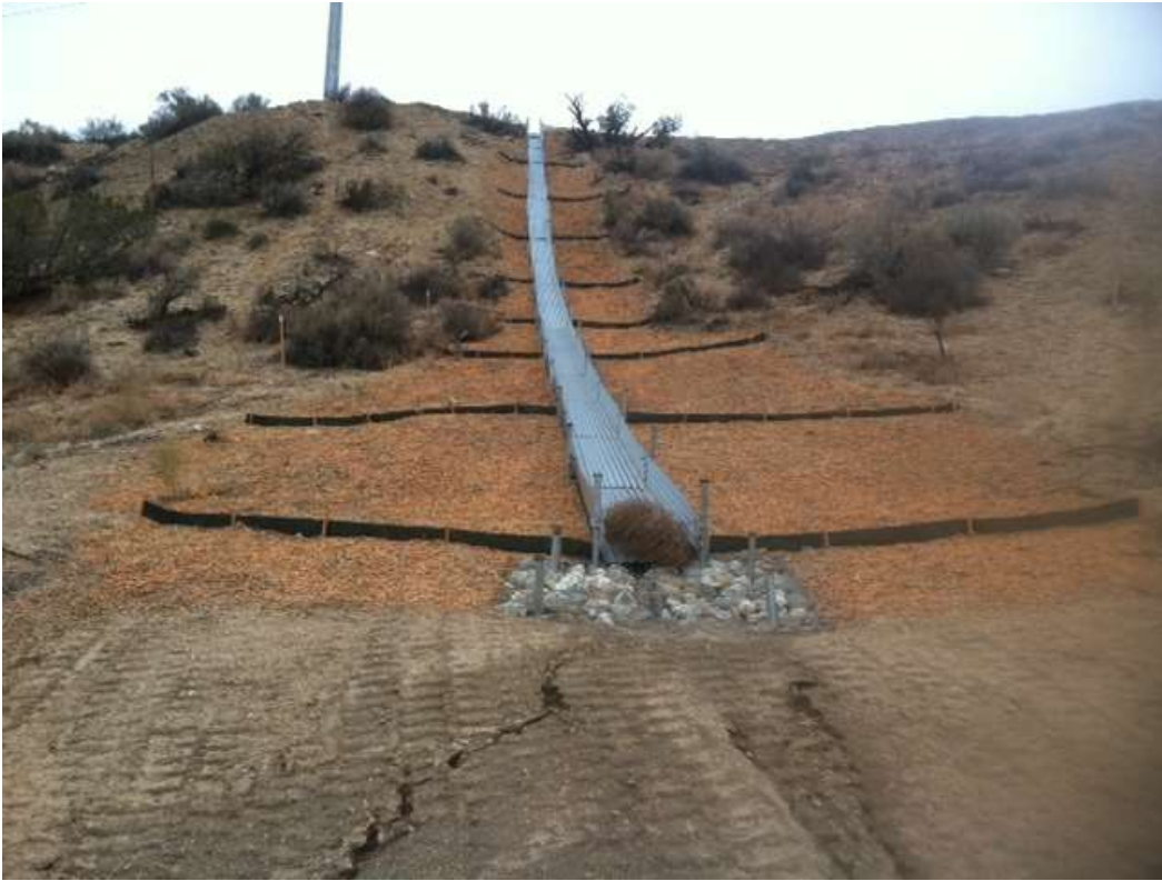
Figure 1: McCarthy Drain 01 on Segment 6A post storm.
