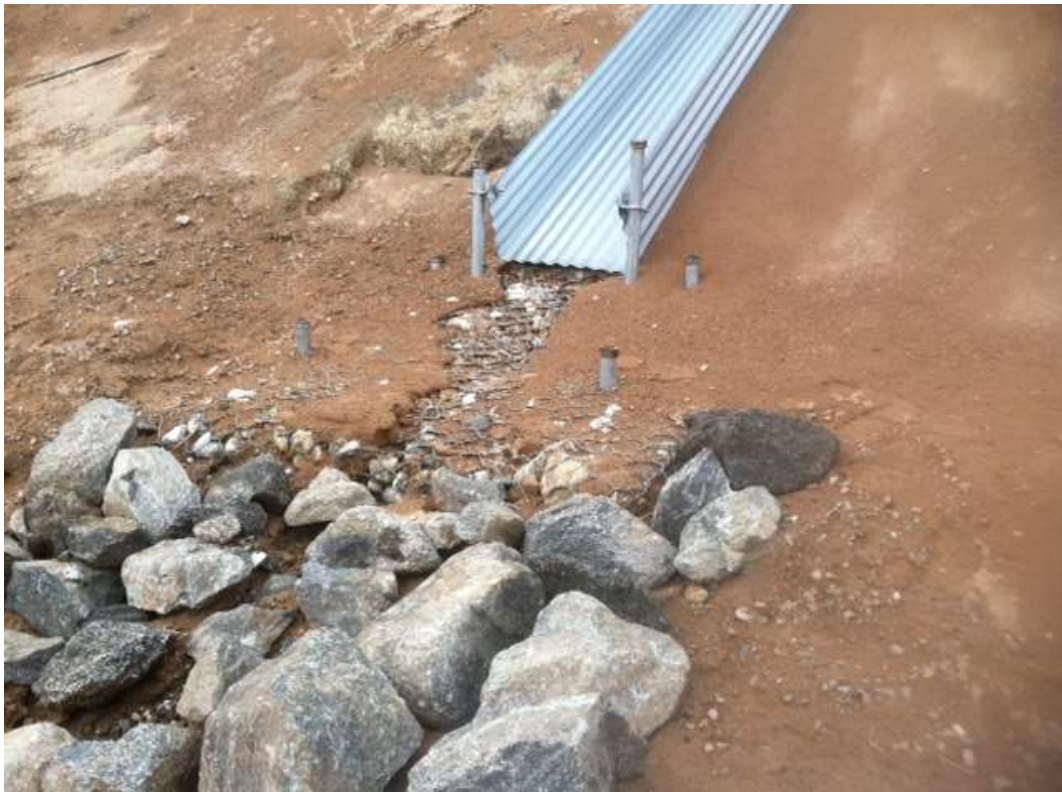
Figure 3: Rock dissipater for drainage of Construct 5 slope, Segment 6A, post-storm.
