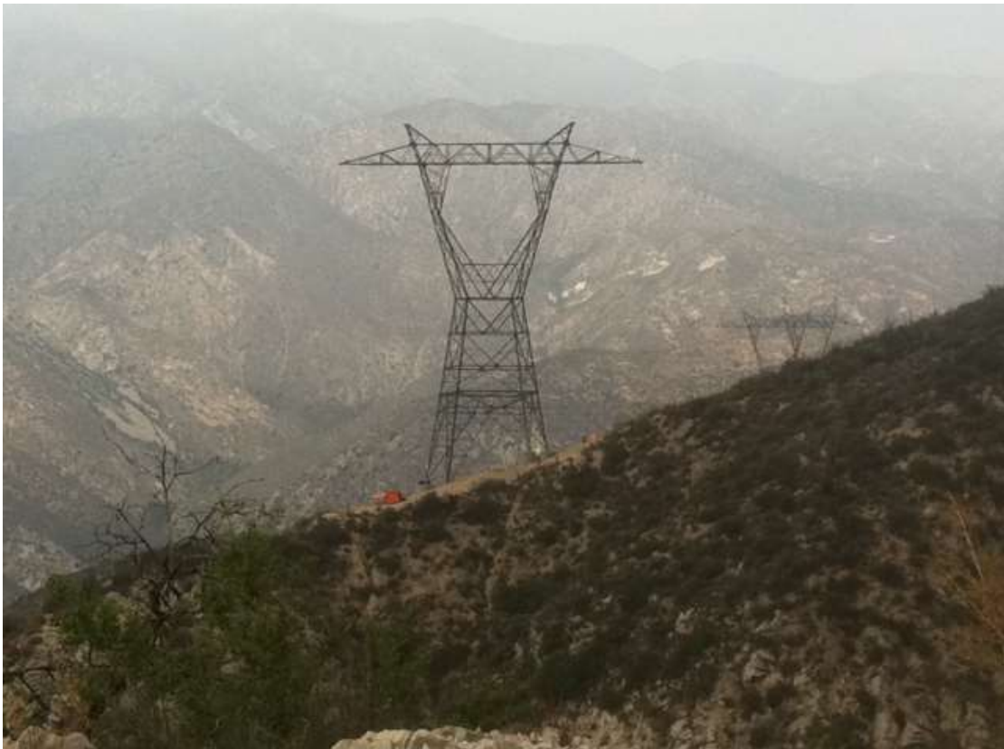
Figure 3: Erection activities at Construct 52, Segment 11C.
