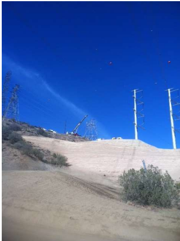
Figure 2: Foundation activities at Construct M17-T3X, Segment 11C.
