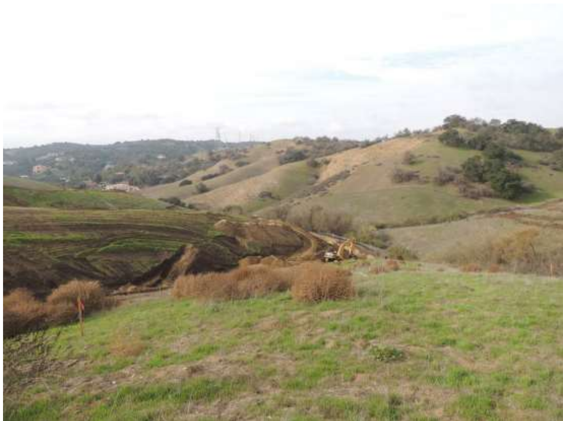
Figure 4: Grading continues at the WTS.
