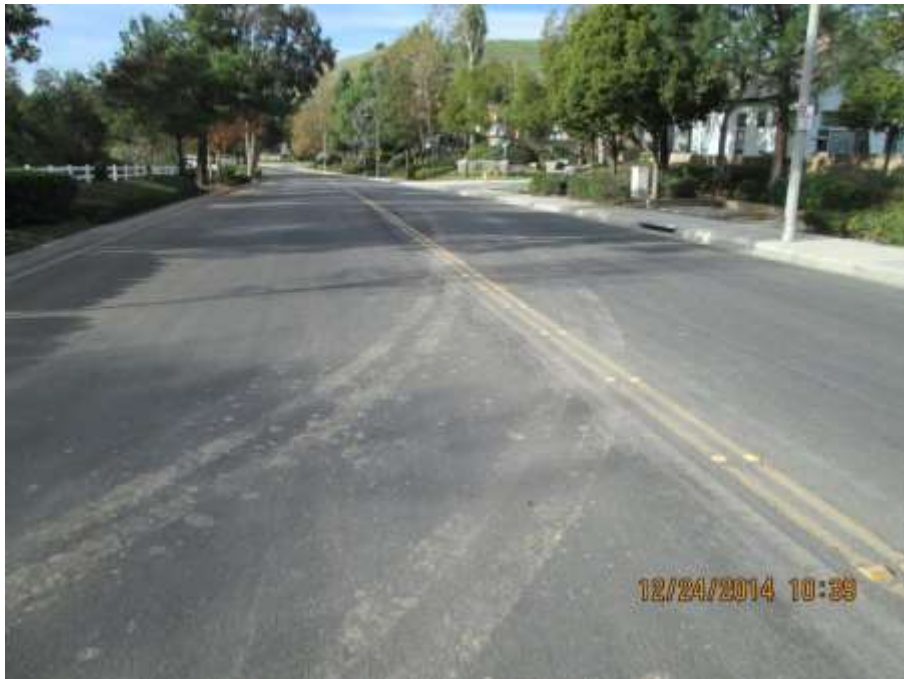
Figure 2: Track out was reported along Eucalyptus Avenue in Chino Hills, Segment 8, 500 kV Underground (photo courtesy of FRED).
