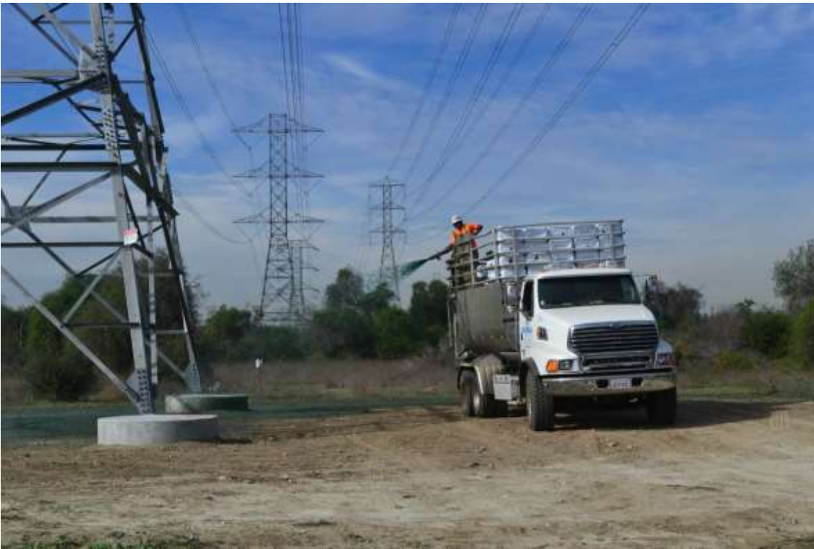
Figure 5: Hydroseeding of disturbed areas in Whittier Narrows, Segment 8, Phase 4.
