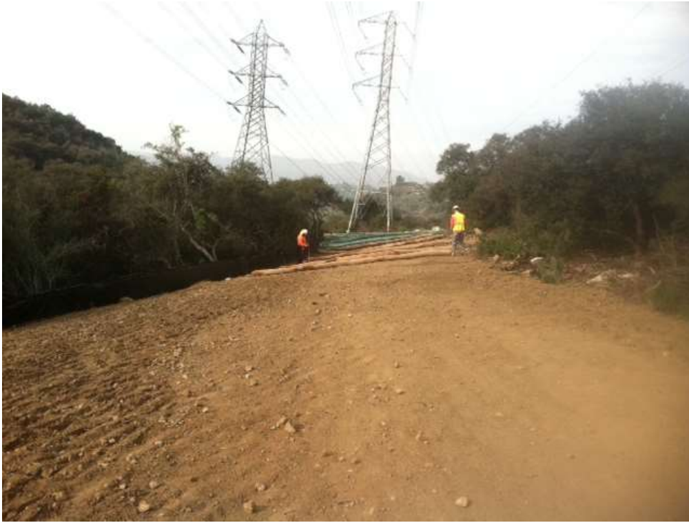
Figure 1: BMP installation at restored Chaney Trails WSS, Segment 11B.
