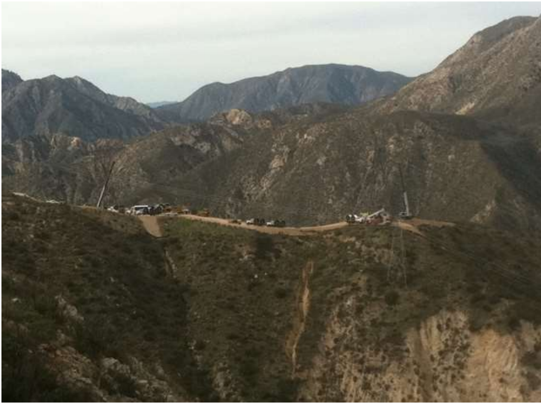
Figure 3: Wire stringing operations at WSS 53/54, Segment 11C.
