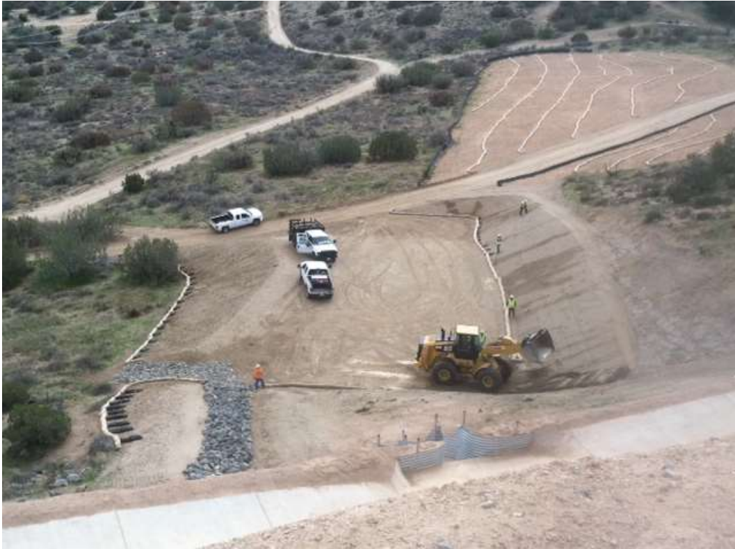
Figure 1: BMP installation activities at Construct 5, Segment 6A.
