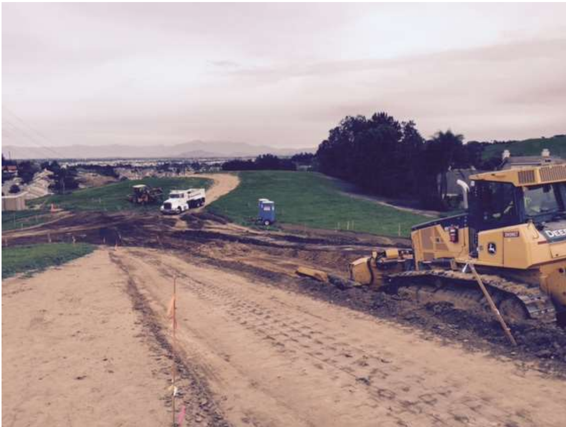
Figure 4: Grading and access road preparation near VC #8, 500 kV Underground.
