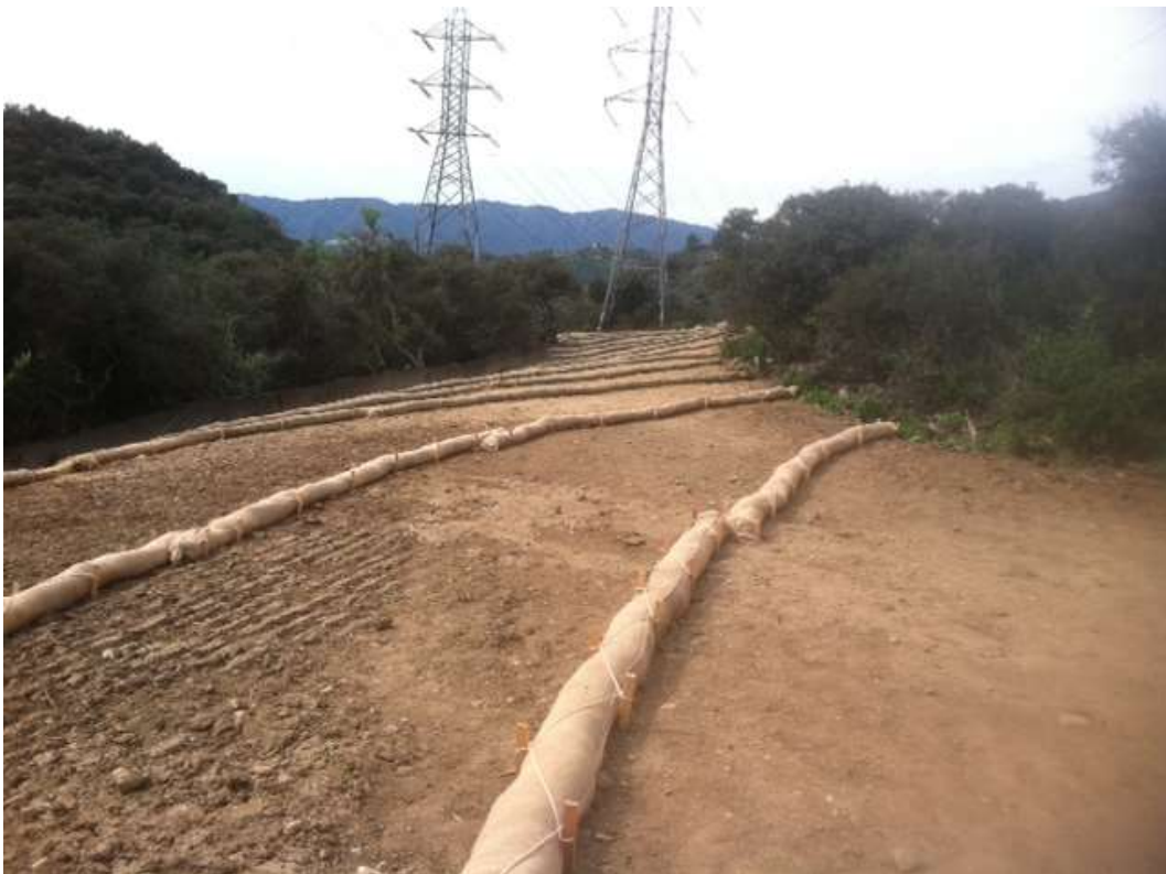
Figure 2: BMP installation at restored Chaney Trails WSS, Segment 11B.
