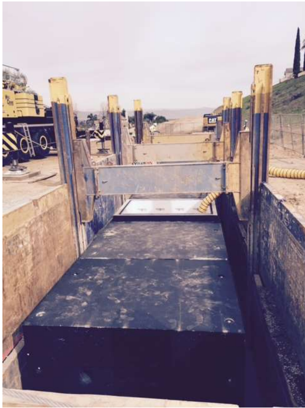
Figure 5: Splice vault installation at VC #5, 500 kV Underground.
