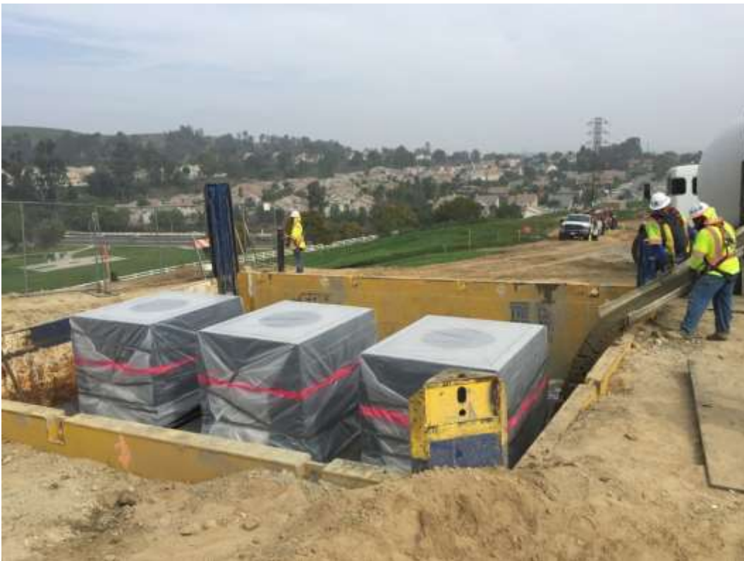
Figure 6: Vault placement occurred on the 500 kV Underground.
