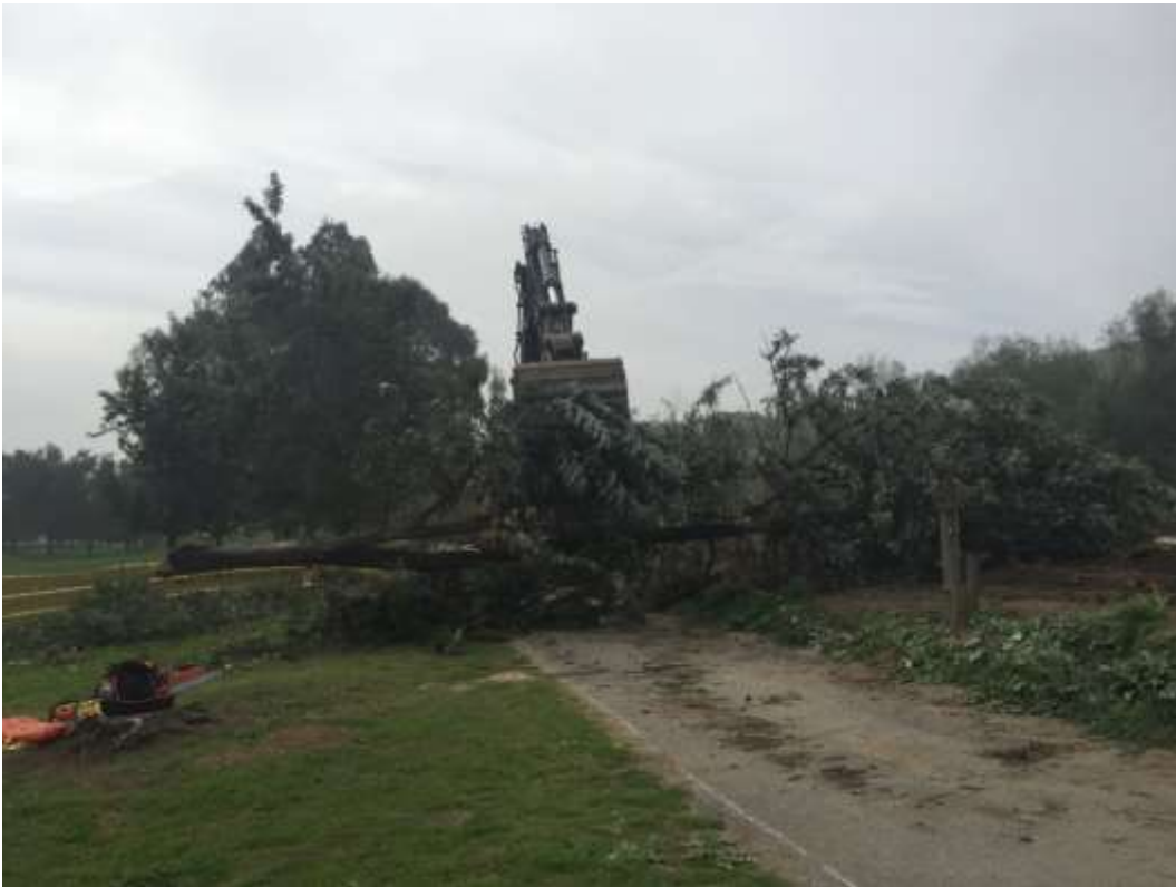
Figure 3: Vegetation removal along the right-of-way between RV #2 and RV #4, 500 kV Underground.
