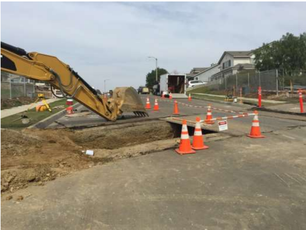
Figure 4: Trenching activities occurred between VC #12 and VC #13, 500 kV Underground.
