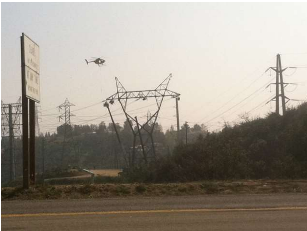
Figure 2: Wire stringing operations at Construct 67, Segment 11C.
