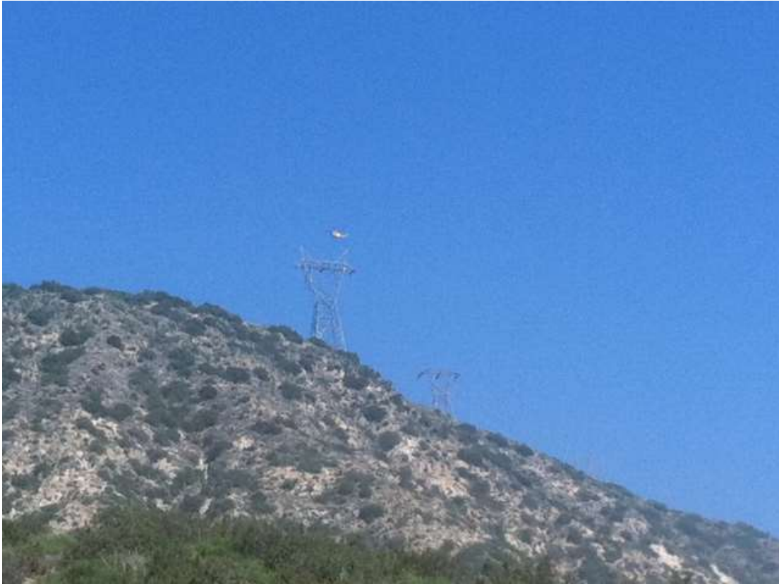
Figure 1: Wire stringing activities at Construct 66, Segment 11C.
