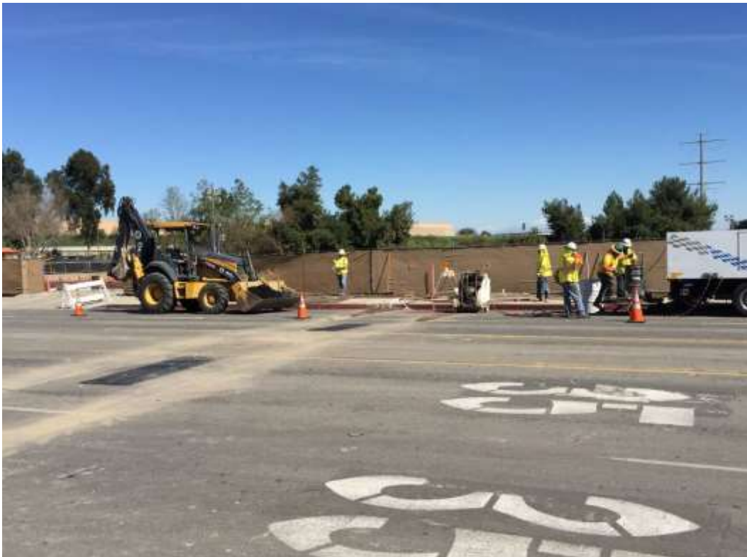
Figure 6: Asphalt cutting along Pipeline Avenue, 500 kV Underground.
