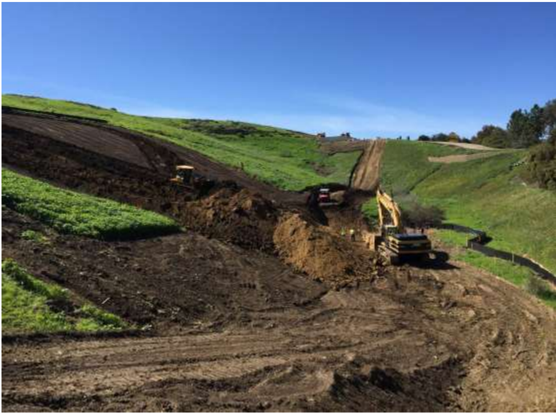
Figure 7: Slope grading and excavation at RV #1, 500 kV Underground.
