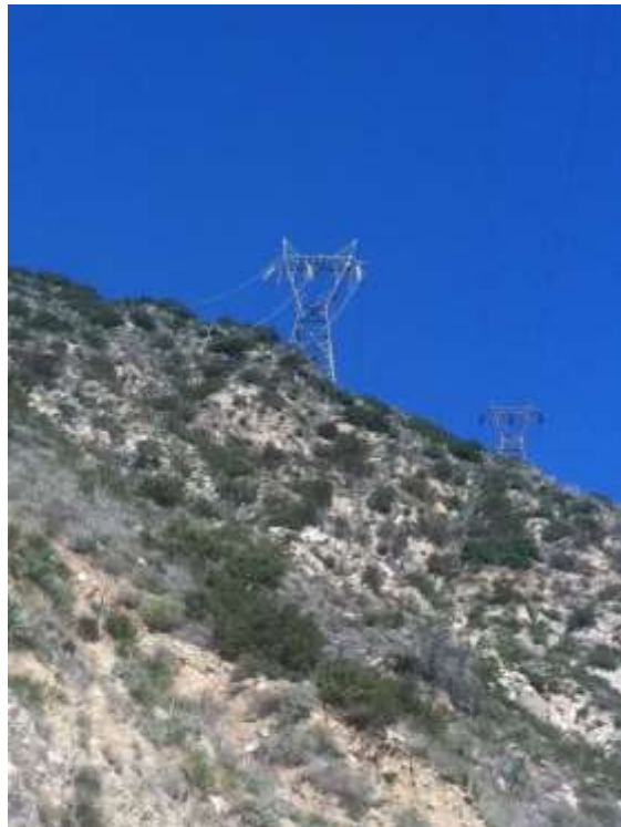
Figure 2: Wire stringing operations at Construct 66, Segment 11C.
