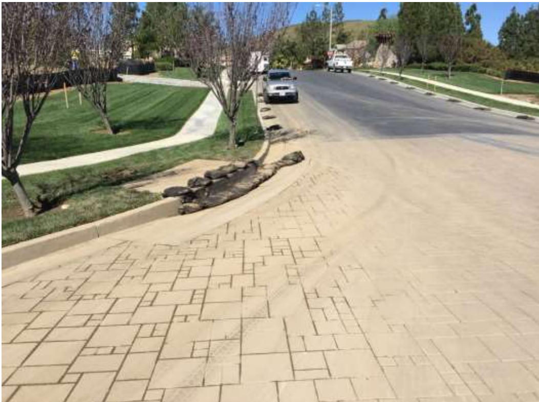
Figure 4: Results of post-storm clean-up along Canon Lane, 500 kV Underground.
