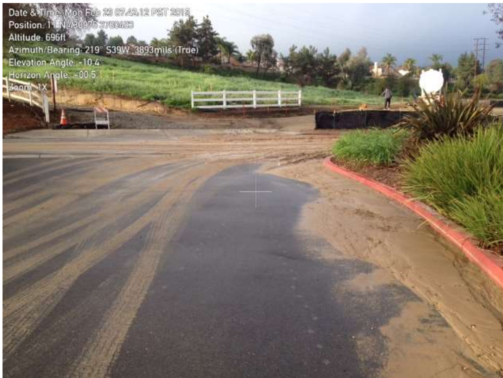
Figure 10: Offsite discharge at Veterans Park in Chino Hills after recent rain event, 500 kV Underground.
