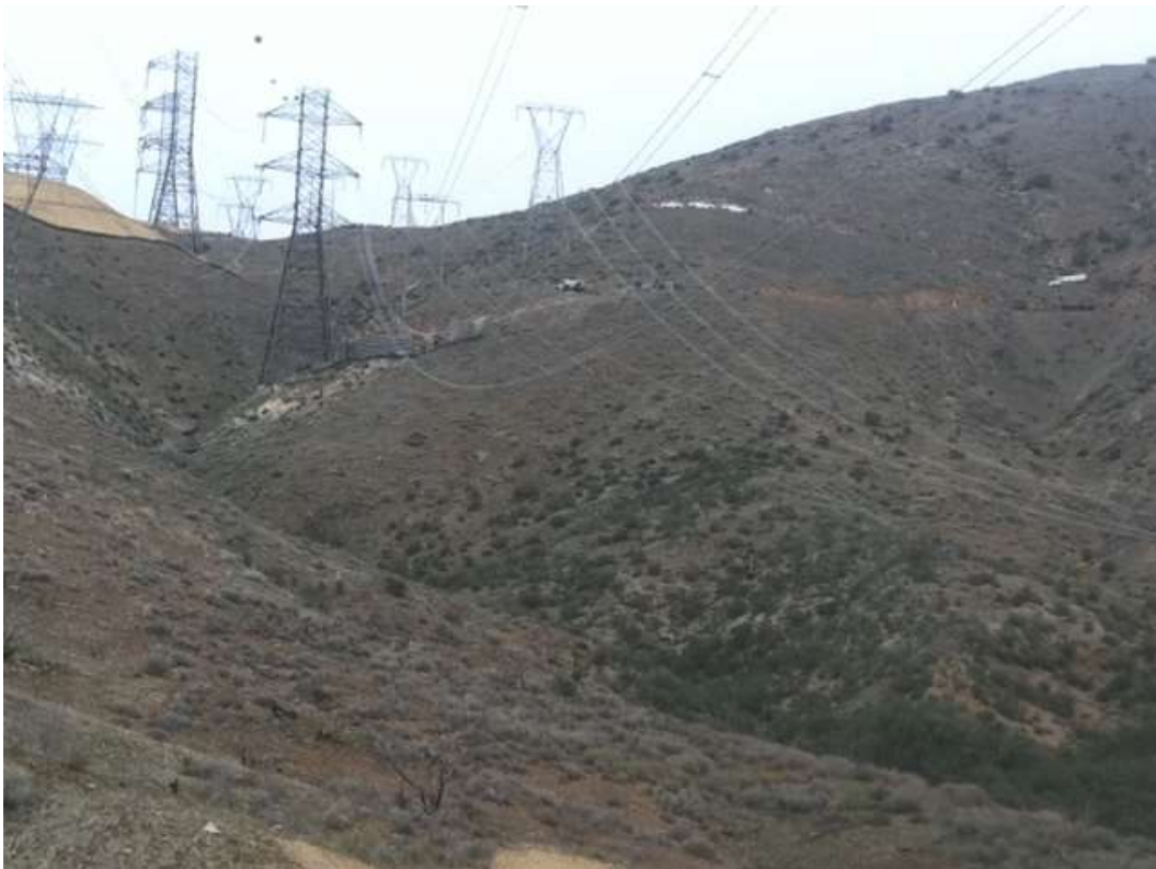
Figure 2: Tower pad grading at Construct 9, Segment 11C.
