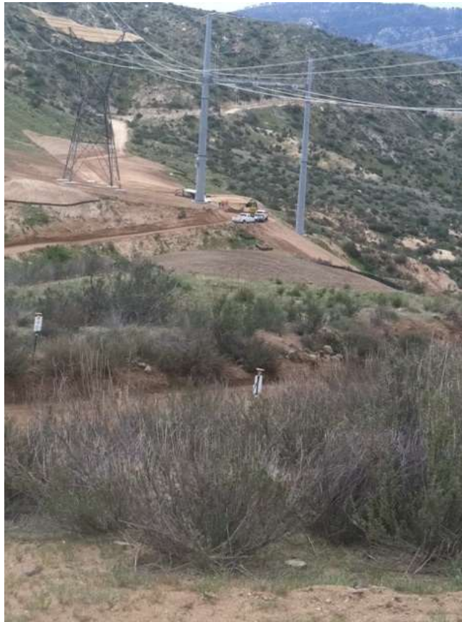
Figure 3: Tower pad grading at Construct 11AX, Segment 11C.
