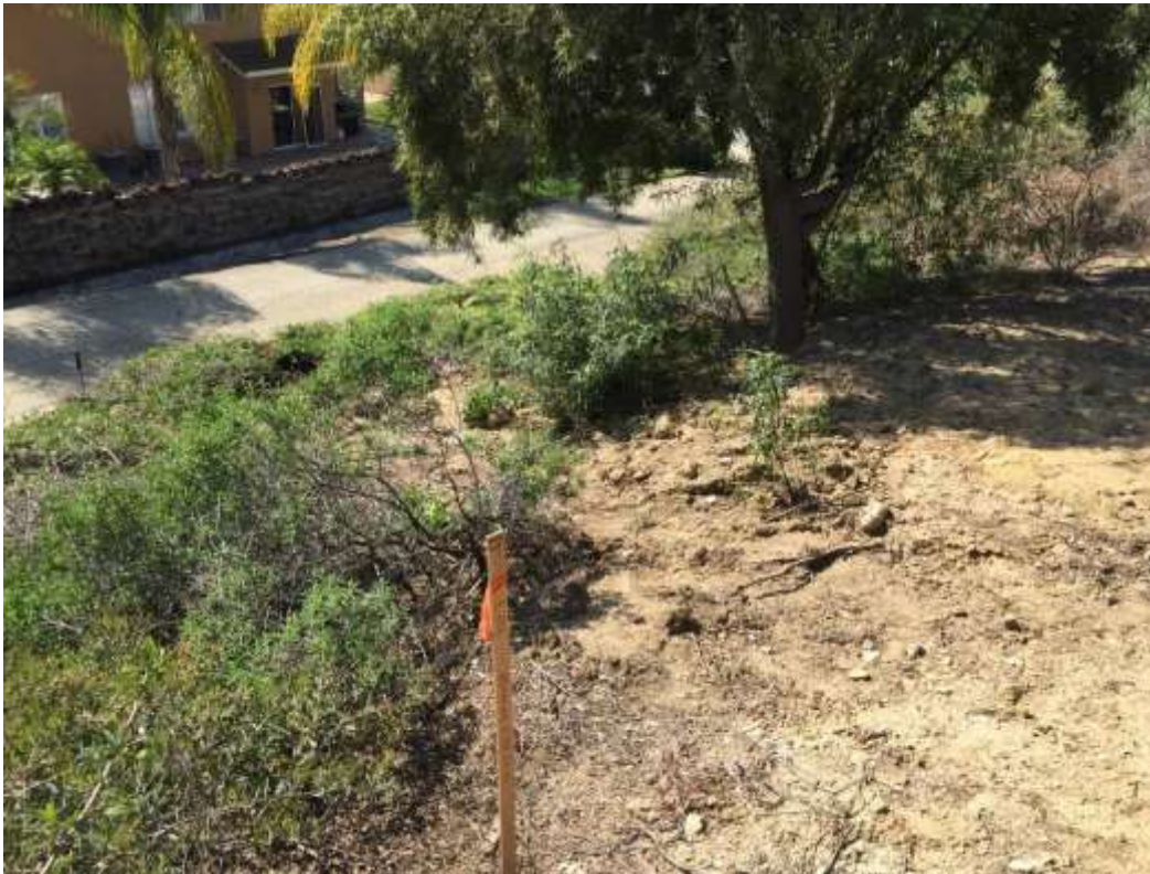
Figure 7: Offsite discharge near VC #9. Note staking indicating approved limits of disturbance (photo courtesy of SCE).
