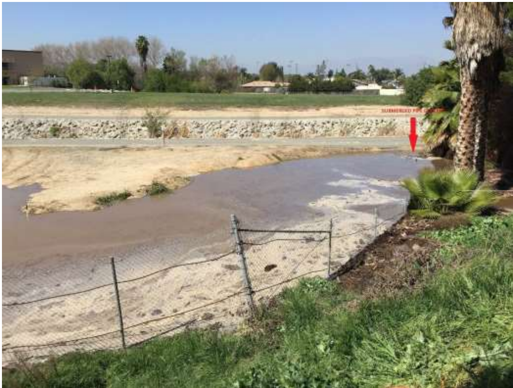
Figure 6: Water and sediment flowing into the Carbon Canyon Creek Channel as a result of the water line rupture (photo courtesy of SCE).
