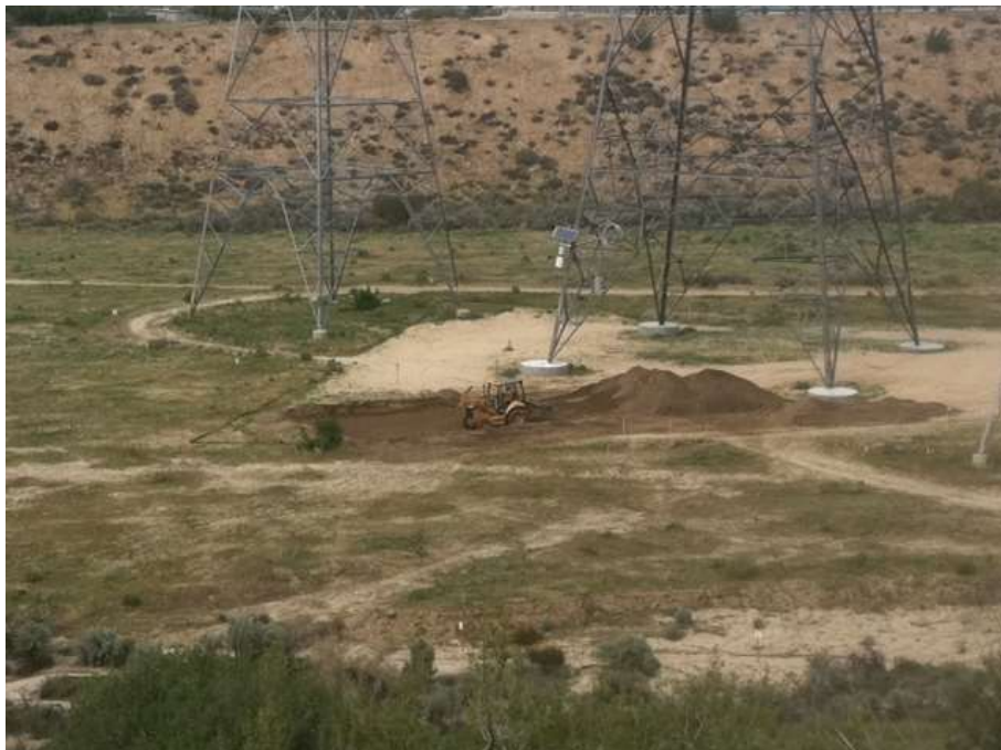
Figure 2: Tower pad grading at Construct 1, Segment 11C.
