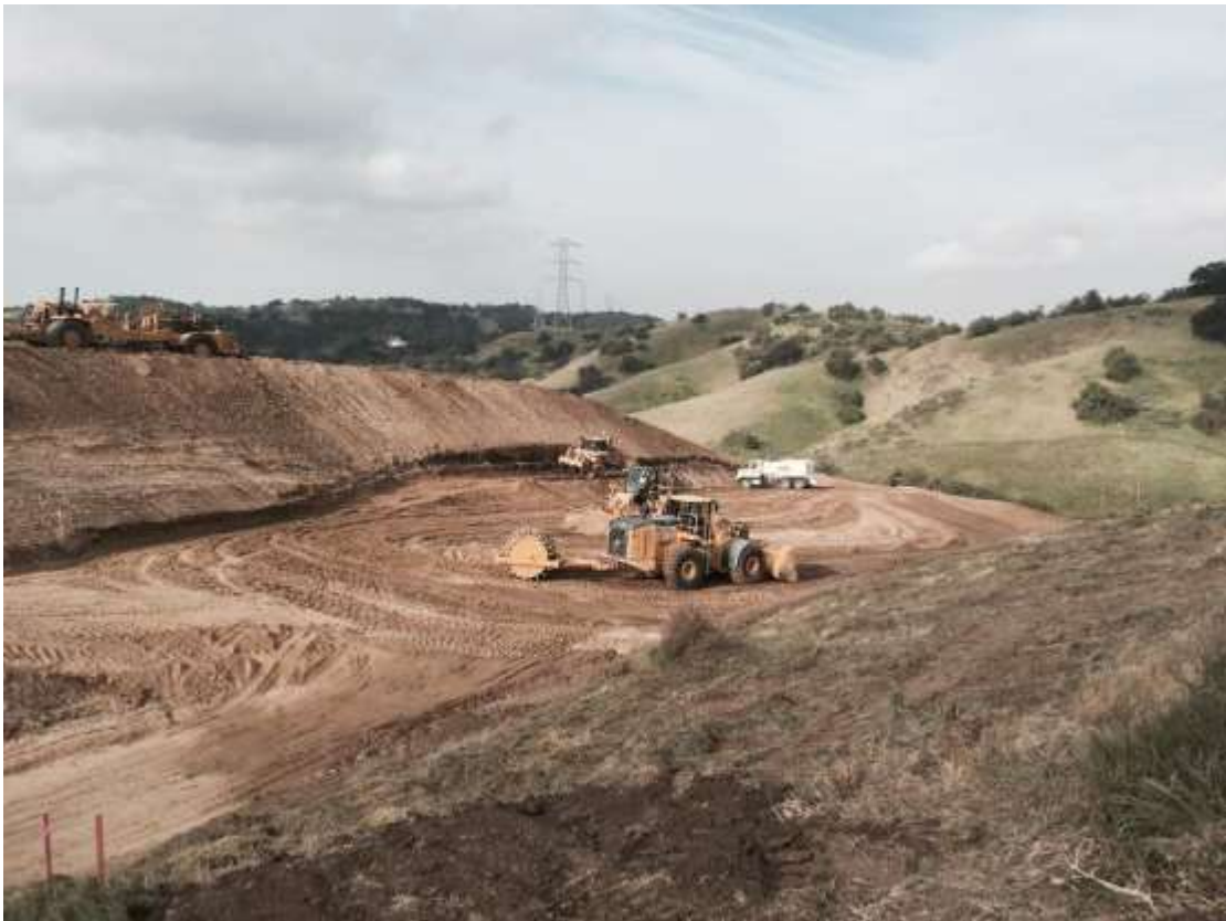
Figure 6: Grading activities occurring at the WTS, 500 kV Underground.
