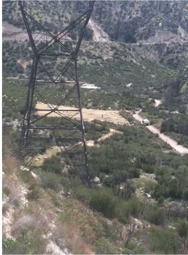
Figure 1: Container planting at Pull Site 28/29, Segment 6.
