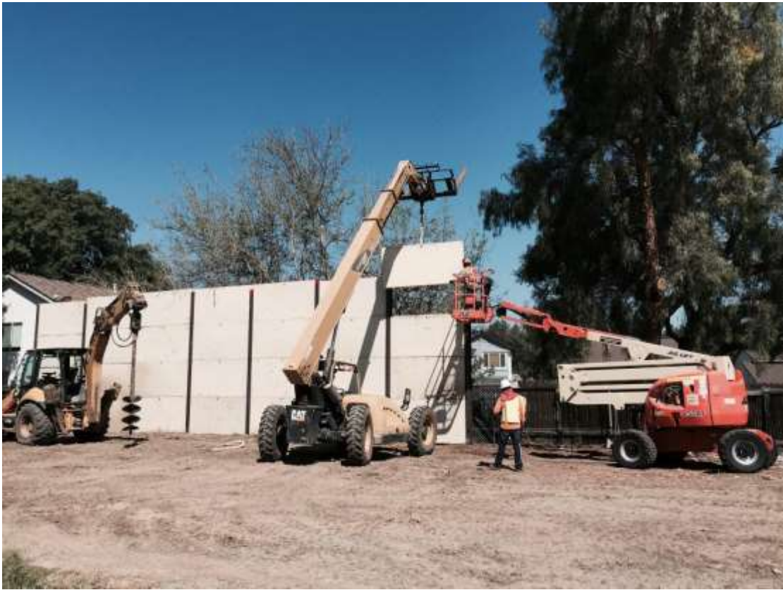
Figure 5: Sound wall installation at the alternate HDD site.
