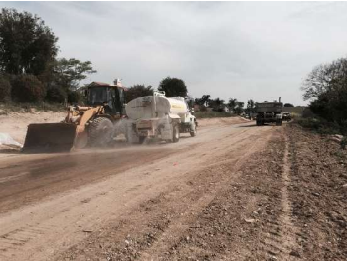
Figure 4: Truck watering for dust abatement along the 500 kV Underground right-of-way.
