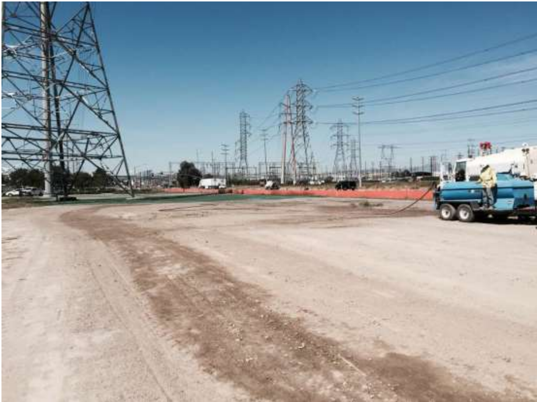
Figure 3: Hydroseeding occurring at Tower M66-T8 (Segment 8, Phase 3).
