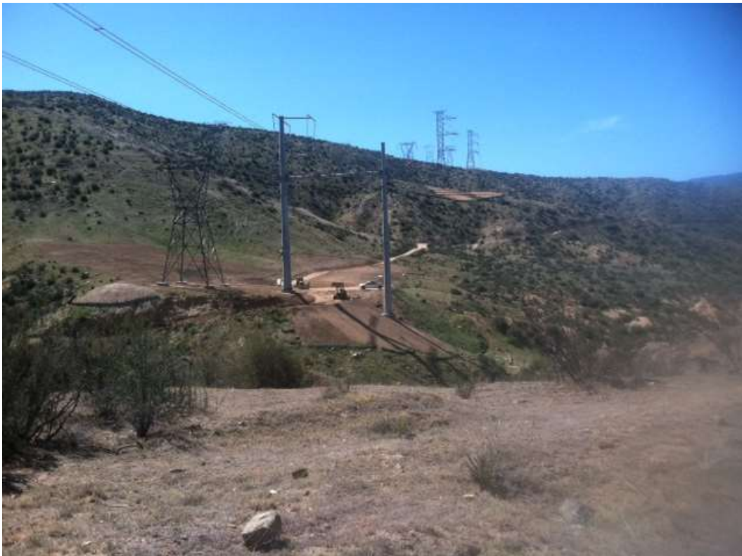
Figure 2: Tower pad and road grading at Construct 11AX, Segment 11C.
