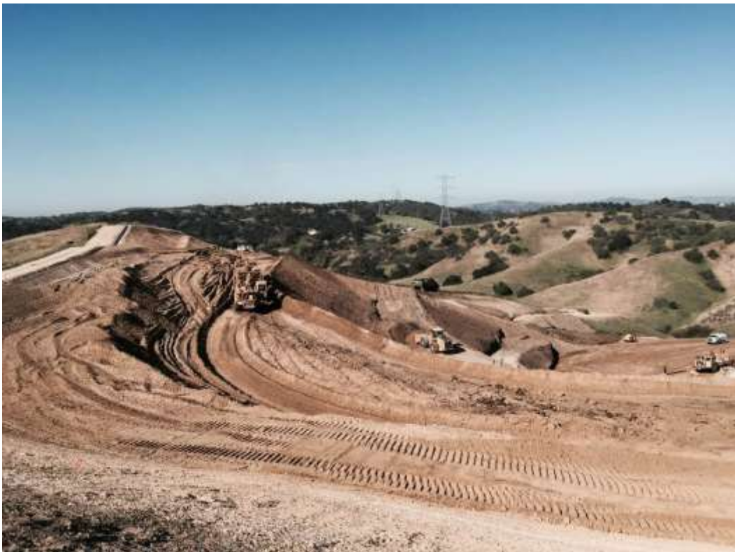
Figure 6: Heavy grading operations occurring at the WTS, 500 kV Underground.
