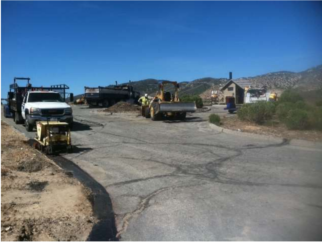
Figure 1: Paving activities at Mill Creek parking area, Segment 6.
