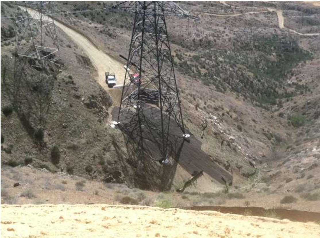
Figure 4: MacMat permanent erosion control blankets (BMP) installation at Construct 9, Segment 11C.
