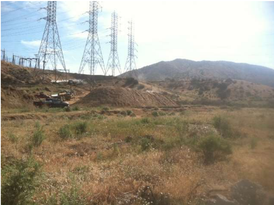
Figure 2: Tower pad grading at Construct -01, Segment 11C.
