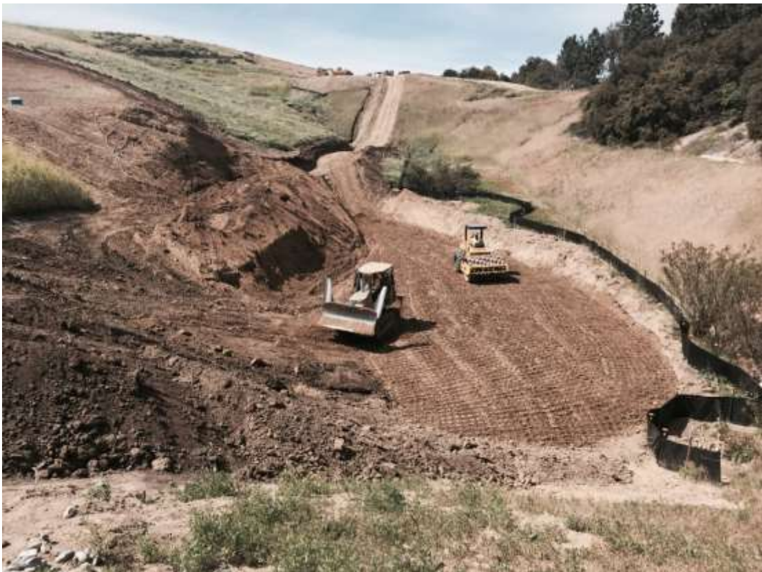
Figure 6: Slope excavation at RV#1, 500 kV Underground.
