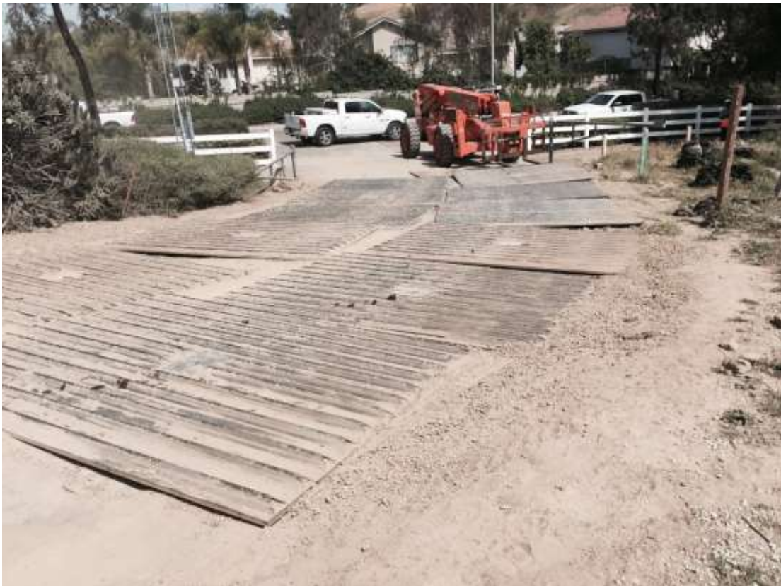
Figure 8: Shaker plate (BMP) installation at the entrance to WTS, 500 kV Underground.
