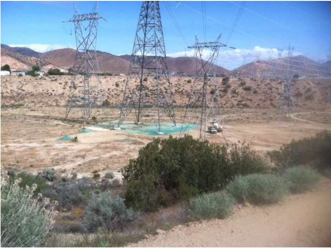
Figure 3: Hydromulching (BMP) installation at Construct 1, Segment 11C.
