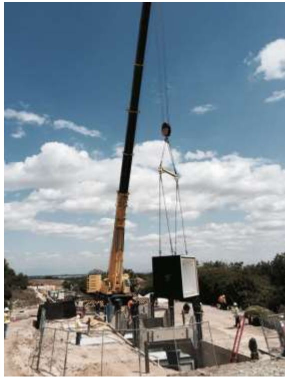
Figure 3: Installing a splice vault at VC #10.
