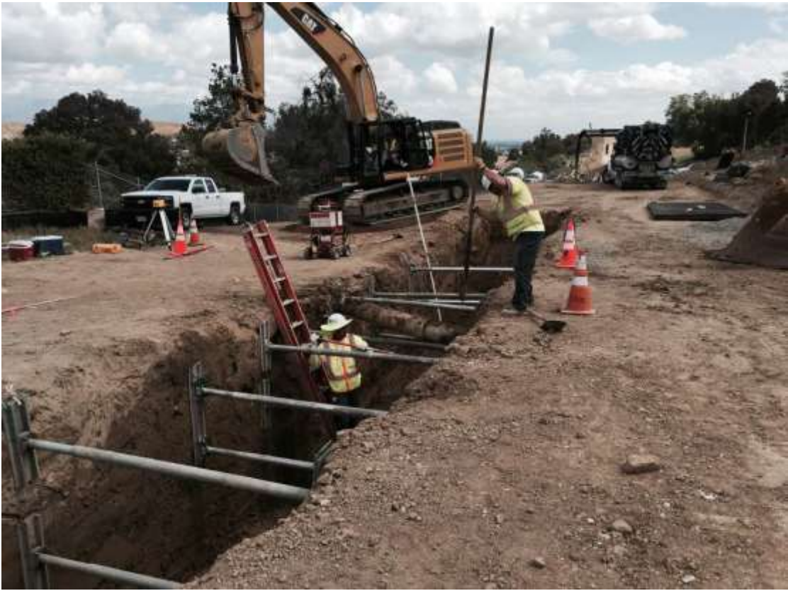
Figure 9: Transite pipe unearthed during trenching work between VC #6 and VC #7.
