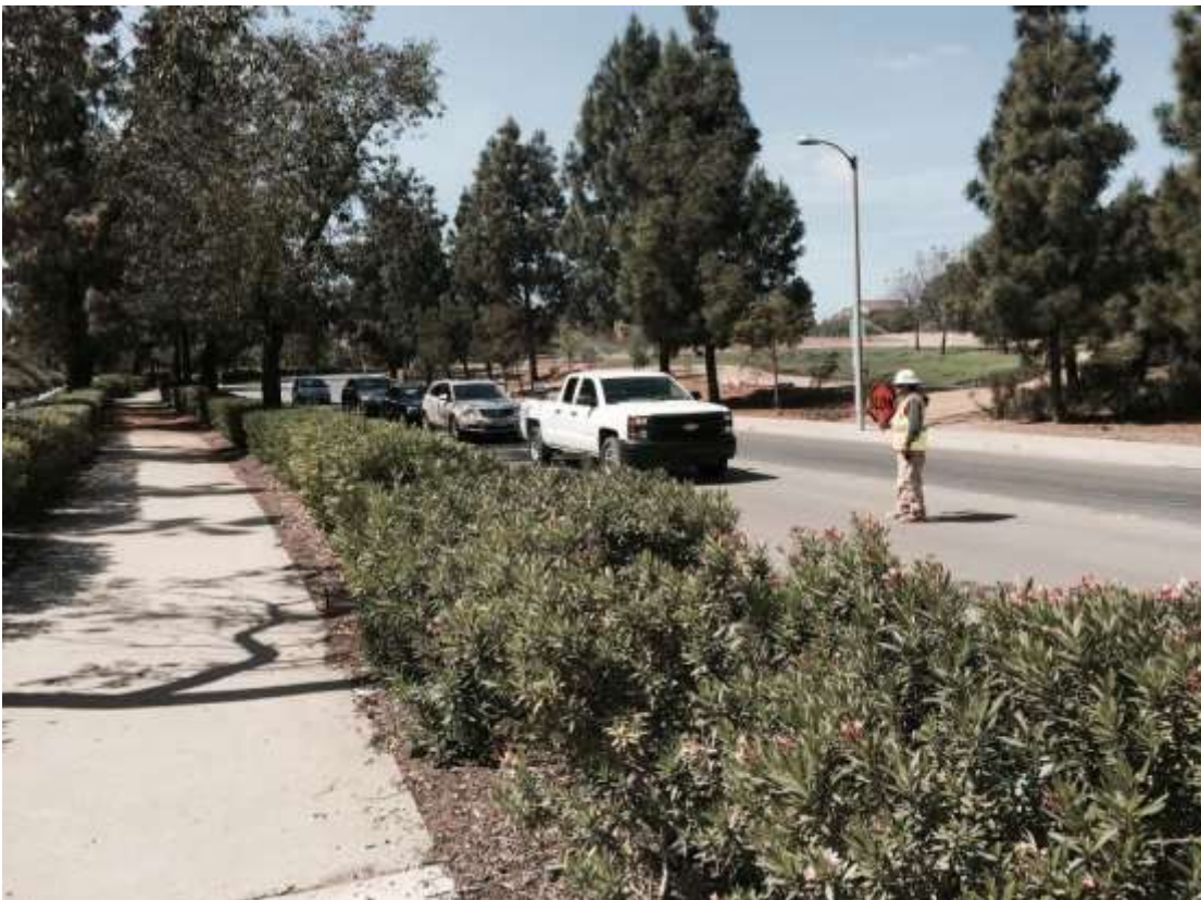
Figure 8: Traffic control station set up within nest buffer along Eucalyptus Avenue.
