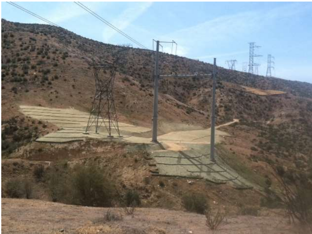
Figure 2: Hydromulch (BMP) installation for final stabilization at Construct 11AXXX, Segment 11C.
