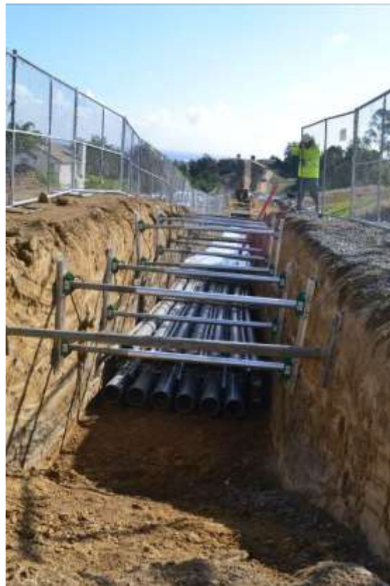
Figure 4: Trenching operations, conduit installation, and concrete encasement between VC #5 and #6.
