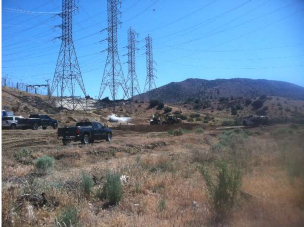
Figure 1: Installation of SoilCement during roadway grading activities at Construct -01, Segment 11C.
