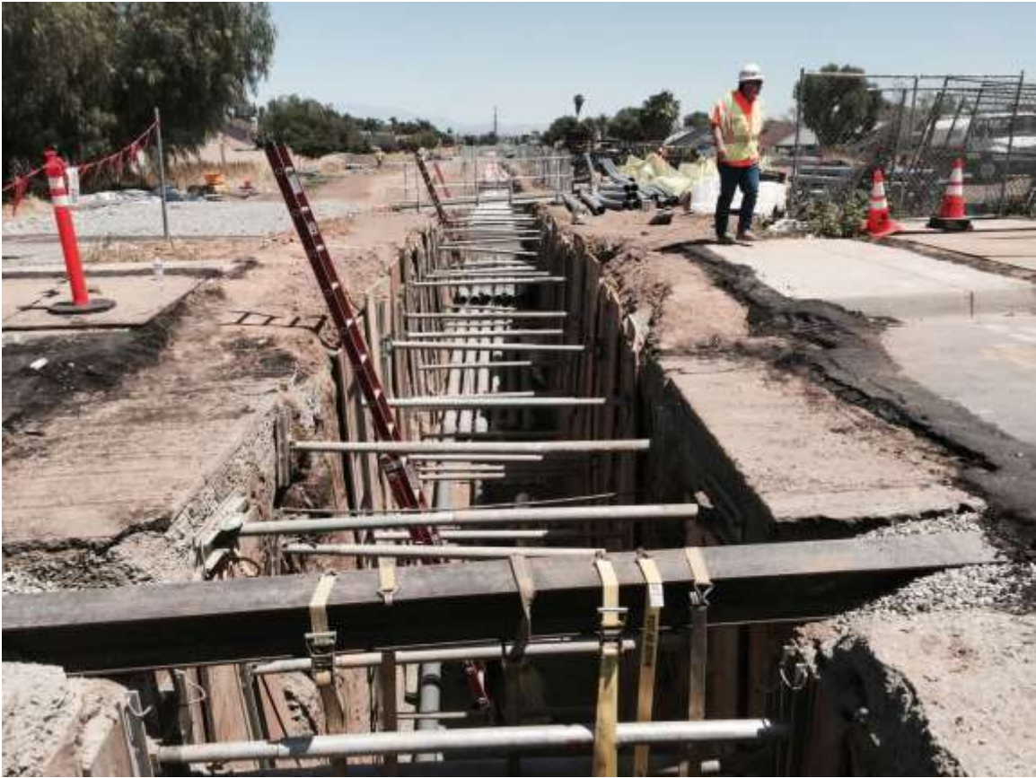
Figure 5: Trenching work between Vault Clusters #12 and #13, 500 kV Underground.
