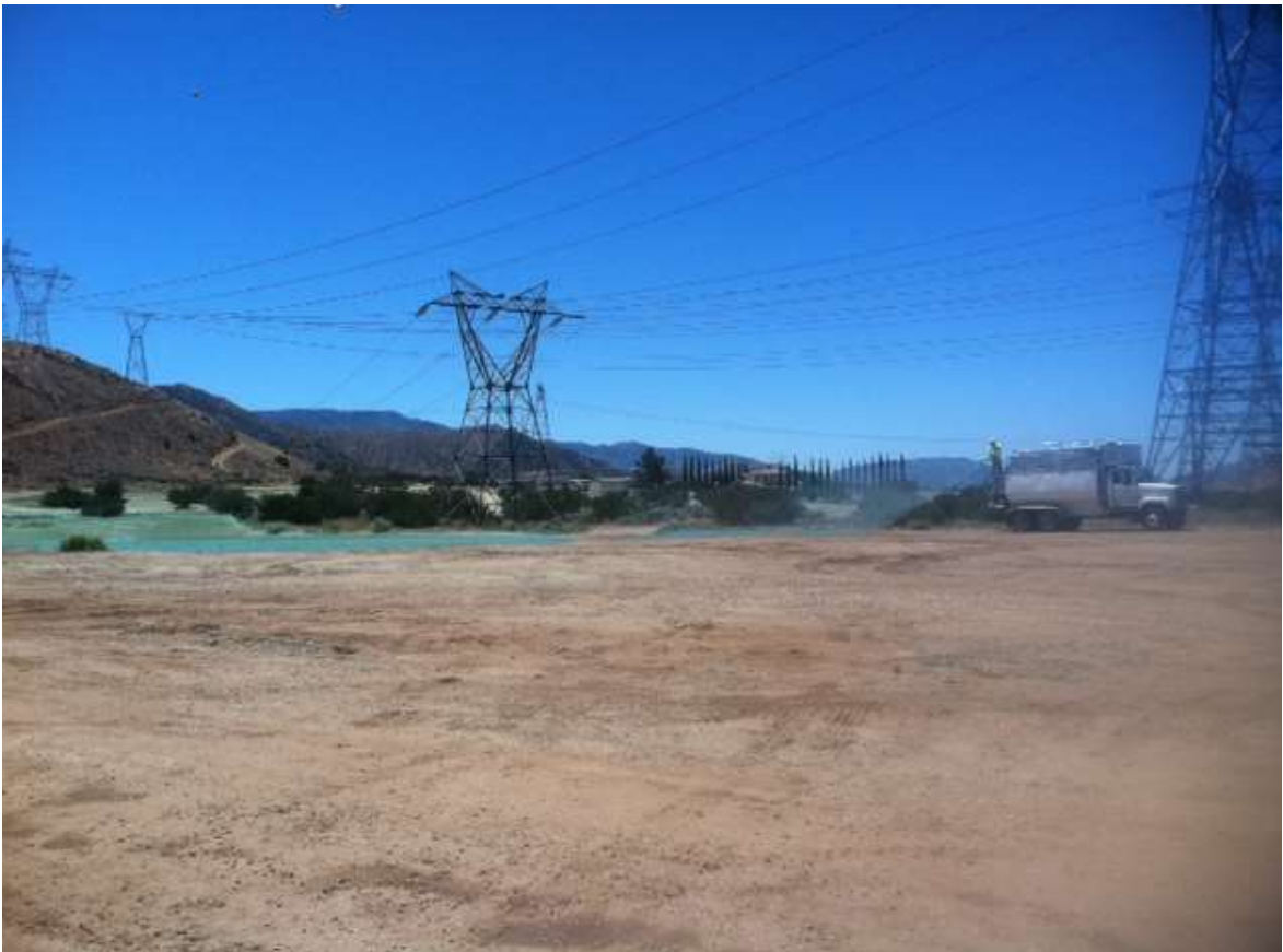
.Figure 3: Hydromulch (BMP) application at Vincent South Yard for final stabilization.
