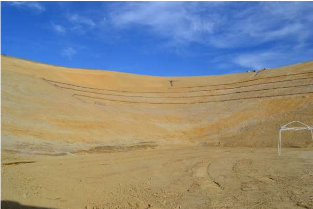
Figure 7: Straw wattles were installed mid slope at the WTS, 500 kV Underground.
