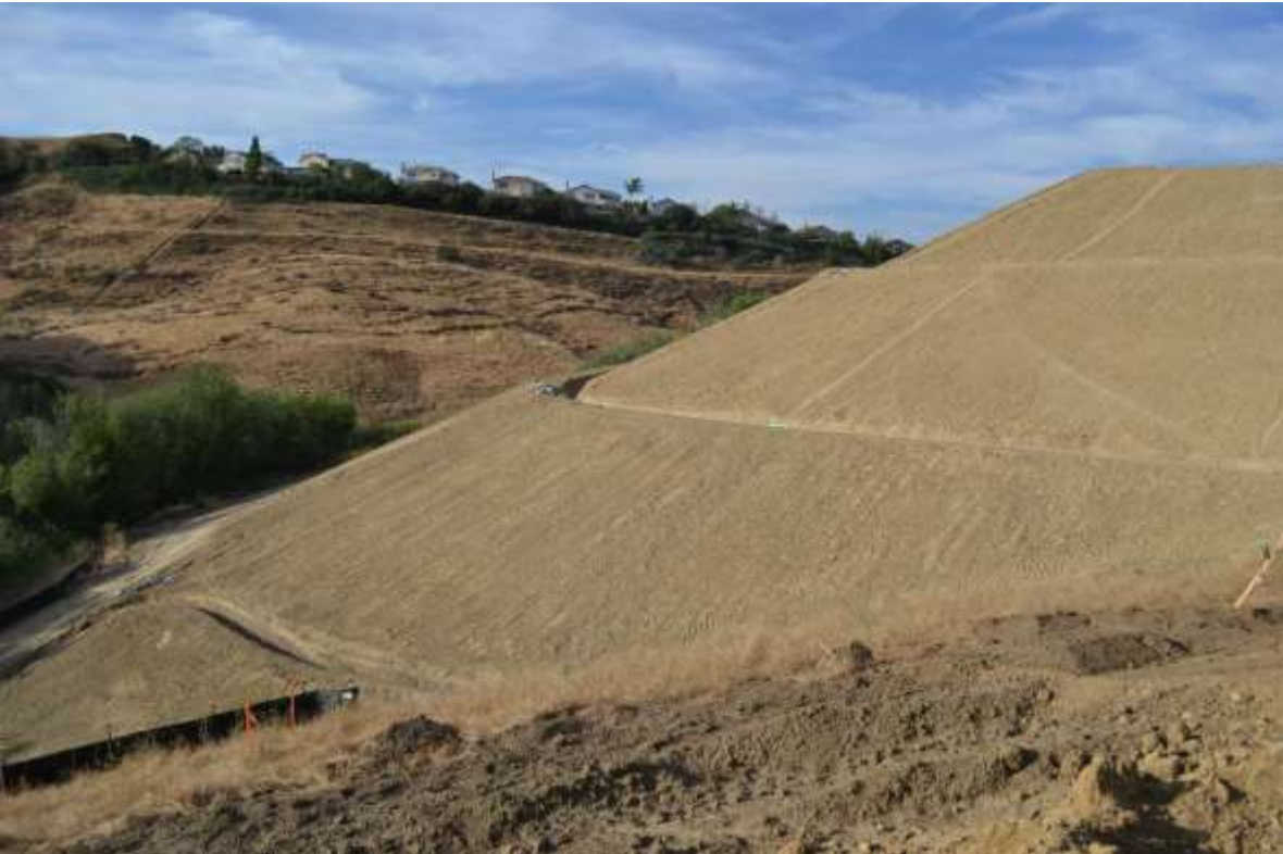
Figure 6: V-ditch construction for drainage at the WTS, 500 kV Underground.
