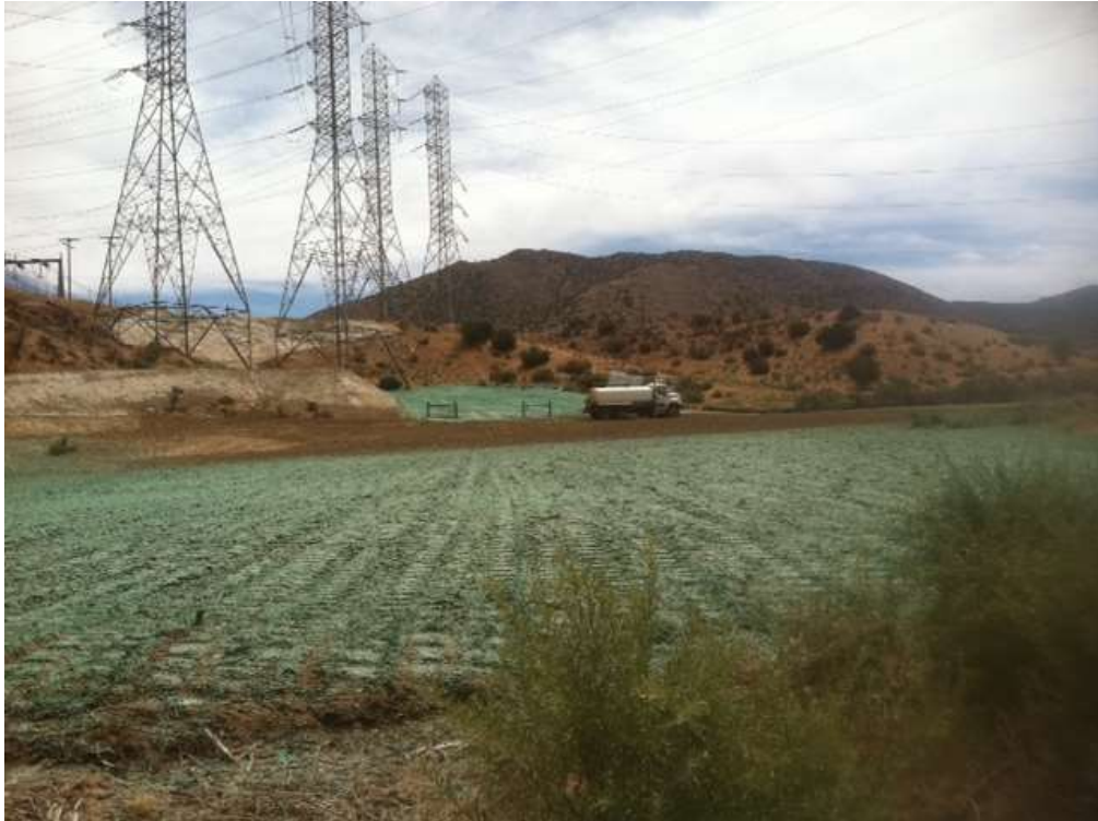
Figure 1: Hydromulching (BMP) for final stabilization at Construct -01, Segment 11C.
