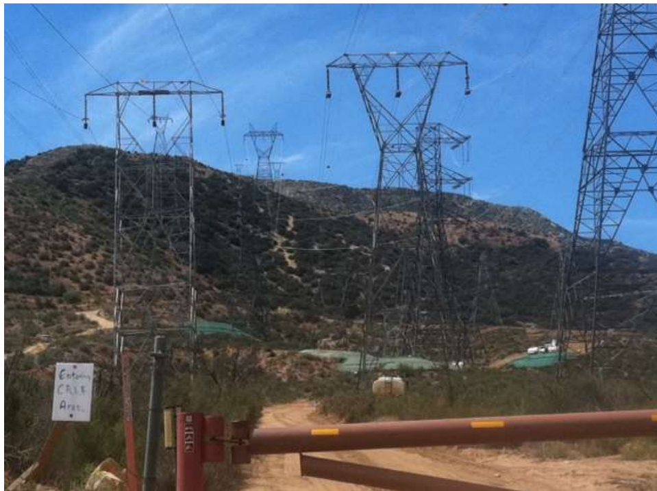
Figure 2: Hydromulching (BMP) application for final stabilization at Constructs 15, 16 and 17, Segment 11C.
