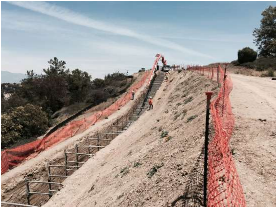
Figure 4: Backfilling mainline trench between VC #7 and VC #8.
