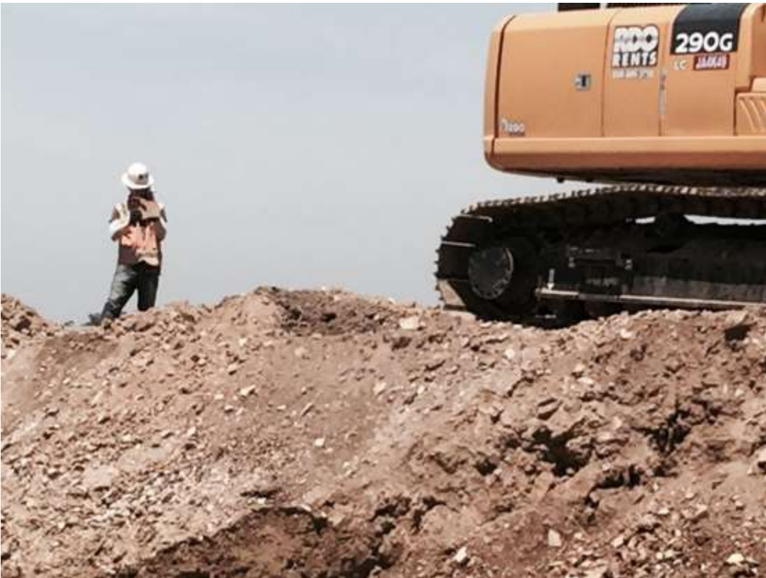
Figure 6: Paleontological Monitor onsite during major excavations at VC #3.
