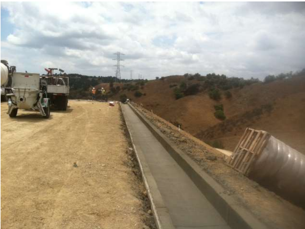
Figure 2: Concrete V-ditch installation at the WTS.
