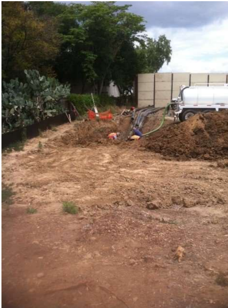
Figure 5: Crews working on conduit retrieval process at VC #12, 500 kV Underground.
