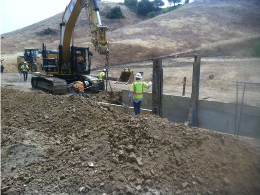
Figure 1: VC #4 excavation activities, 500 kV Underground.
