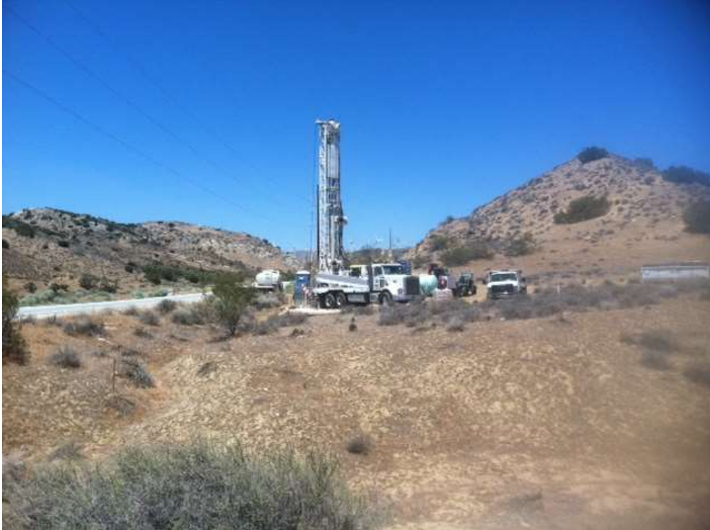
Figure 1: Ground Rod #16 excavation for cathodic protection activities, Segment 3B.
