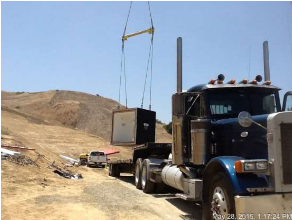
Figure 4: Vault installation activities at VC #4, 500 kV Underground.
