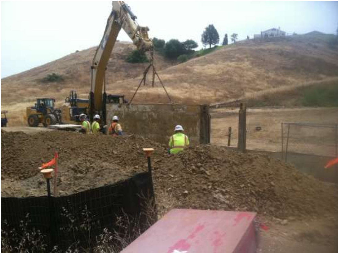
Figure 3: Excavation activities at VC#4, 500 kV Underground.
