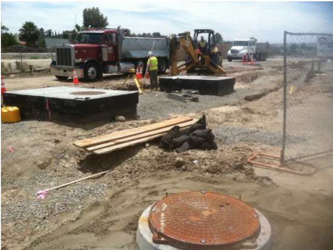
Figure 5: In/Out trench activities at VC #14, 500 kV Underground.
