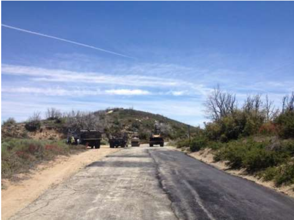
Figure 2: Paving activities along Mt. Gleason Road, Segment 11C.
