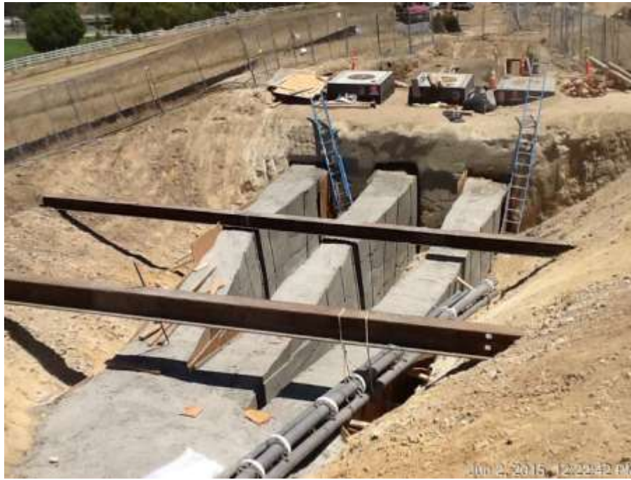
Figure 5: In/Out trench activities at VC #8, 500 kV Underground.
