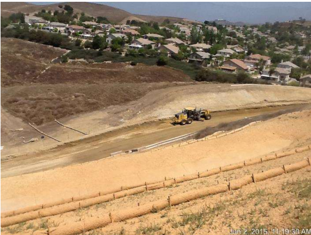
Figure 4: Backfilling and grading trenchline between WTS and VC #1, 500 kV Underground.
