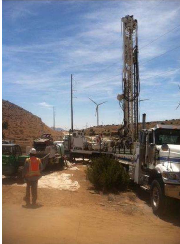
Figure 1: GR #16 excavation for cathodic protection activities, Segment 3B.
