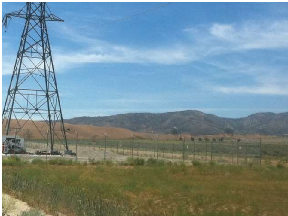
Figure 2: Gravel excavation activities to prepare area for Highwind Substation wall.
