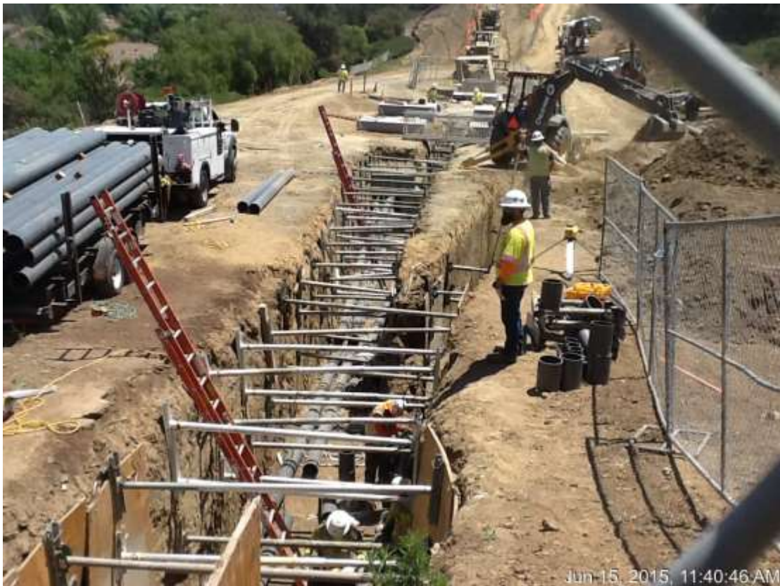
Figure 4: Conduit installation at VC #7, 500 kV Underground.
