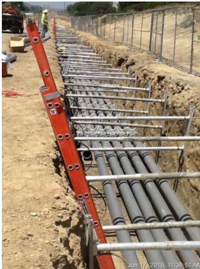
Figure 5: Conduit installation at VC #11, 500 kV Underground.
