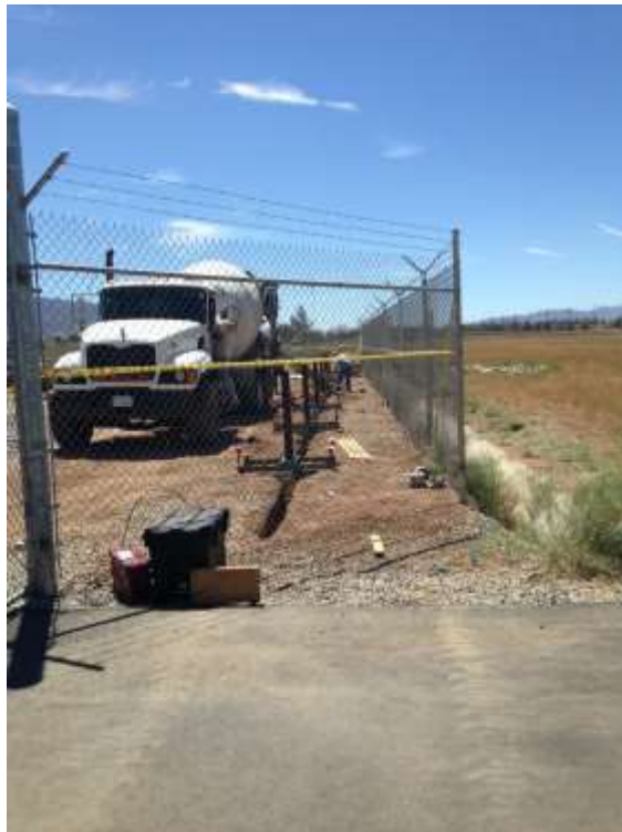
Figure 2: Placement of wall posts at Highwind Substation wall.
