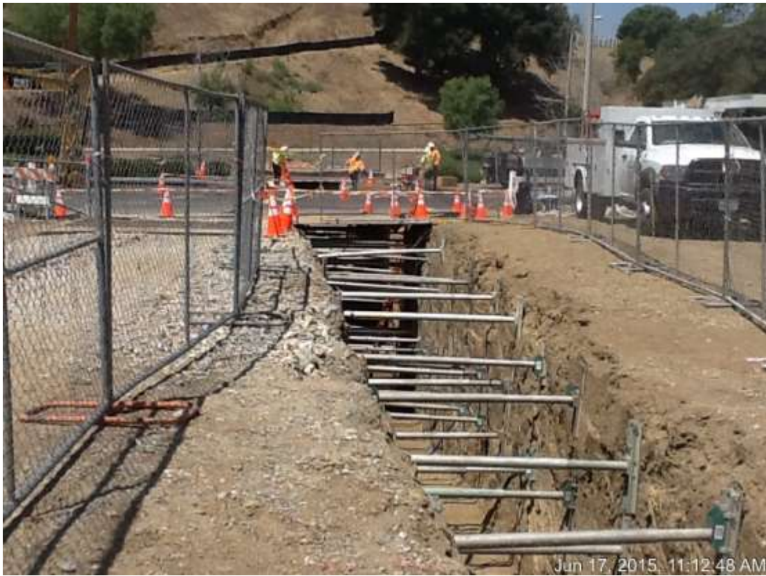
Figure 3: Trenching activities across Chino Hills Parkway, 500 kV Underground.
