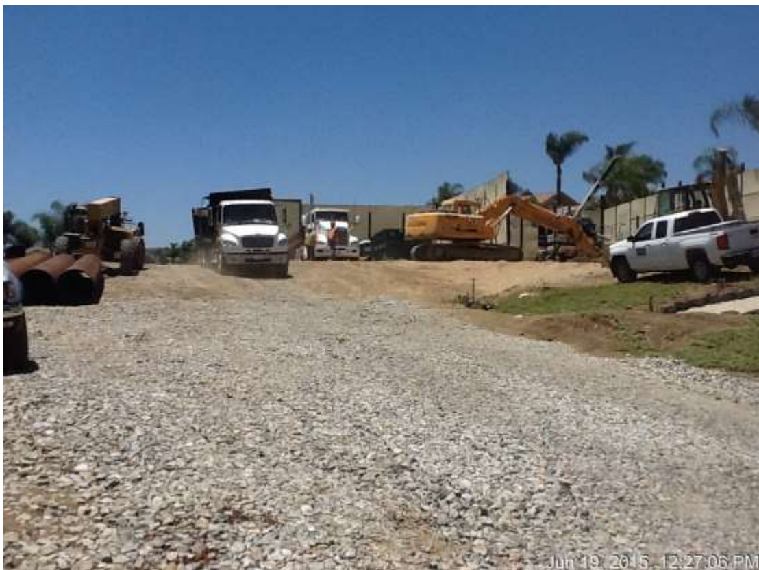
Figure 8: HDD activities at VC#11, 500 kV Underground.
