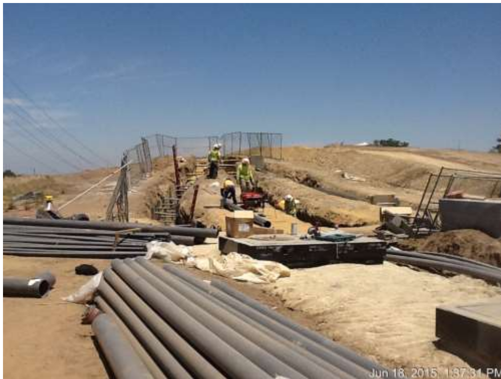
Figure 6: Conduit installation at VC #8, 500 kV underground.
