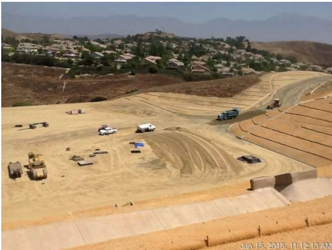
Figure 7: Class II Base application at the WTS access road, 500 kV Underground.
