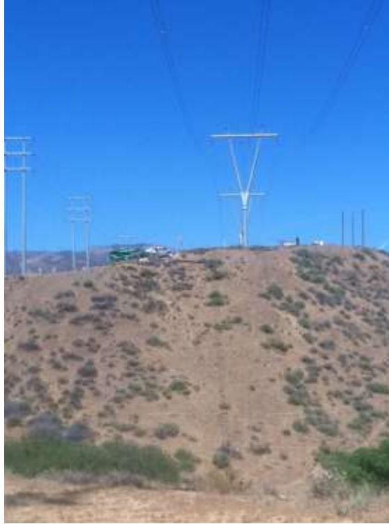
Figure 1: GR #13 relocation activities for cathodic protection activities, Segment 3B.
