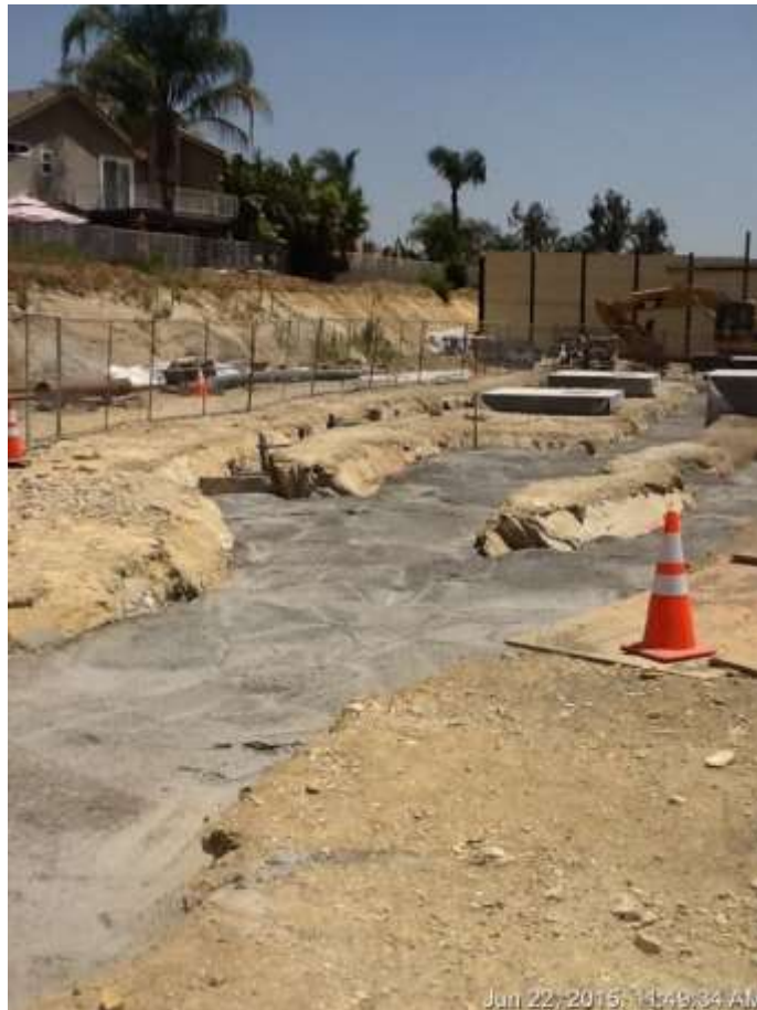
Figure 4: Concrete pour of trench lines at VC #11, 500 kV Underground.
