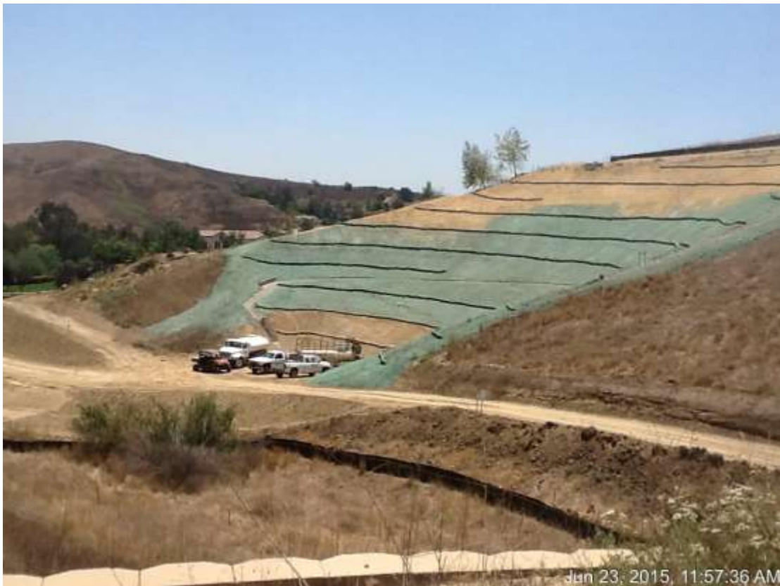
Figure 6: Hydromulching (BMP) installation at RV #1, 500 kV underground.
