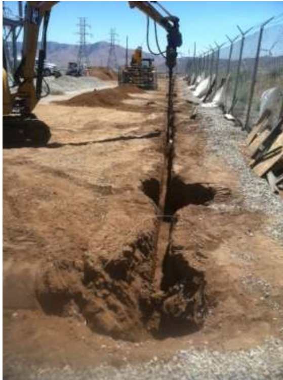
Figure 2: Placement of wall posts and trench at Highwind Substation wall.
