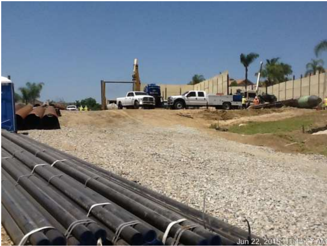
Figure 5: HDD operations at VC #11, 500 kV Underground.
