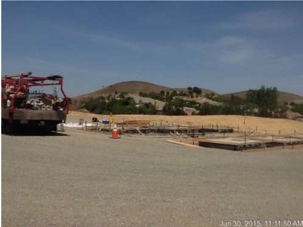
Figure 1: Form installation for concrete cap for VC#1, 500 kV Underground.
