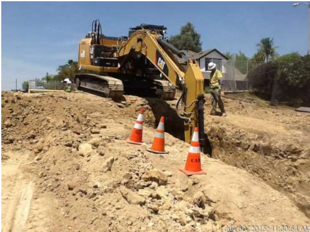
Figure 2: Trenching activities at the Morningfield Road crossing, 500 kV Underground.
