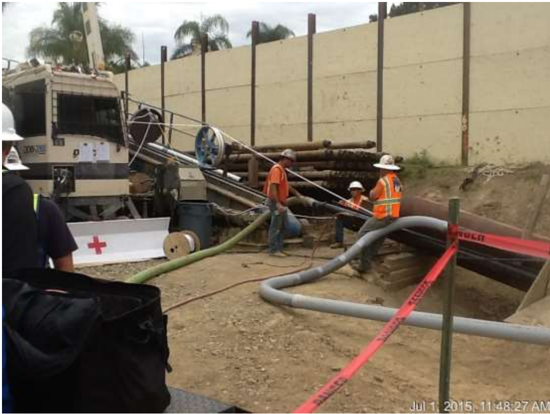
Figure 5: Crew members onsite during manned entry activities, 500 kV Underground.
