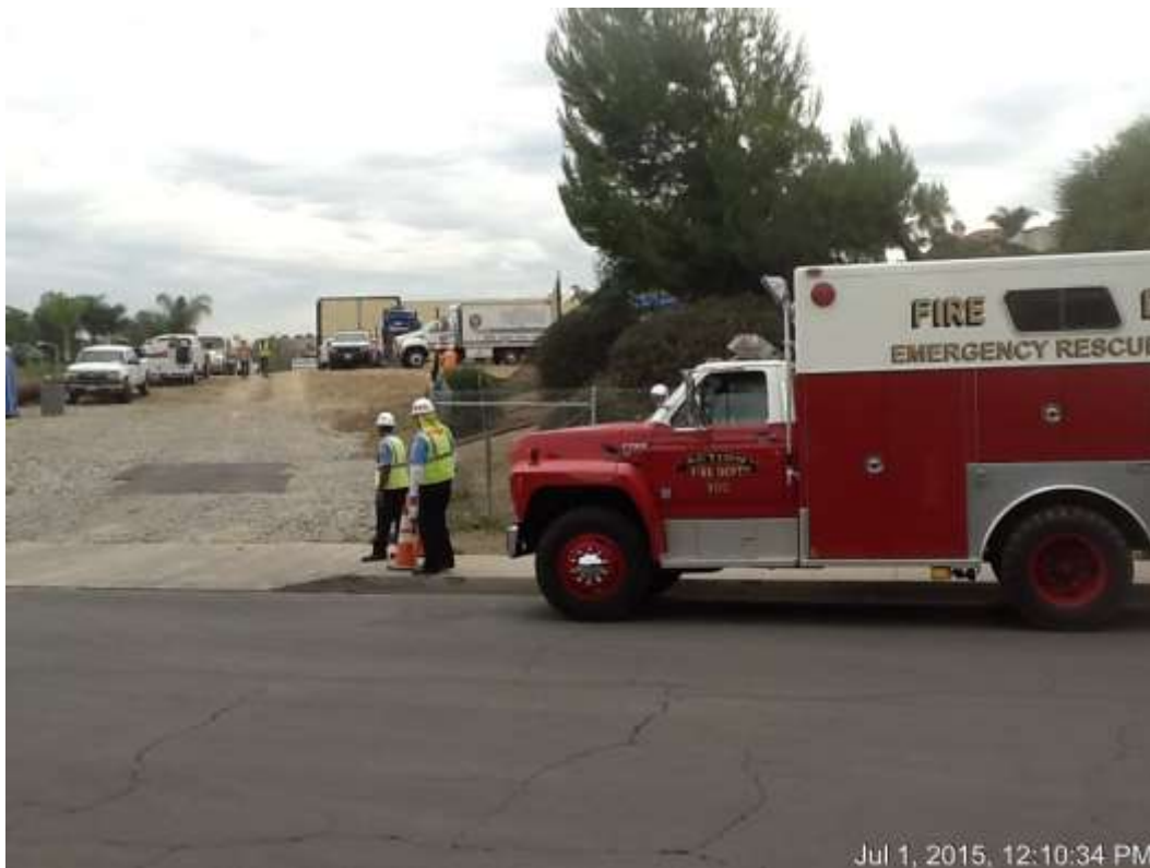
Figure 4: Private emergency response team onsite during manned entry activities, 500 kV Underground.
