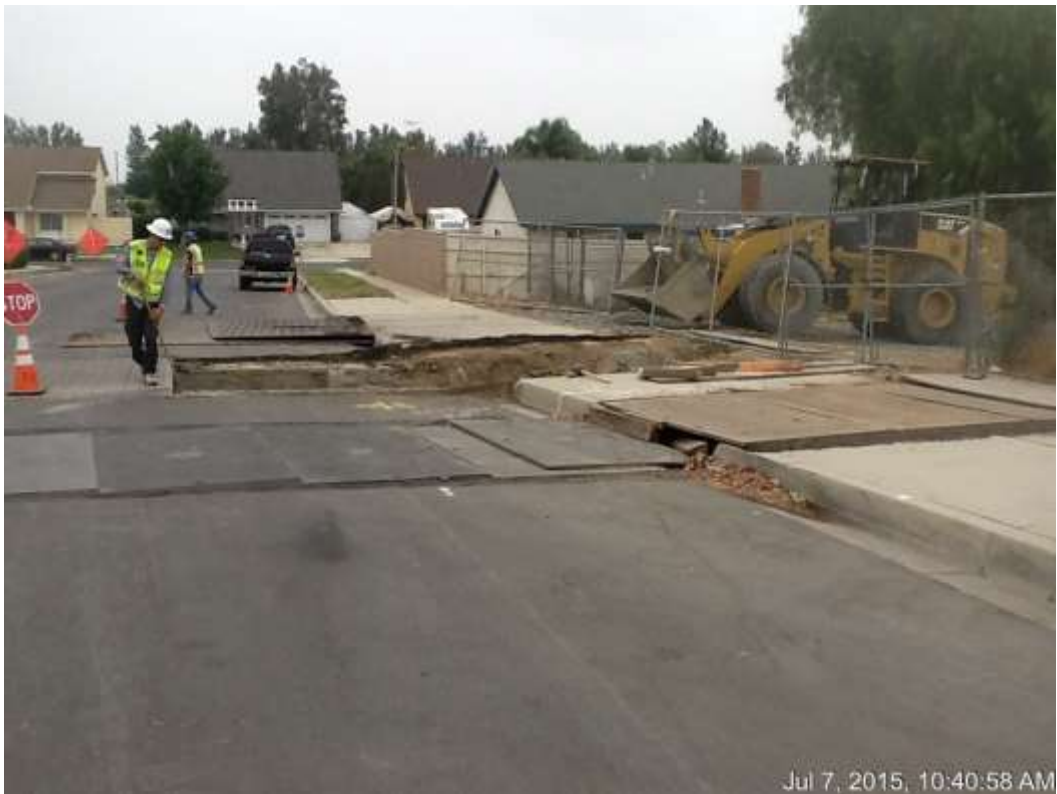
Figure 5: Trenching activities across Cork Drive, 500 kV Underground.
