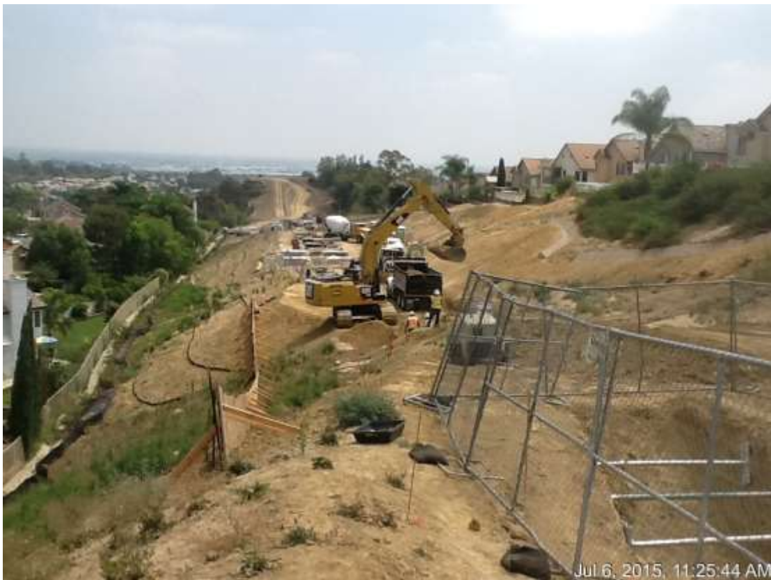
Figure 7: Trenching activities near VC #6, 500 kV Underground.
