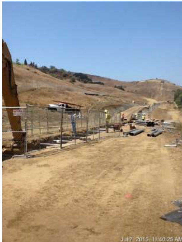
Figure 6: Trenching activities between RV #4 to VC #5, 500 kV Underground.
