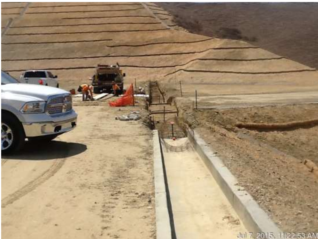
Figure 8: Swale installation at the WTS, 500 kV Underground.
