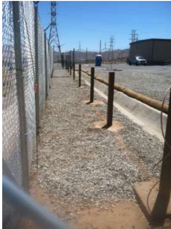
Figure 2: Wall pylons installed at Highwind Substation.
