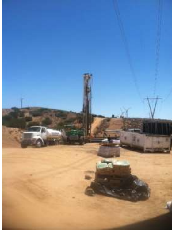
Figure 1: Ground Rod #14 in process on Segment 3B.
