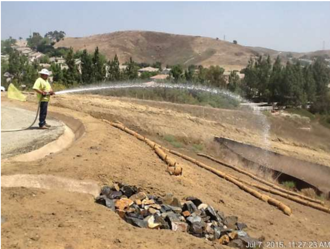
Figure 9: Watering of hydroseed at the WTS, 500 kV Underground.
