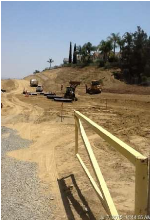
Figure 4: Grading activities at VC #7, 500 kV Underground.
