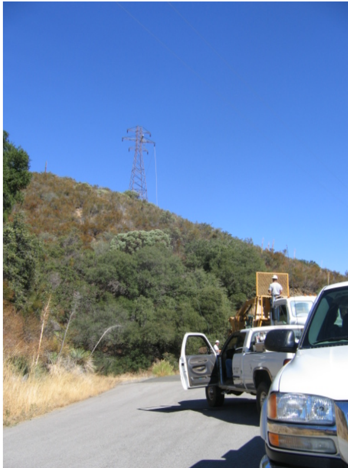
Figure 3: Crews completed the conductor removal in the ANF on October 6 th .
