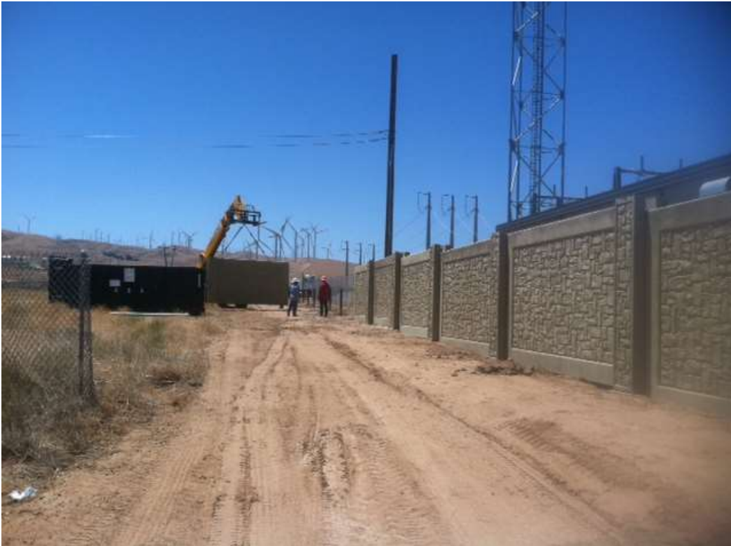
Figure 2: Wall panel installation at Highwind Substation.
