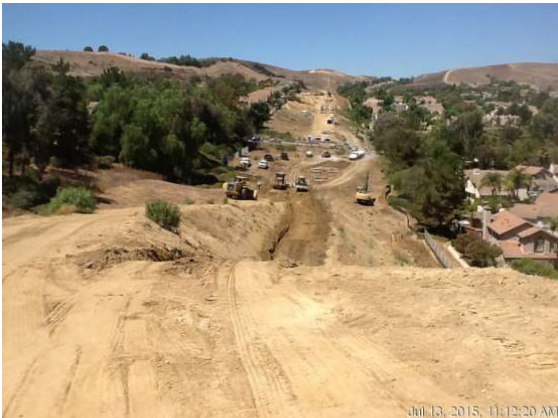
Figure 4: Grading activities between VC #7 and VC #8, 500 kV Underground.
