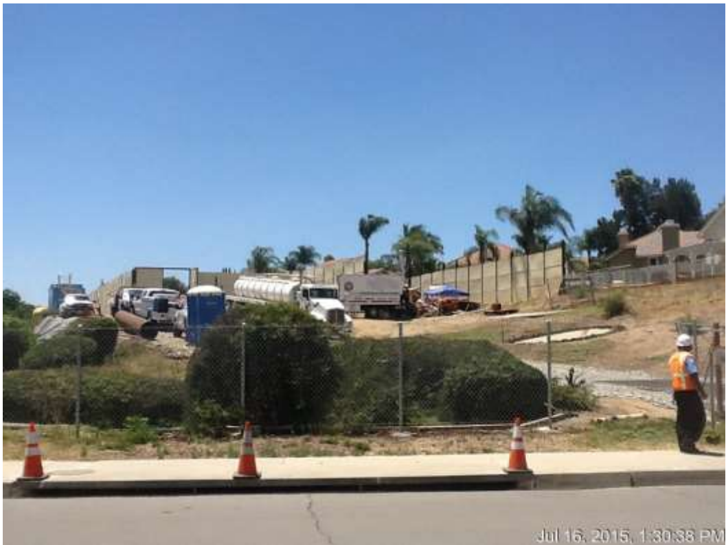
Figure 7: HDD manned entry activities continue at VC#11, 500 kV Underground.
