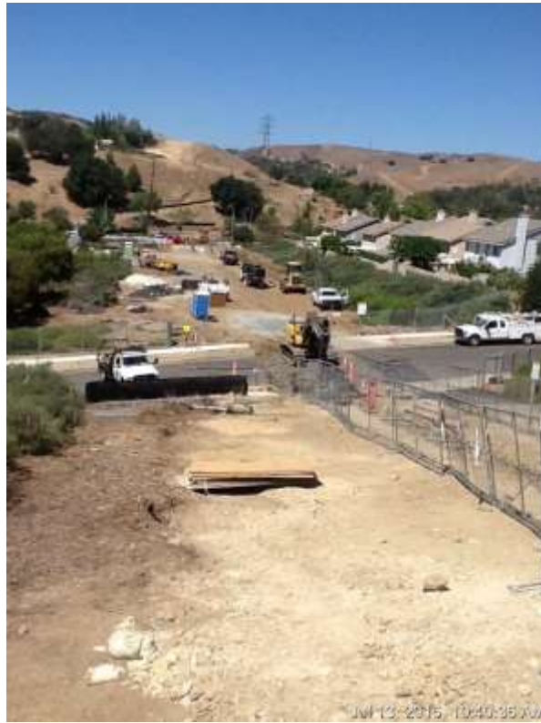
Figure 5: Trenching across Little Bend, 500 kV Underground.
