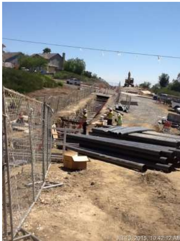
Figure 6: Trenching activities between VC #9 and #10, 500 kV Underground.
