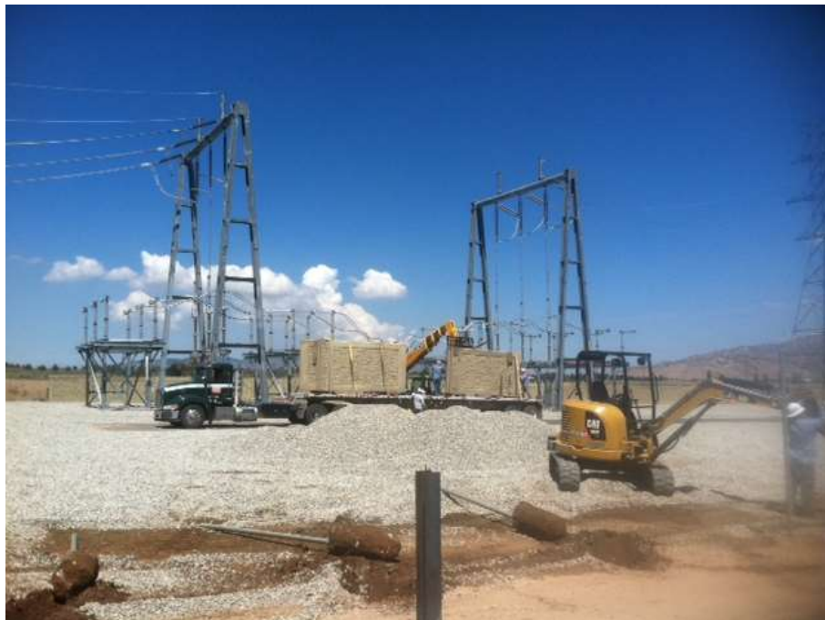
Figure 2: Wall panel delivery and installation at Highwind Substation.
