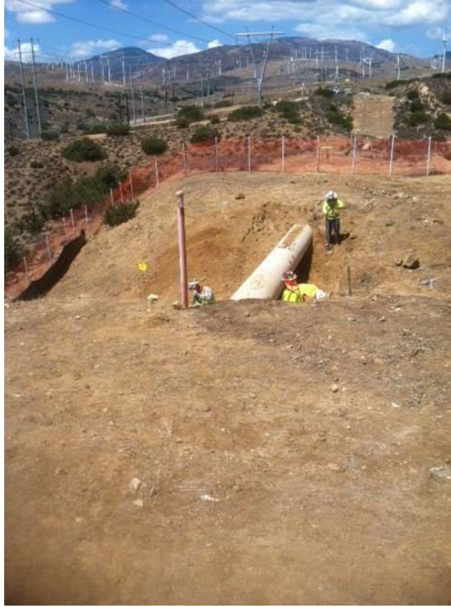
Figure 1: Gas pipeline span burial activities on Segment 3B.
