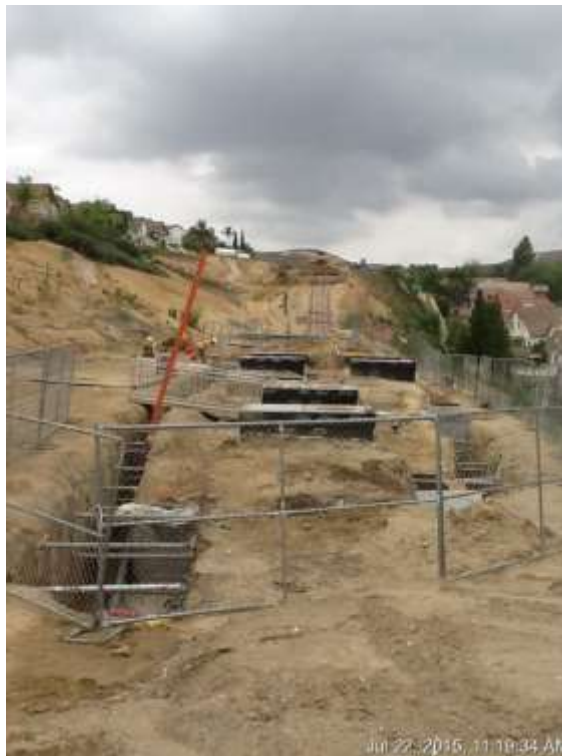
Figure 4: Conduit installation between VC #6, 500 kV Underground.
