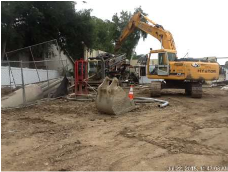
Figure 5: Conduit retrieval activities at VC #12, 500 kV Underground.
